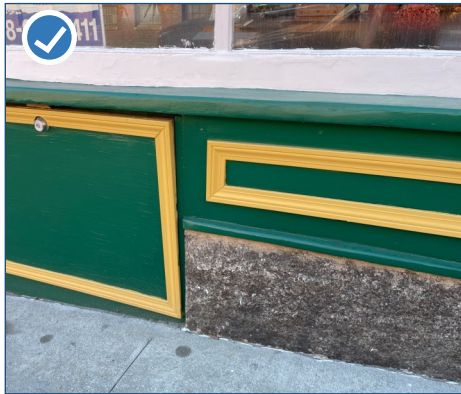
Figure 129: Appropriately obscured access to mechanical equipment within a storefront bulkhead.
