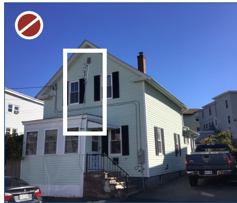
Figure 132: Inappropriate location of unpainted and unconcealed antenna.
