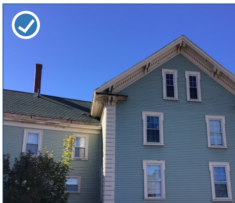
Figure 124: Appropriately preserved roof shape and roofing material.
