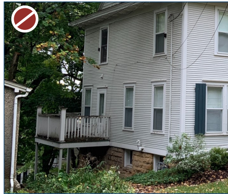
Figure 121: Inappropriate side deck addition.
