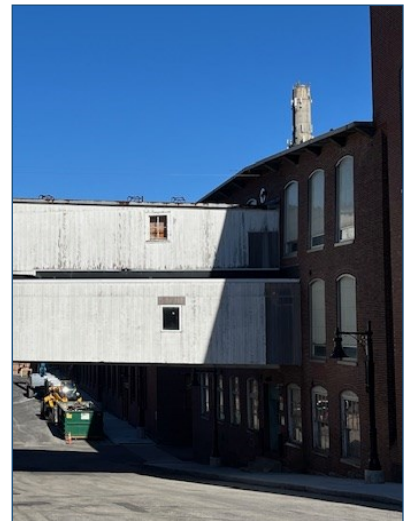
Figure 20: Wooden enclosed bridges can be found throughout the Biddeford / Saco Mills Historic District. The bridges connect the former mill buildings.
