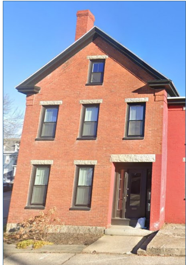
Figure 40: Residence with Greek Revival elements such as general symmetry, pronounced lintels over windows and doors, and a decorative cornice with a gable return.
