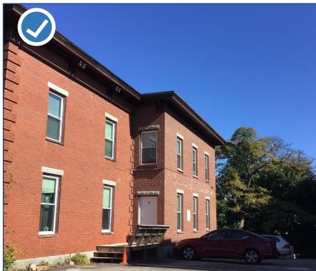
Figure 138: Appropriate rear addition built with compatible materials, roof form, and features.
