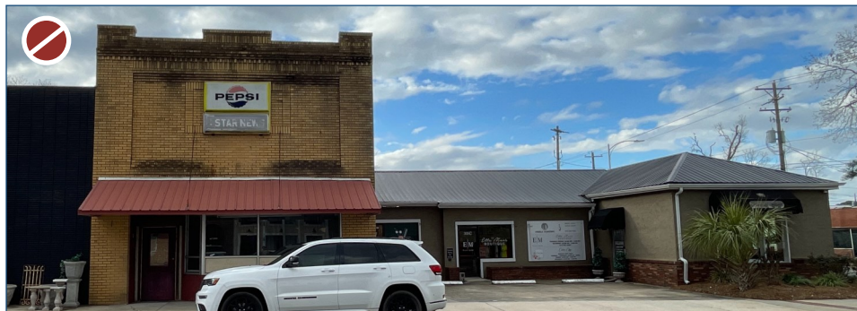
Figure 136: Inappropriate new construction within a commercial area with an incompatible setback, alignment, massing, height, scale, and rhythm.
