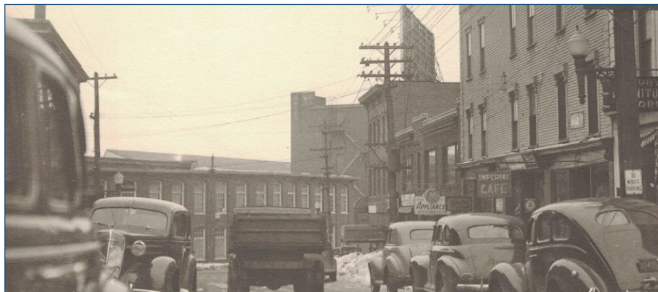
Figure 11: Alfred Street, Biddeford, near Bacon Street looking toward Main Street. February 17, 1945. Source: Biddeford Historical Society.
