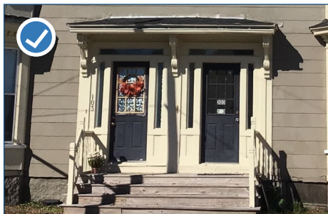
Figure 118: Preserved bracketed front porch.
