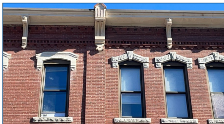
Figure 98: Architectural features on the front façade of a historic commercial building.
