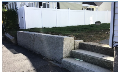
Figure 67: Historic fences and retaining walls should be maintained or replaced in-kind as needed.
