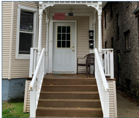
Figure 60: Porch flooring and steps replaced with compatible substitute material similar in visual qualities.
