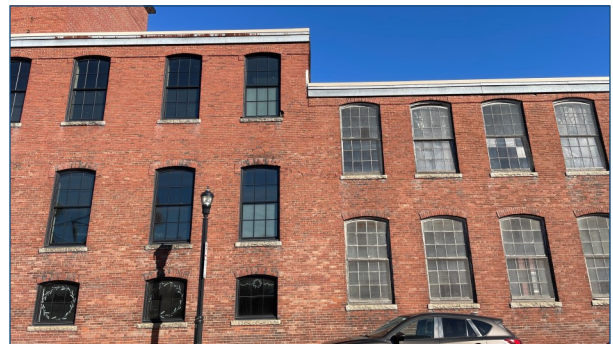
Figure 36: Many industrial mill buildings were constructed with a vernacular style.
