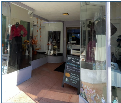
Figure 83: Menu board signage at the front of a storefront, appropriately located out of the public right-of-way.
