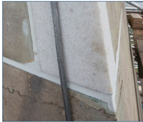
Figure 61: Appropriate dutchman replacement on masonry.
