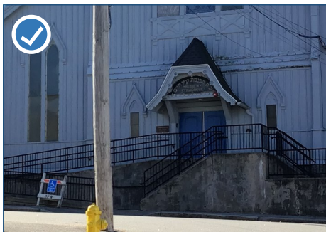
Figure 87: Appropriate ramp on the front façade of a public building.
