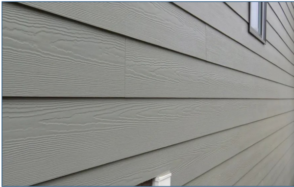
Figure 161: Synthetic Vinyl siding. Source: Urban Exteriors.
