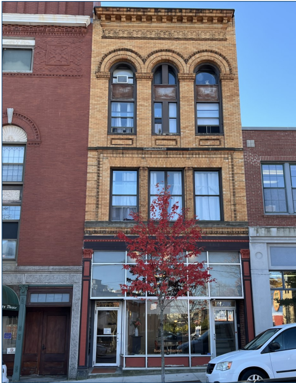
Figure 15: Italianate commercial building located at 215 Main Street.
