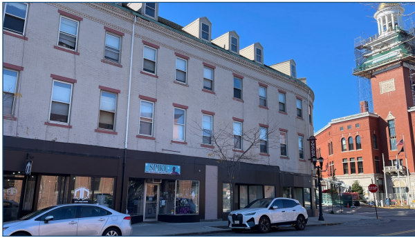
Figure 38: Large commercial building constructed in a Greek Revival style.
