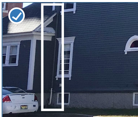
Figure 126: Appropriately located and painted downspout on the side of a residence.
