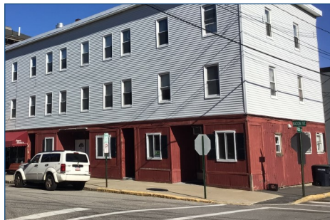
Figure 68: Sidewalk and curb found in the commercial area.
