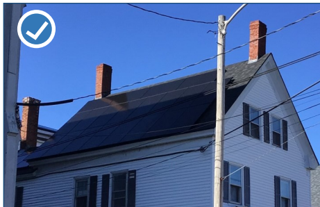
Figure 133: Appropriately located solar panels on side elevation of a historic residence.
