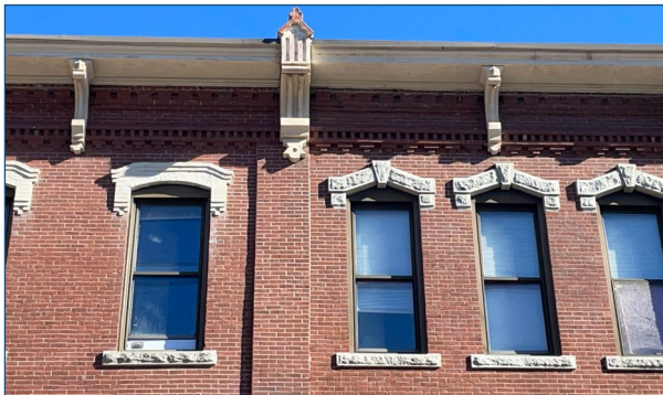
Figure 44: Italianate features found on a commercial building within the Biddeford Main Street Historic District.
