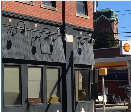
Figure 115: Typical gooseneck lighting within the commercial area of Biddeford.
