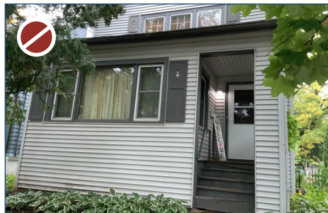
Figure 119: Inappropriately enclosed front porch.
