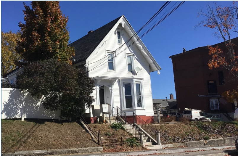
Figure 41: Vernacular example of a Gothic Revival style residence.
