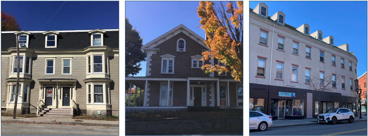
Figure 55: These examples of properties with moderate historic integrity have all retained their form, but some materials and stylistic details have been lost or changed.
