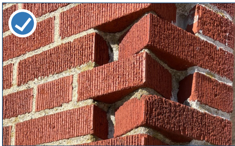
Figure 93: Appropriate brick and mortar pairing within Biddeford.
