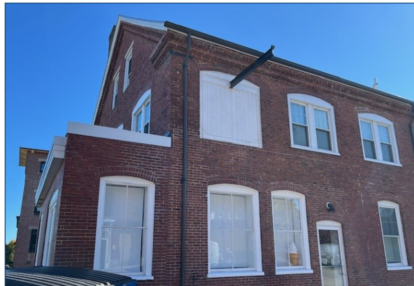
Figure 39: An office building in the Biddeford / Saco Mill Historic District that features some Greek Revival elements.
