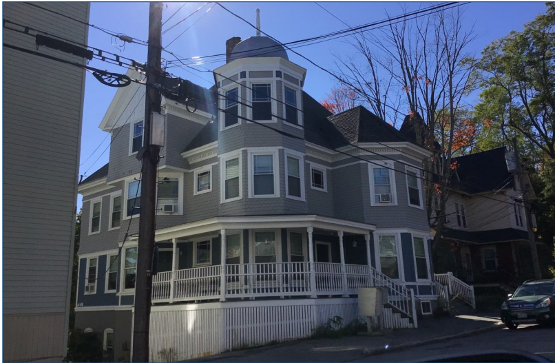
Figure 49: Queen Anne style residences are typically constructed larger in size and so many have later been converted to multi-family homes.
