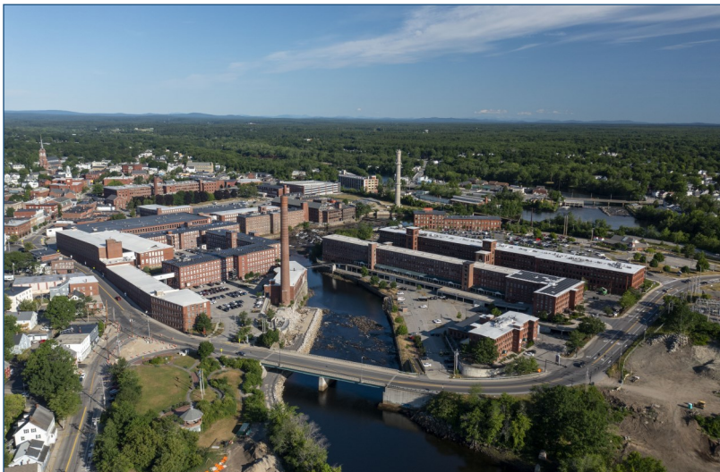
Figure 19: Aerial view of the Biddeford / Saco Mills Historic District, which is located along the Saco River.
