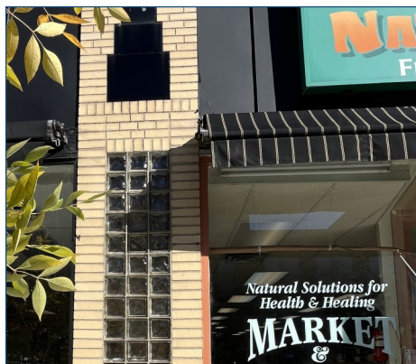
Figure 113: Sloped, retractable awnings within Biddeford's commercial area.
