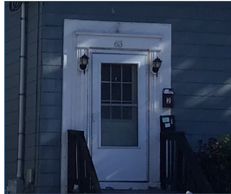
Figure 116: Many residences have paired lights around the front door.
