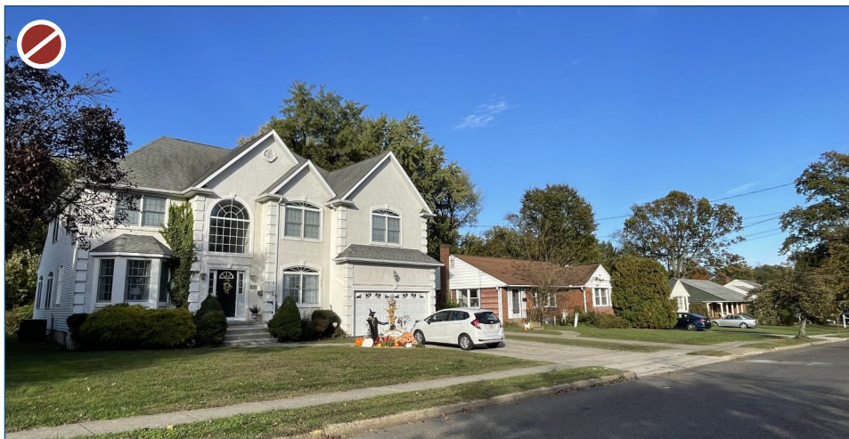
Figure 142: New residential construction with inappropriate materials along with scale and massing.
