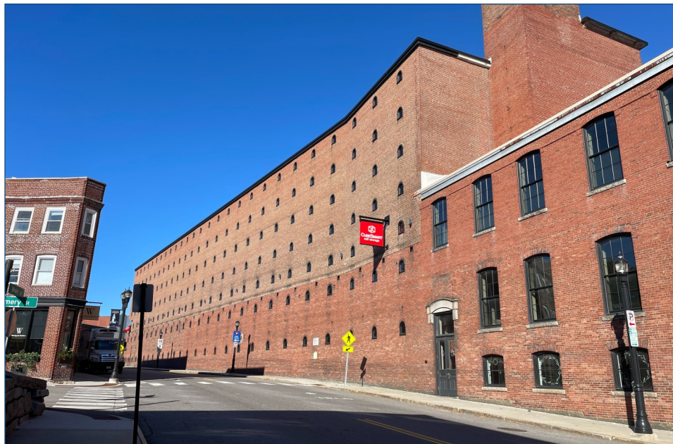
Figure 72: Street furniture located along the Biddeford / Saco Mills Historic District.
