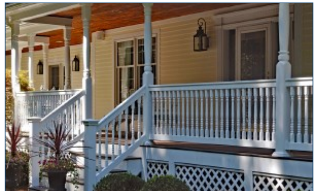
Figure 154: Pressure treated lumber porch railing. Source: Perfection Fence.
