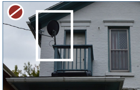
Figure 134: Inappropriate location of a satellite dish on the front façade of a historic residence.
