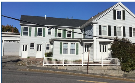
Figure 66: Example of fencing and a retaining wall along the front of a residence.
