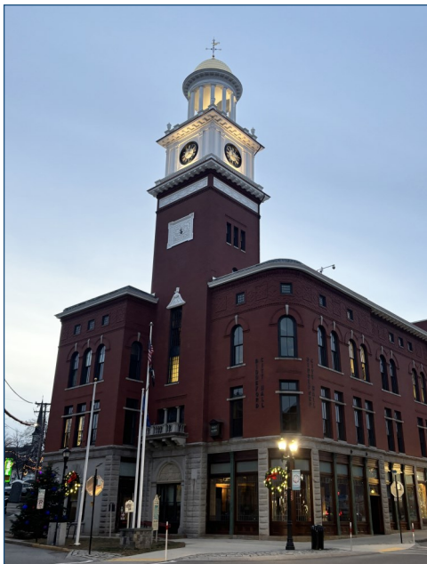
Figure 21: Biddeford's City Hall located at 205 Main Street.
