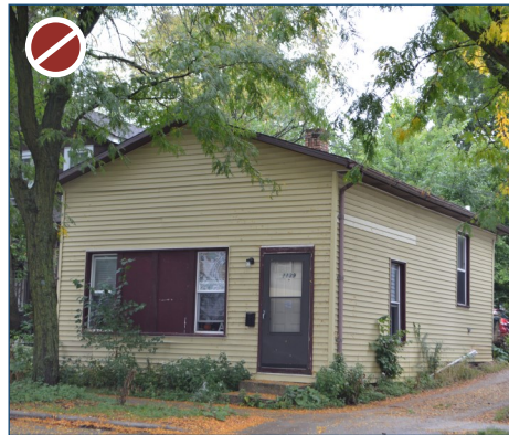
Figure 97: Inappropriate siding replacement that has resulted in a loss of historic integrity for the residence.
