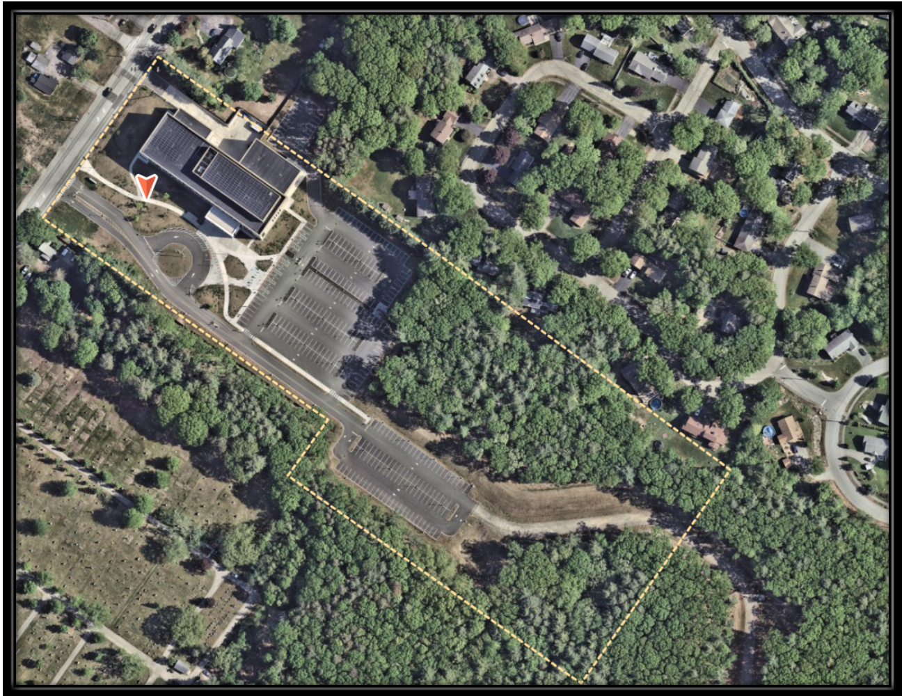
Existing Site Conditions May 7, 2024
