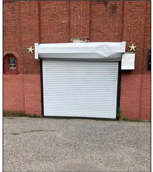
Existing Overhead Door, South Elevation
