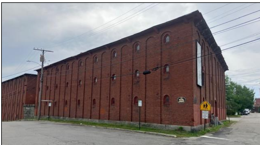
North elevation from Pearl Street looking South
