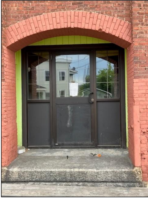
Existing Entry Doors, West elevation
