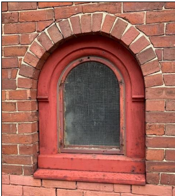
Existing Portal Windows Measures 24" x 32" Approx.
