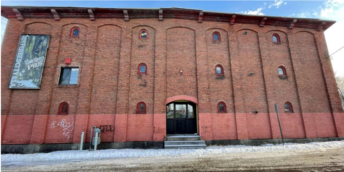
Figure 2 Buildings 12 Pearl Street— The existing structure is an empty former mill building that has remained vacant for numerous years.
