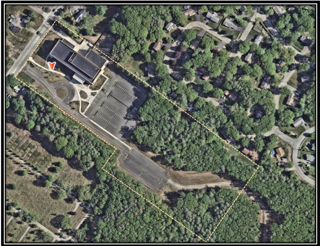
Existing Site Conditions May 7, 2024
