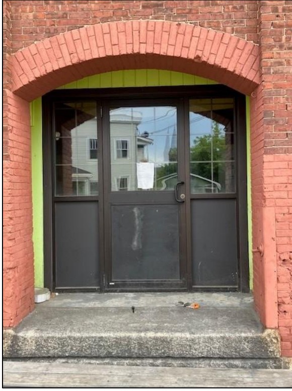
Existing Entry Doors, West elevation
