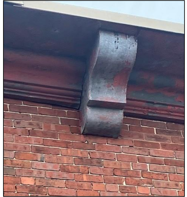
Existing Corbels (Typical)
