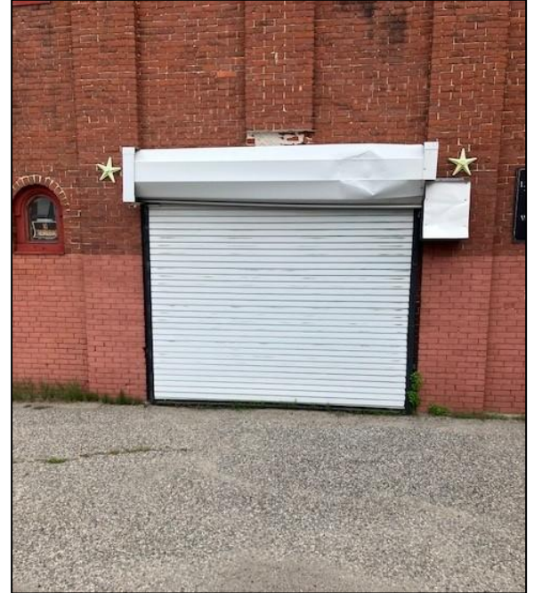
Existing Overhead Door, South Elevation
