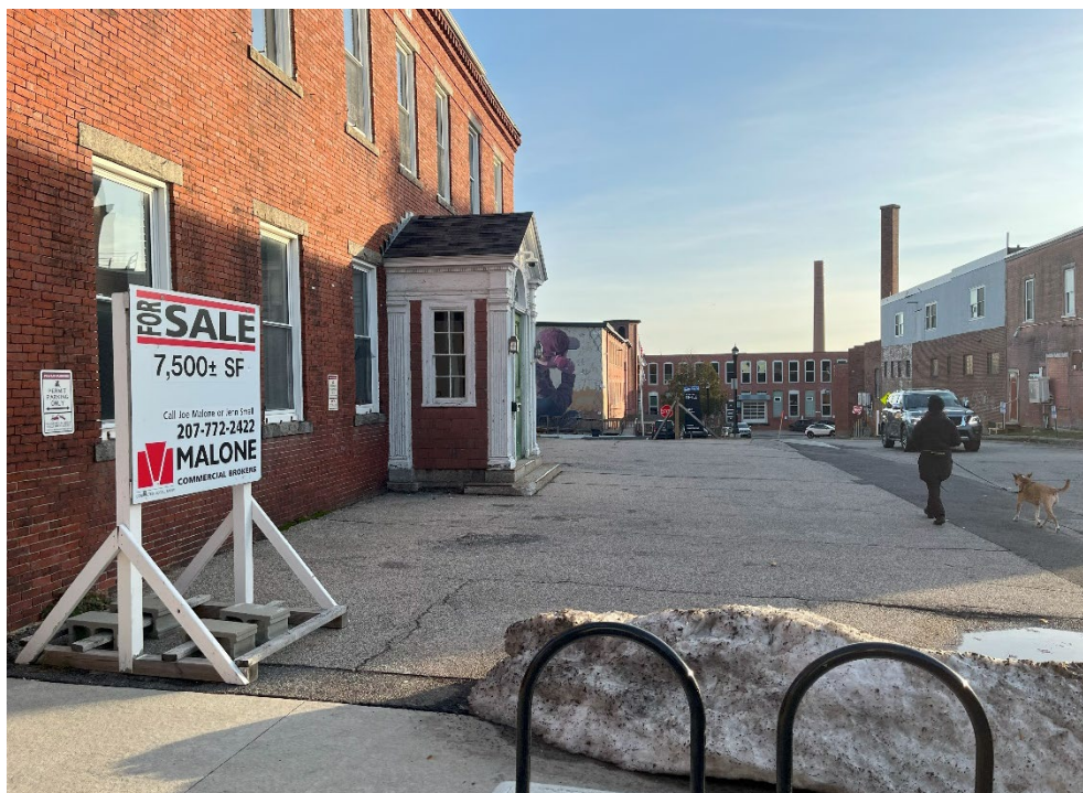
Figure 1: View of the south side of Building 30 facing east down York Street.
