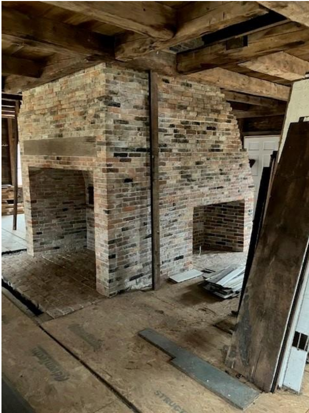
Figure 9 New central chimney John Tarr House November 13, 2025
