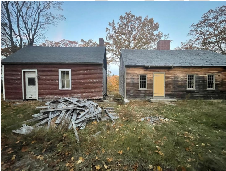
Figure 6 John Tarr House November 13, 2025, with ell no longer attached and altered door/window.
