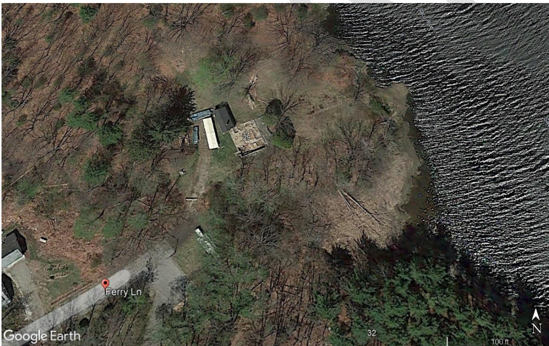
Figure 2 Location of the John Tarr House in a May 2018 aerial photograph with the ell present but the house moved.
