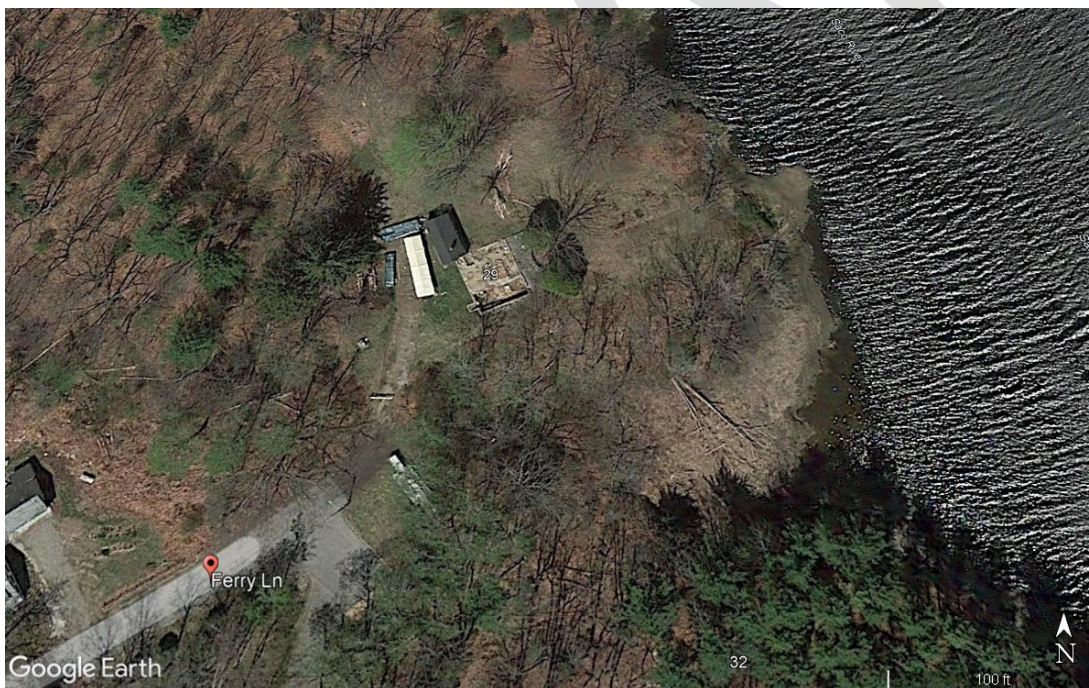
Figure 2 Location of the John Tarr House in a May 2018 aerial photograph with the ell present but the house moved.
