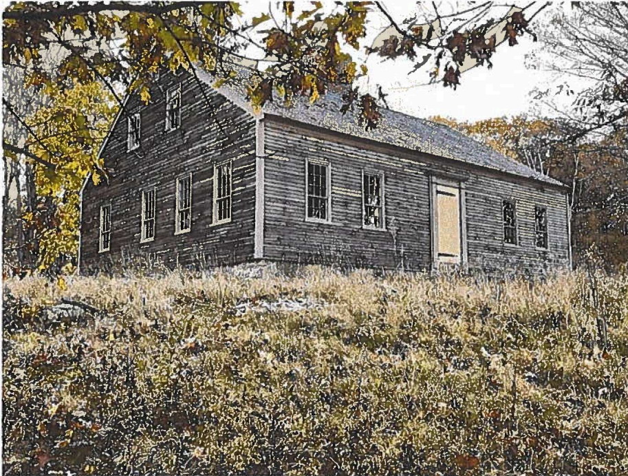
Figure 5 John Tarr House November 13, 2025 with door on the gable side replaced with a window.
