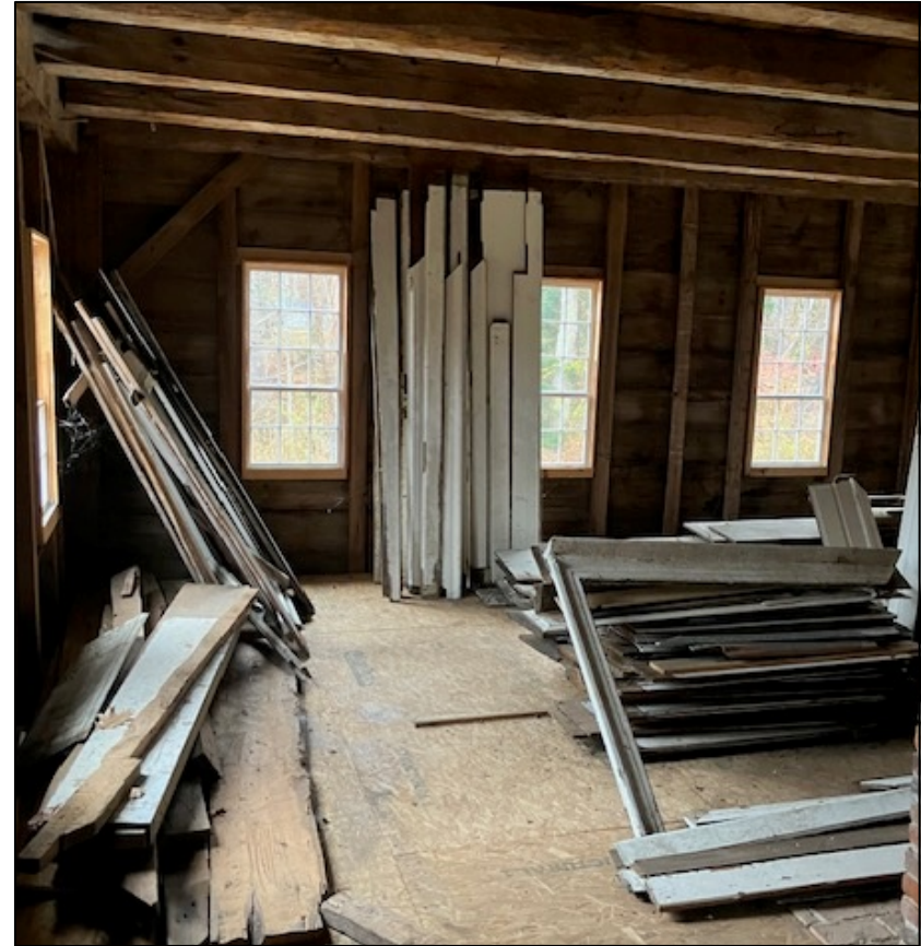
Wood Paneling Removed from Interior
