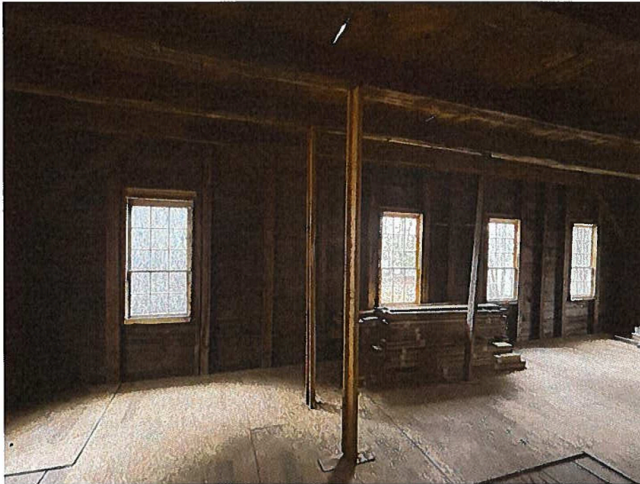
Figure 7 Interior of John Tarr House November 13, 2025, no interior finishes or partitions
