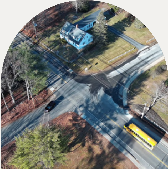
McManus Road – Existing Conditions ↓
