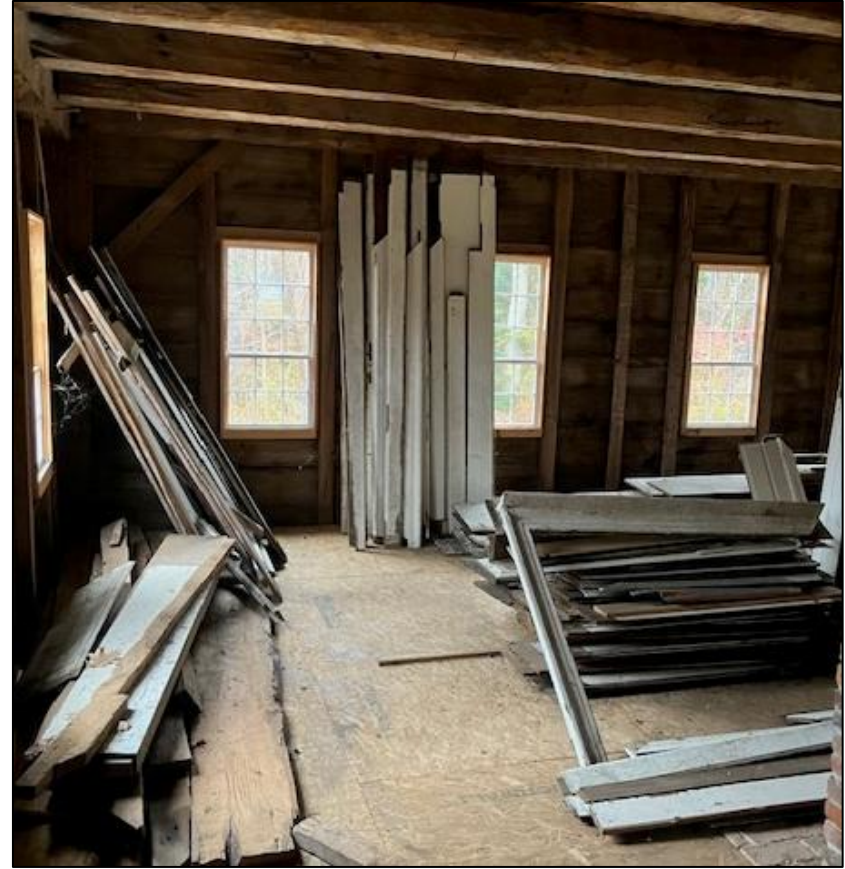
Wood Paneling Removed from Interior
