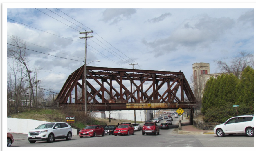
Figure 4. Elm Street Railroad Bridge
