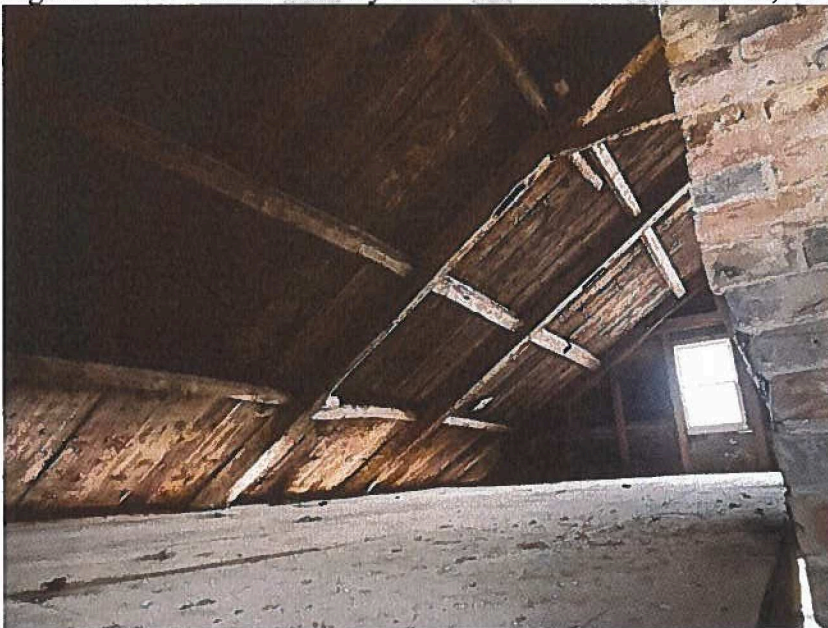
Figure 10 Attic of John Tarr House November 13, 2025
