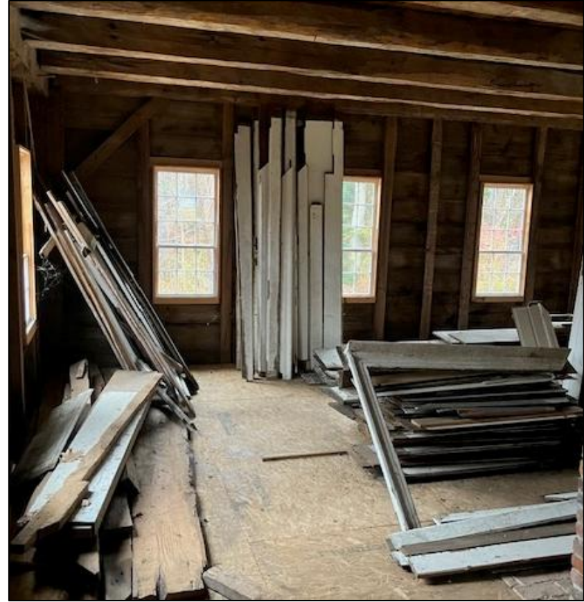
Wood Paneling Removed from Interior
