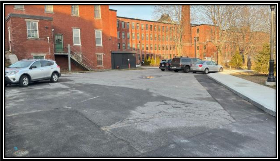
Pepperill Mill - Building # 30 – 2 York Street – Front Façade
