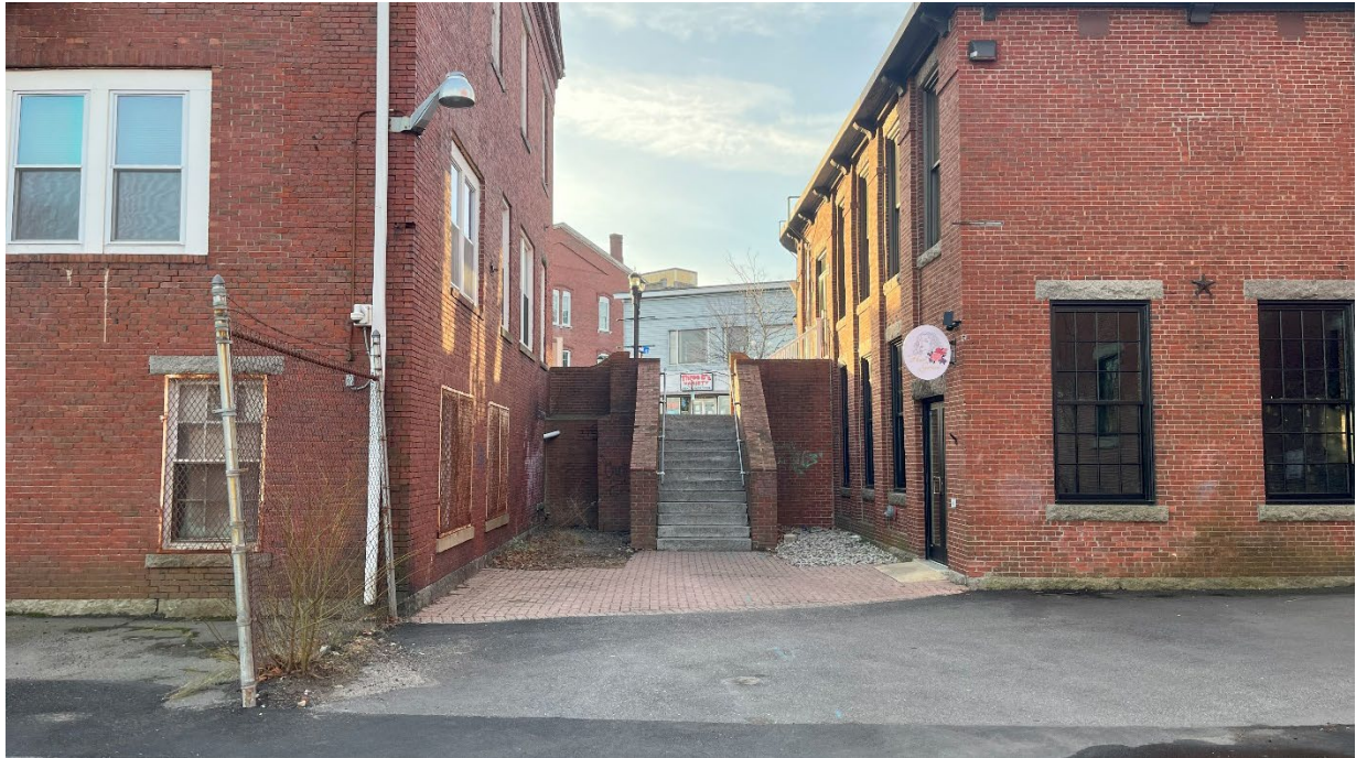
Figure 3: View of stairwell on west side of building 30. Facing south.
