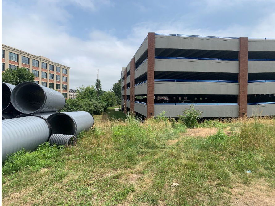
5. Standing in the middle of Lot 1. Facing east toward the existing parking garage.
