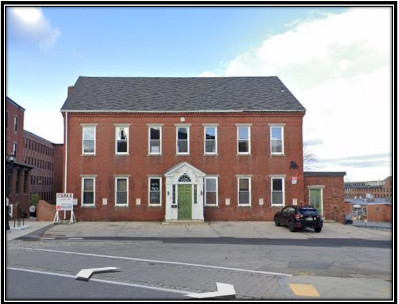
Pepperill Mill - Building # 30 – 2 York Street – Front Façade
