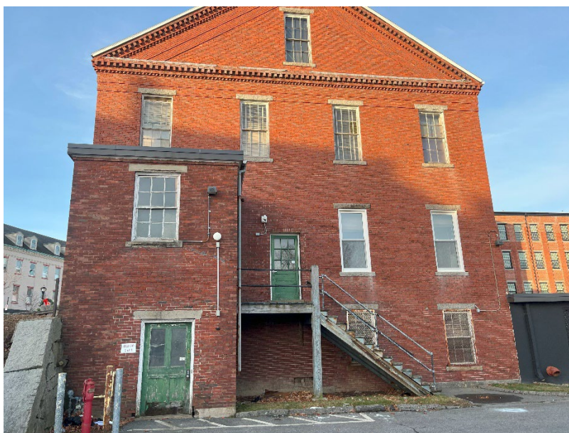
Figure 2: View of the east face of Building 30 facing west.
