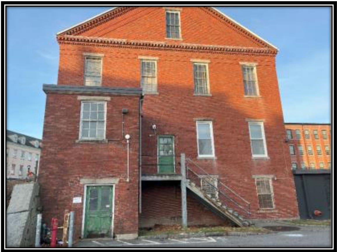
Pepperill Mill - Building # 30 – 2 York Street – Side / East Façade
