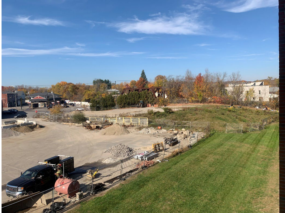
7. Looking down onto Lot 1B from adjacent municipal garage.
