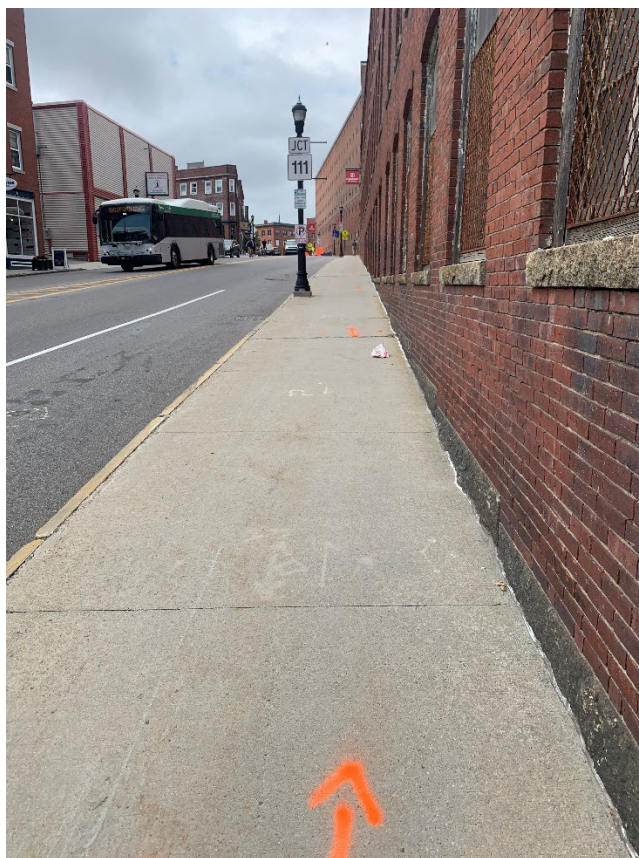
Figure 4: View of the south face of Building 19 & 20 facing west.
