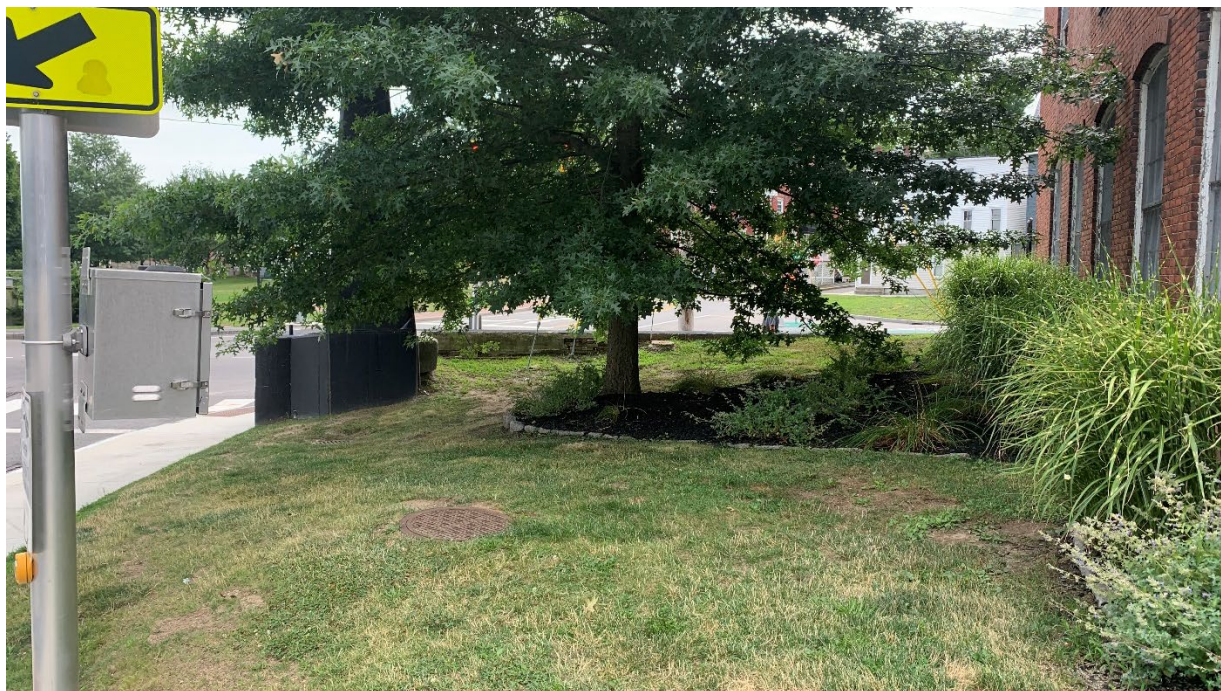
Figure 3: View of the east face of Building 20 facing south.
