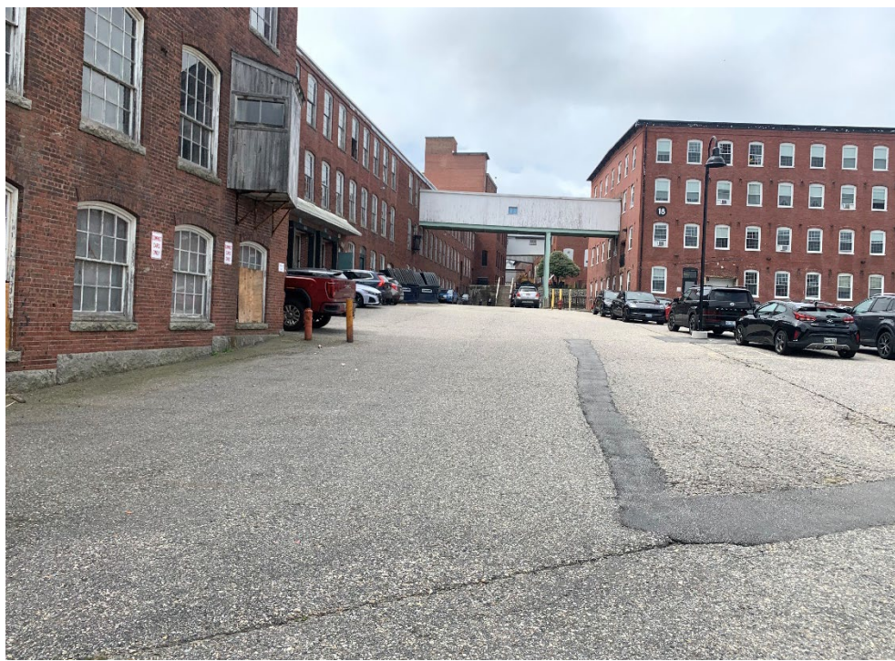
Figure 1: View of the north face of Building 19 & 20 (left side of image) facing west.
