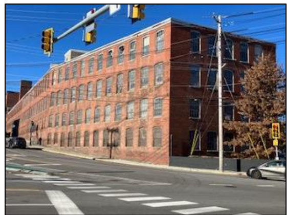
Building 20 anchors the entrance to North Dam Mill at Main Street.
