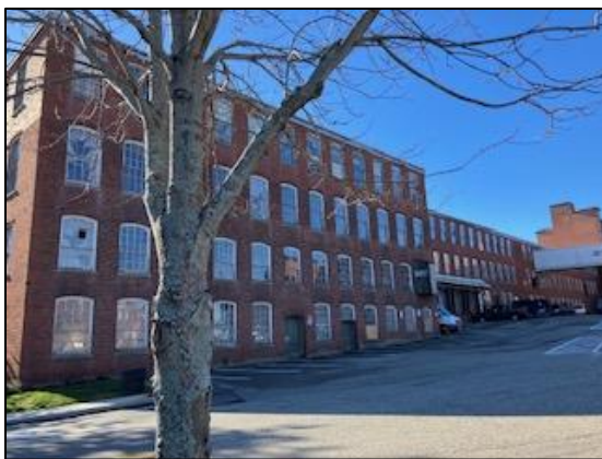
North side of Buildings 20 (left) and 19 (right).
