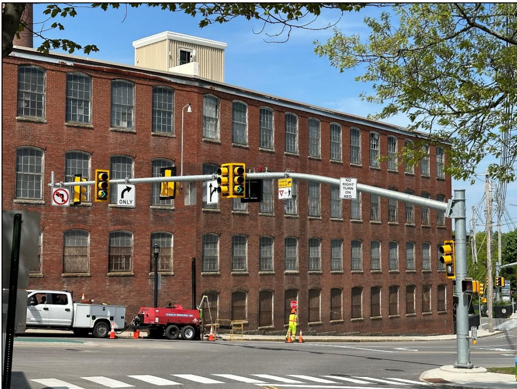
Building 20 as viewed from Hill Street
