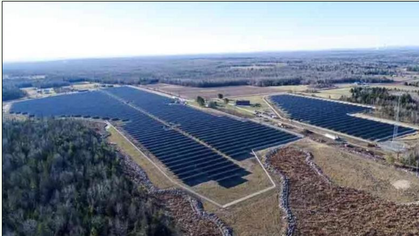
At left: 10 mega watt solar array in Pittsfield
