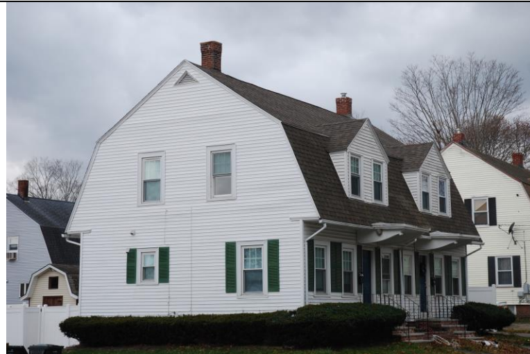
Photo 7: #2-4 Spare Street, looking southwest
