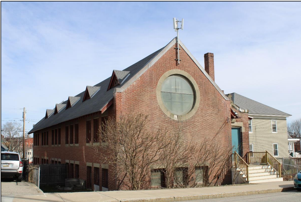
The building as it appeared in the 2022 Kleinfelder Survey
