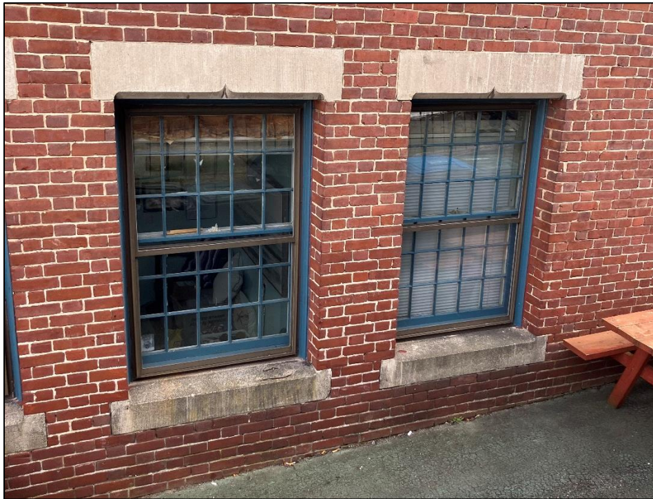
Existing Conditions: Windows "A" on South elevation
