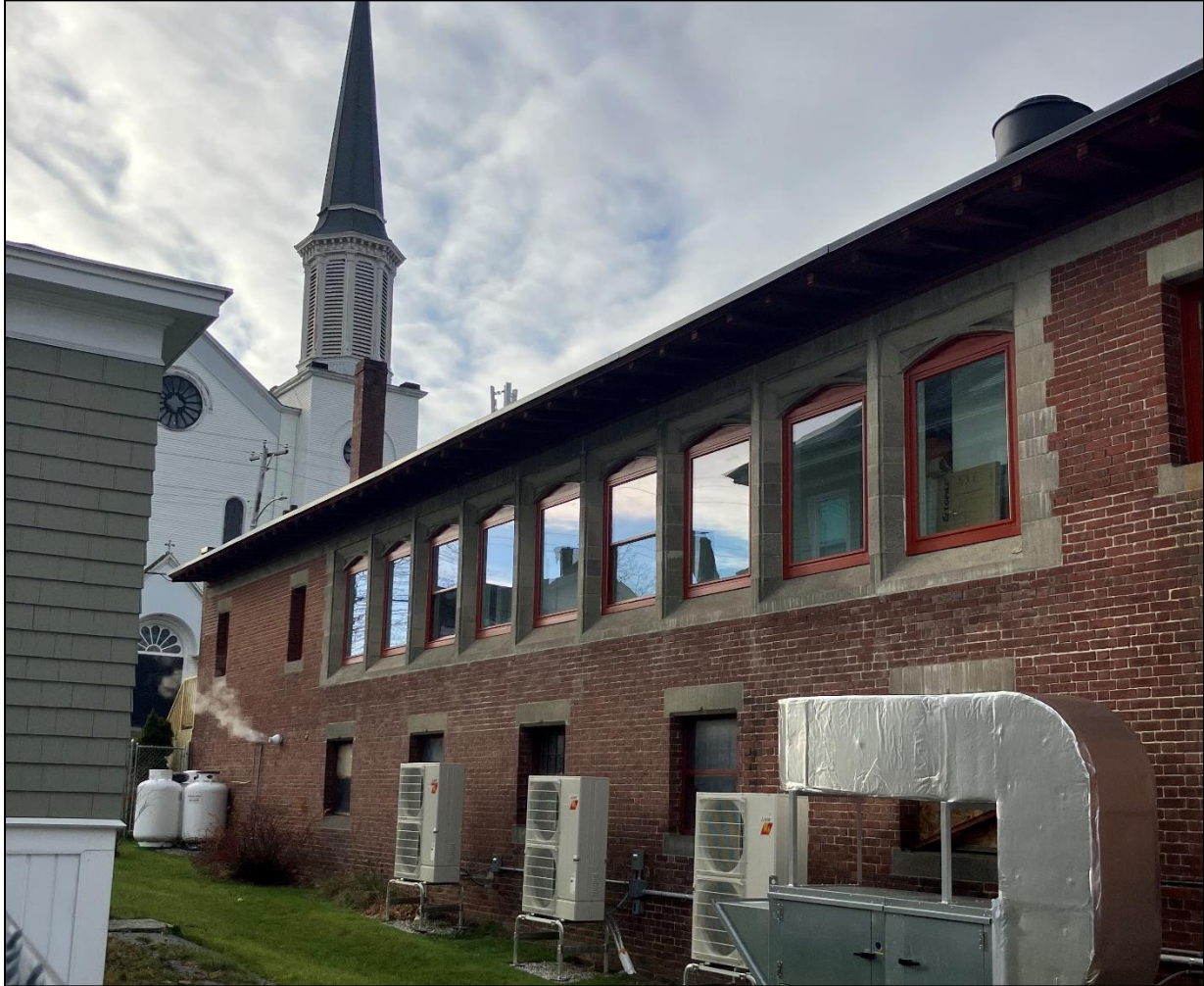
Existing Windows at South Elevation. These units were replaced during the summer of 2024.
