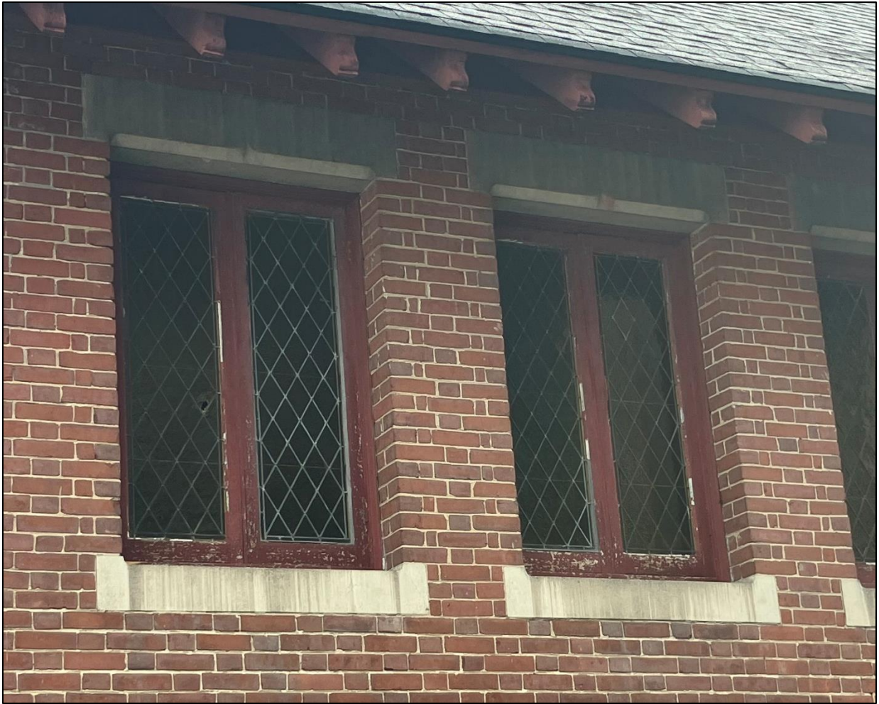
Existing Diamond Grille Pattern Windows to be Refinished.
