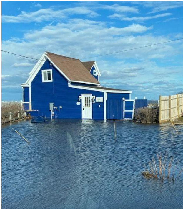
Flooding after the storm.
