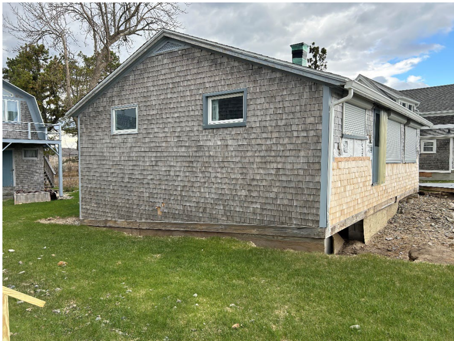
Building 2 view to Northeast
