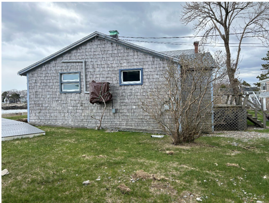
Building 2 view to Southwest
