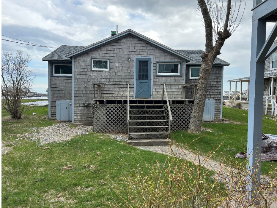
Building 2 view to Southeast
