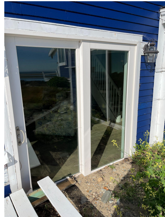
Existing grade above sliding door.
