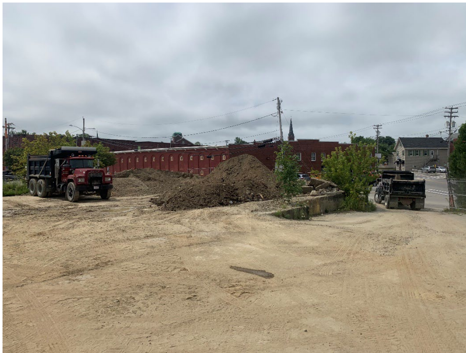
6. Standing in the middle of Lot 1. Facing west.
