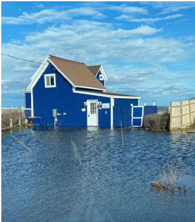
Flooding after the storm.
