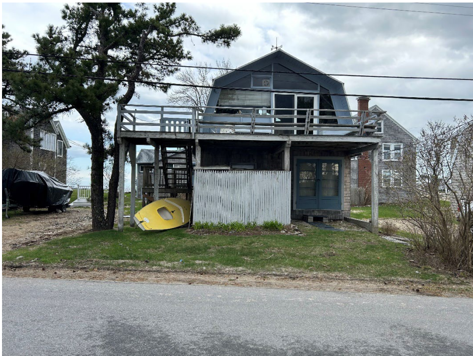
Building 1 view from Granite Point Road (to Southeast)
