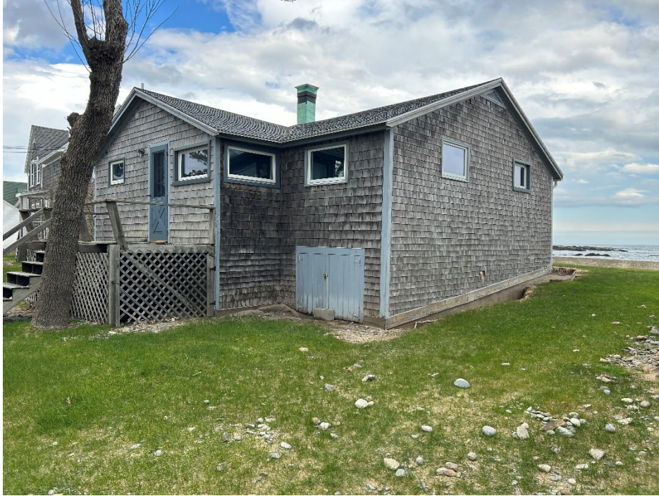
Building 2 view to East
