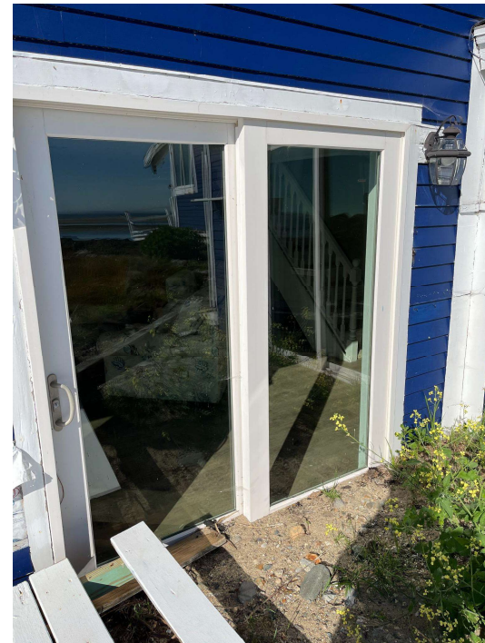
Existing grade above sliding door.
