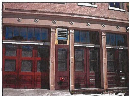
Left and Upper Right: The left bay was enlarged to create a vehicular opening which is compatible with the building's historic character.
