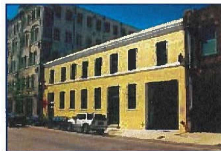
This building was constructed with a single pedestrian entrance in 1886, and a garage door was added later (left). When the building was rehabilitated for office use, an existing window was removed from the end bay and replaced with a new glazed entryway (center and right).
