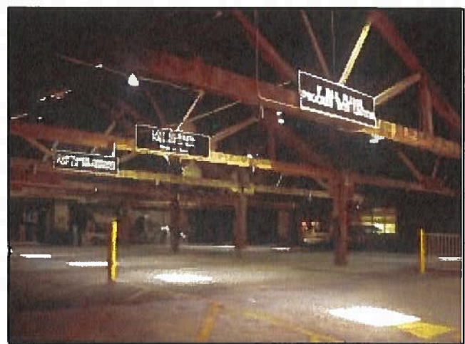
The historic heavy-timber trusses were left exposed in the parking area.
