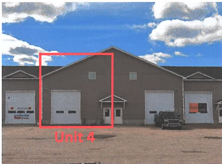
Unit #4 front view
