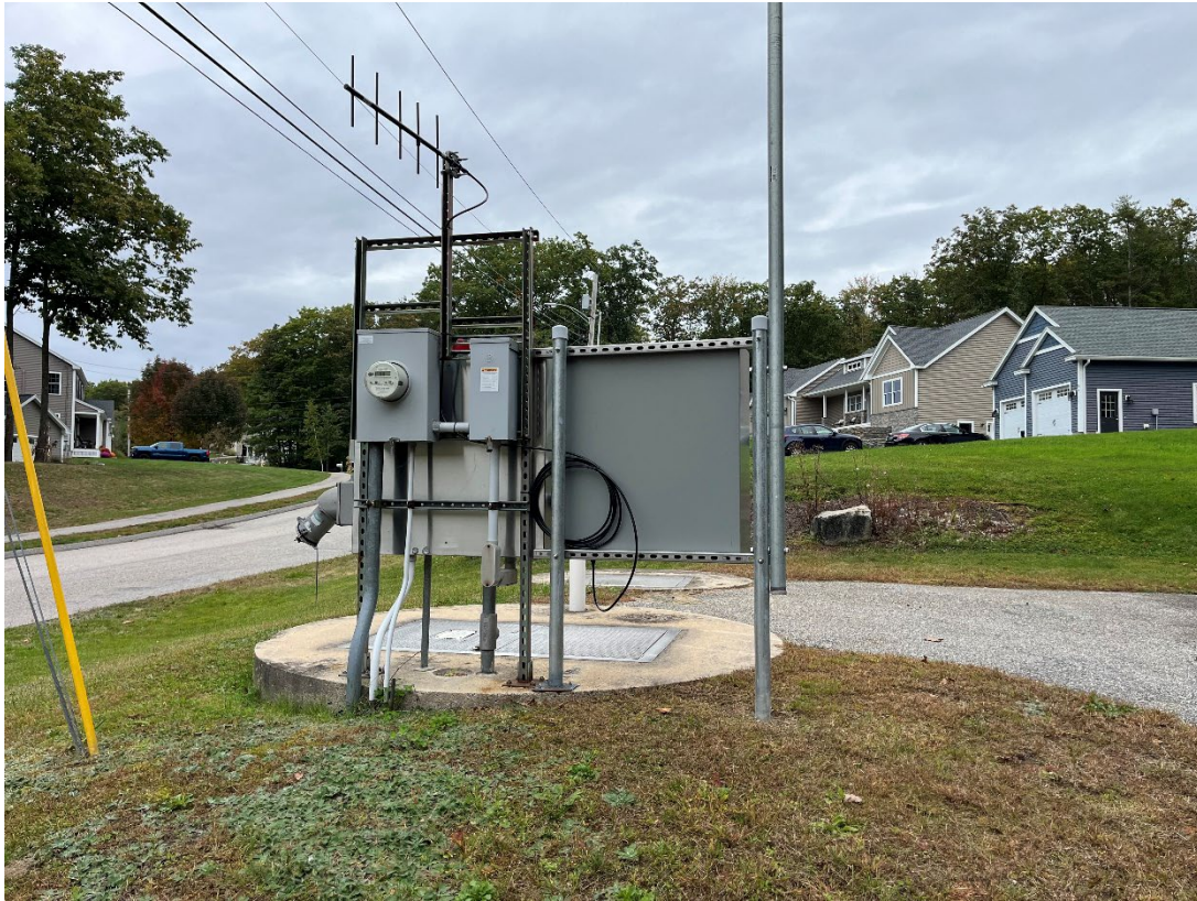
PHOTO 7 – EXISTING PUMP STATION ON PARKSIDE DRIVE.
