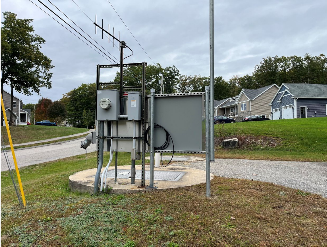
PHOTO 7 – EXISTING PUMP STATION ON PARKSIDE DRIVE.
