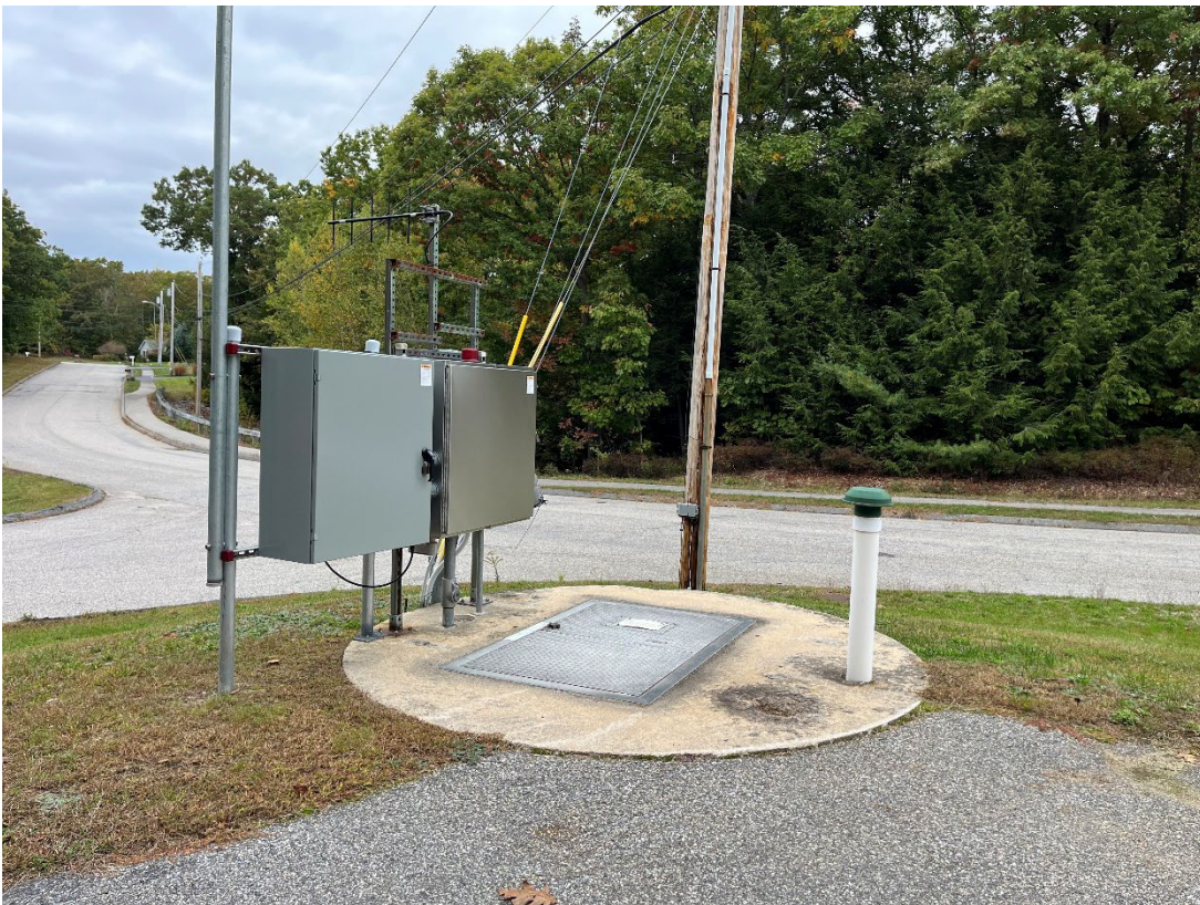
PHOTO 8 – LOOKING AT PUMP STATION AND PARKSIDE DRIVE DRIVEWAY.
