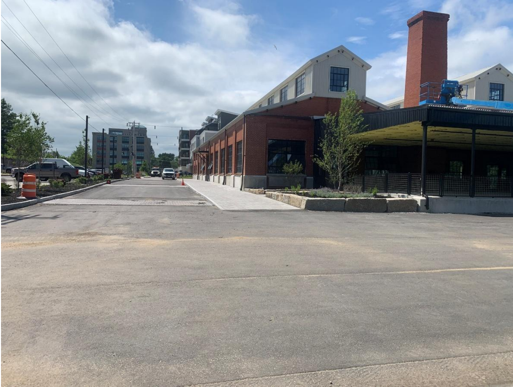
Photo 2: Overview of the 30 Upper Falls Road Building (right) facing west towards Elm Street
