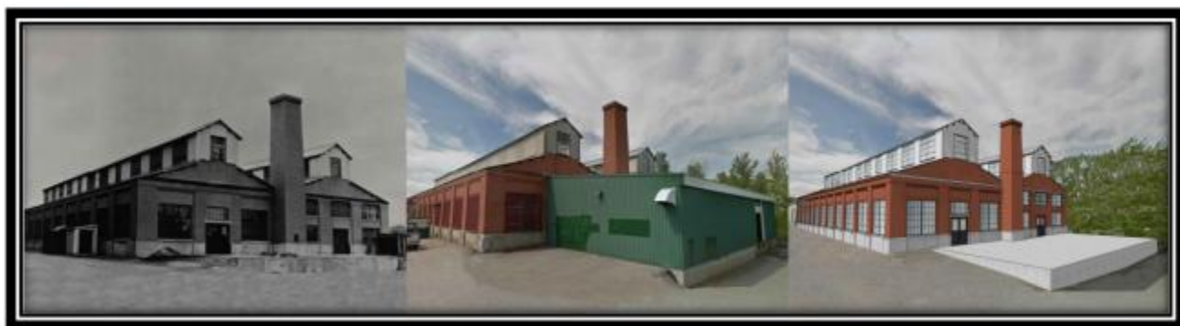
30 Upper Falls Road- Partial demolition and redevelopment of existing building (Photos: L to R: Historic, Pre-demo & Existing).
