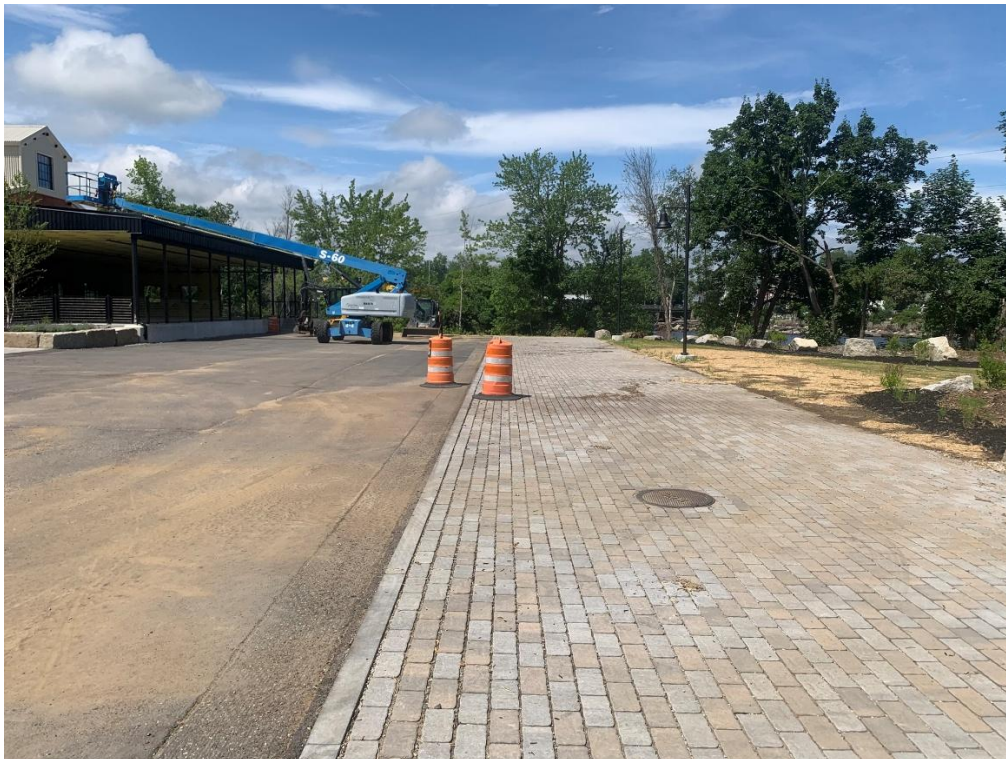
Photo 3: Overview of the 30 Upper Falls Road Building (left) facing north toward the Saco River.
