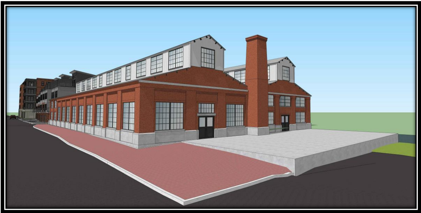
30 Upper Falls Road – East Elevation
