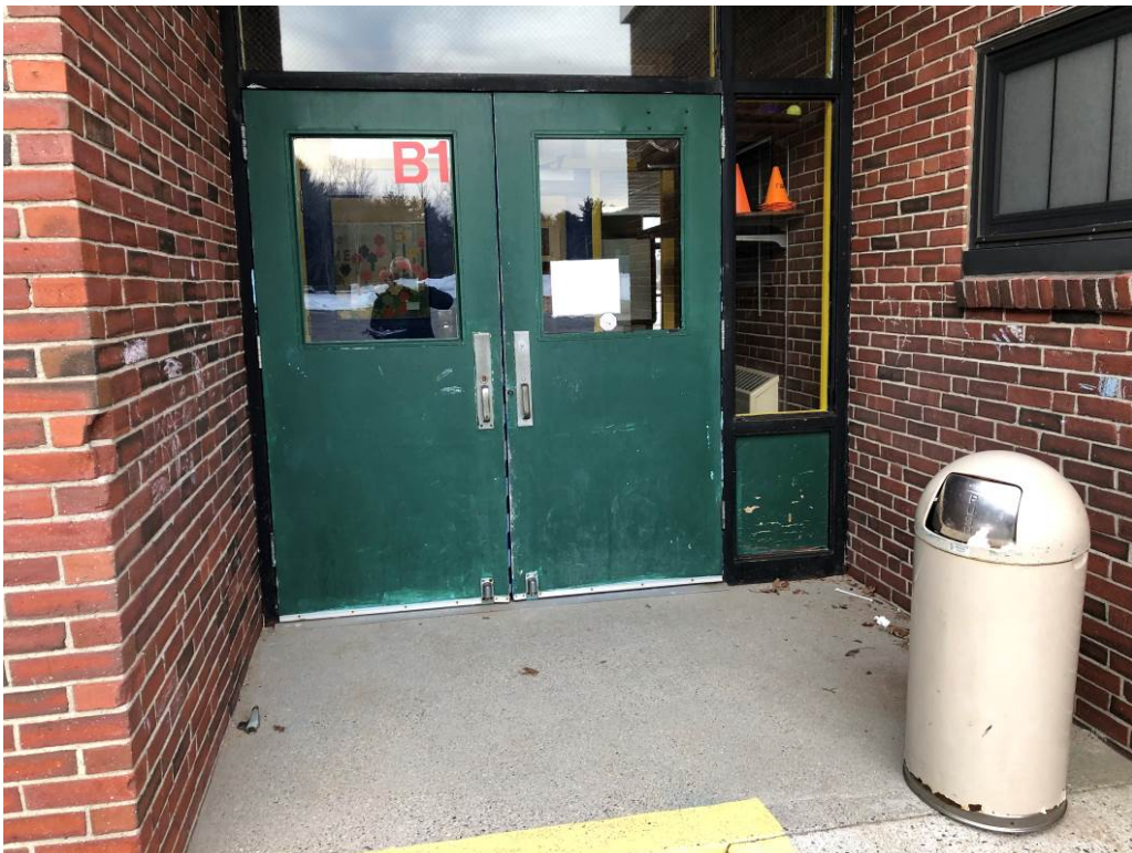
Architectural Photo 4 - Condition of exterior metal door.
