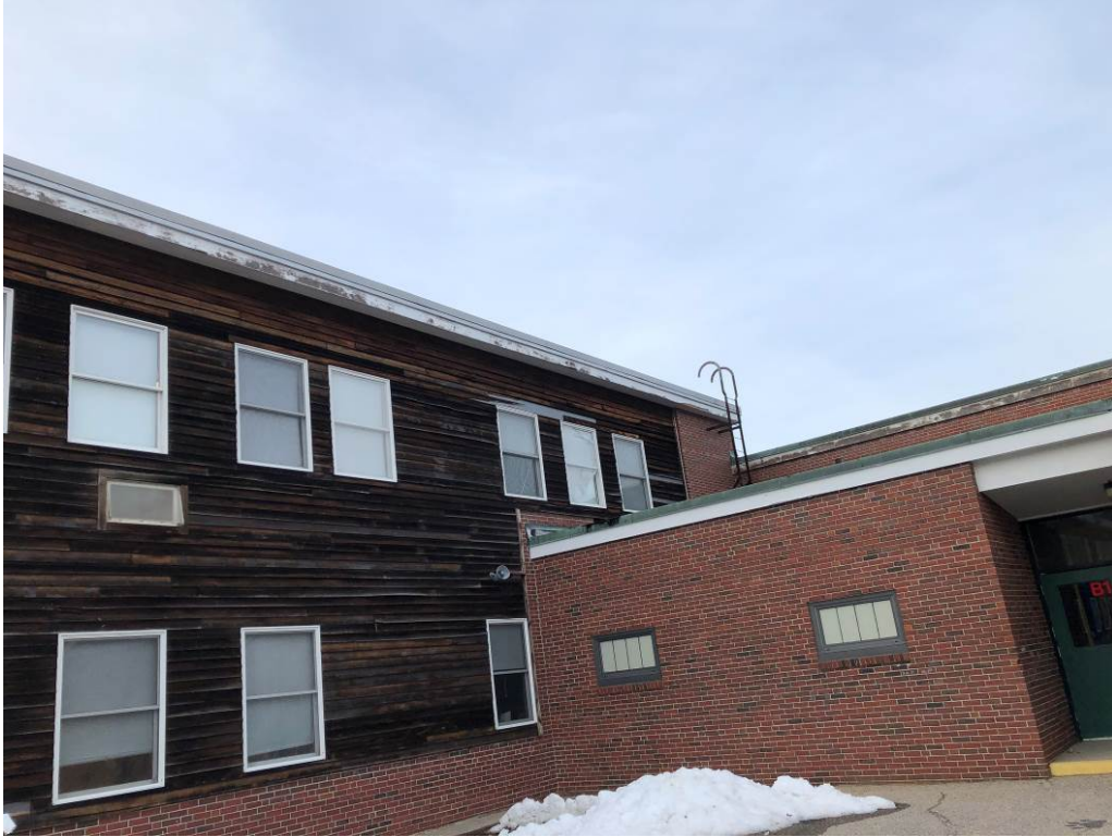
Architectural Photo 1 - Multi-level roof access by steel ladder.
