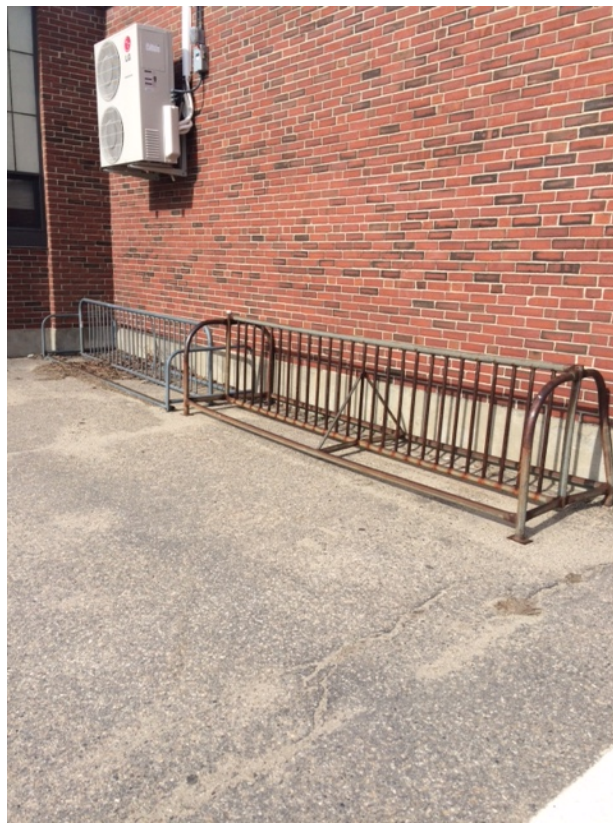
Civil Photo 8 - Bicycle racks.
