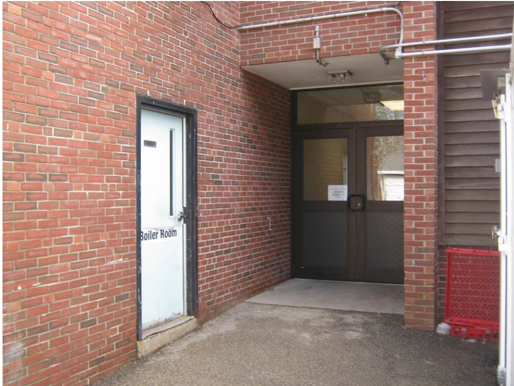
Civil Photo 15 - Entrance near boiler room.
