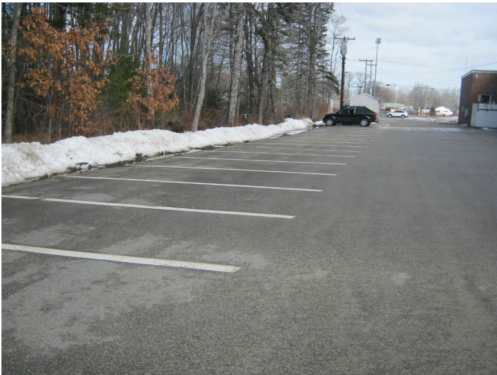
Civil Photo 2 - Parking area at north of building (north side).
