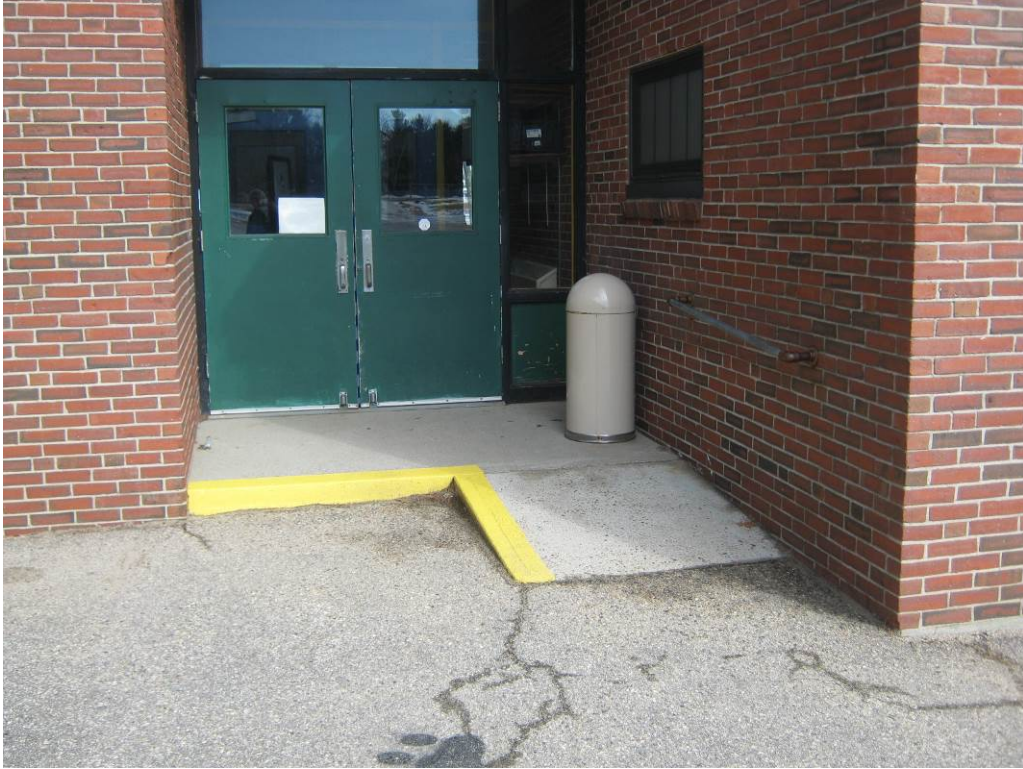
Civil Photo 13 - Curb ramp at Vestibule 2.
