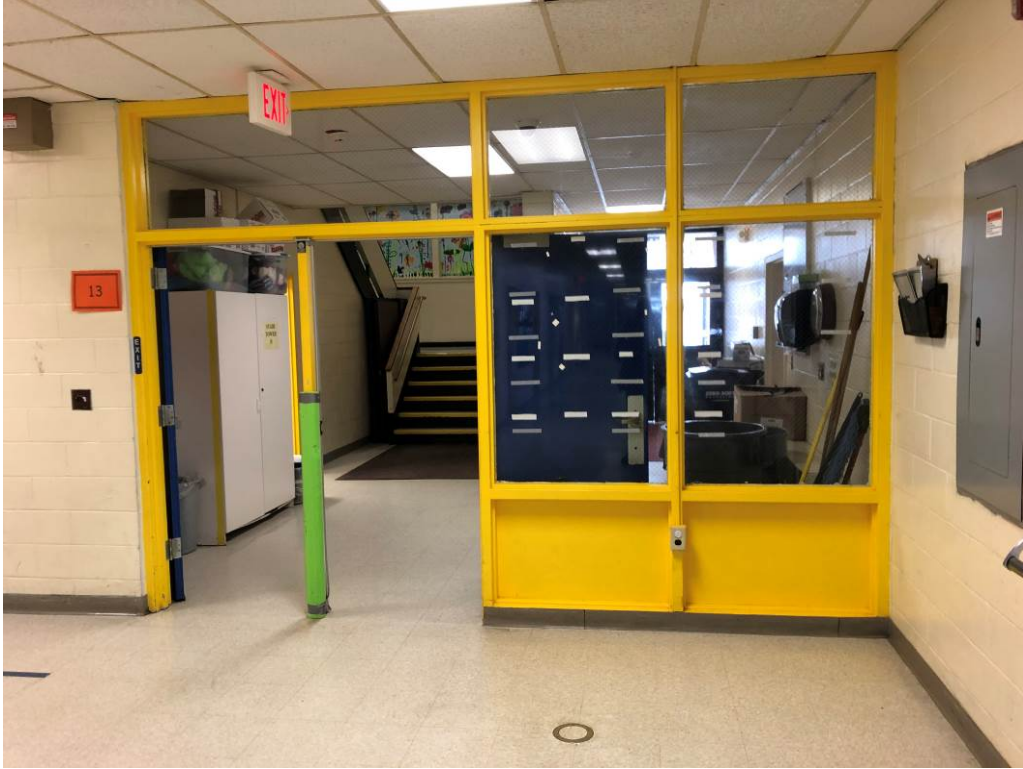
Architectural Photo 7 - Typical fire partition into stairwell enclosure showing wire glazing and painted plywood infills.
