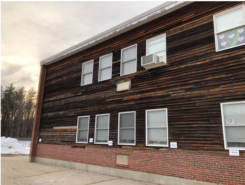
Architectural Photo 2 - Typical condition of clapboard siding and single hung windows.
