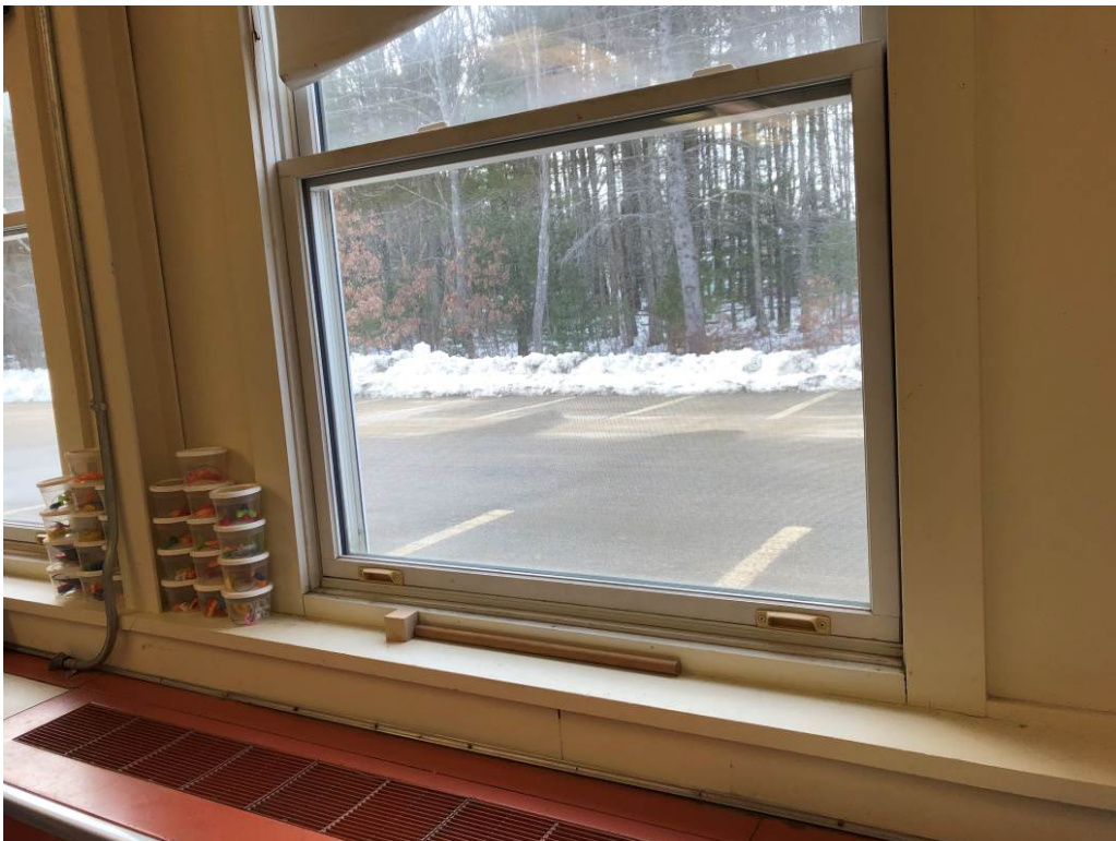
Architectural Photo 6 - Typical condition of single-hung vinyl-clad windows, and dowel used to hold them open.
