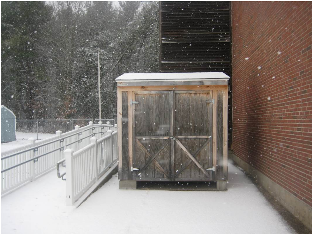
Civil Photo 34 – Storage building built/delivered sometime after Spring, 2016.
