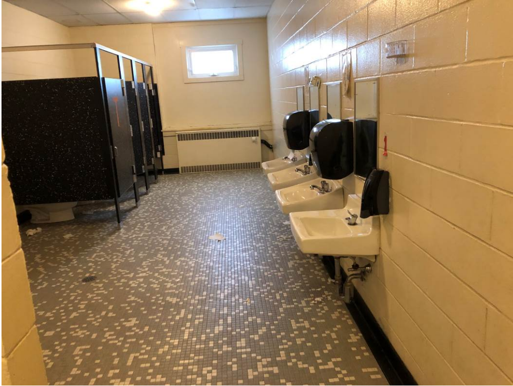
Architectural Photo 15 - Typical condition of multi-user toilet room, showing translucent window.
