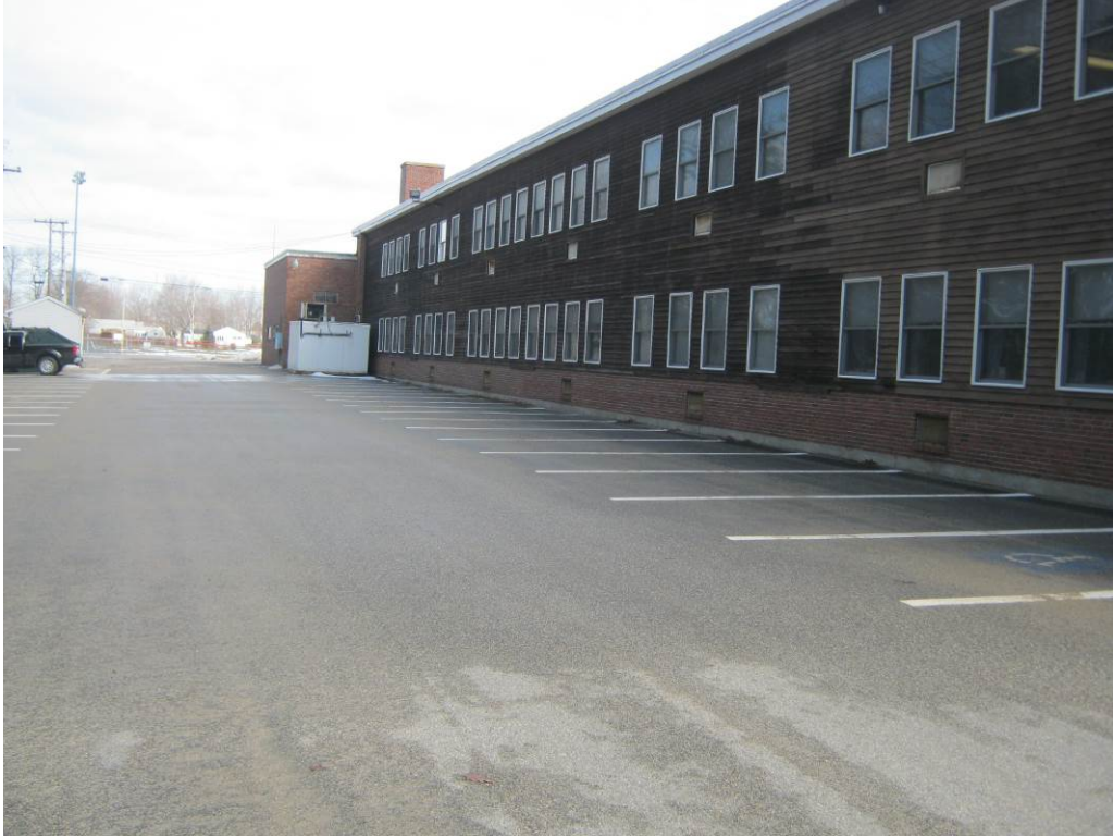
Civil Photo 1 - Parking area at north of building (south side).
