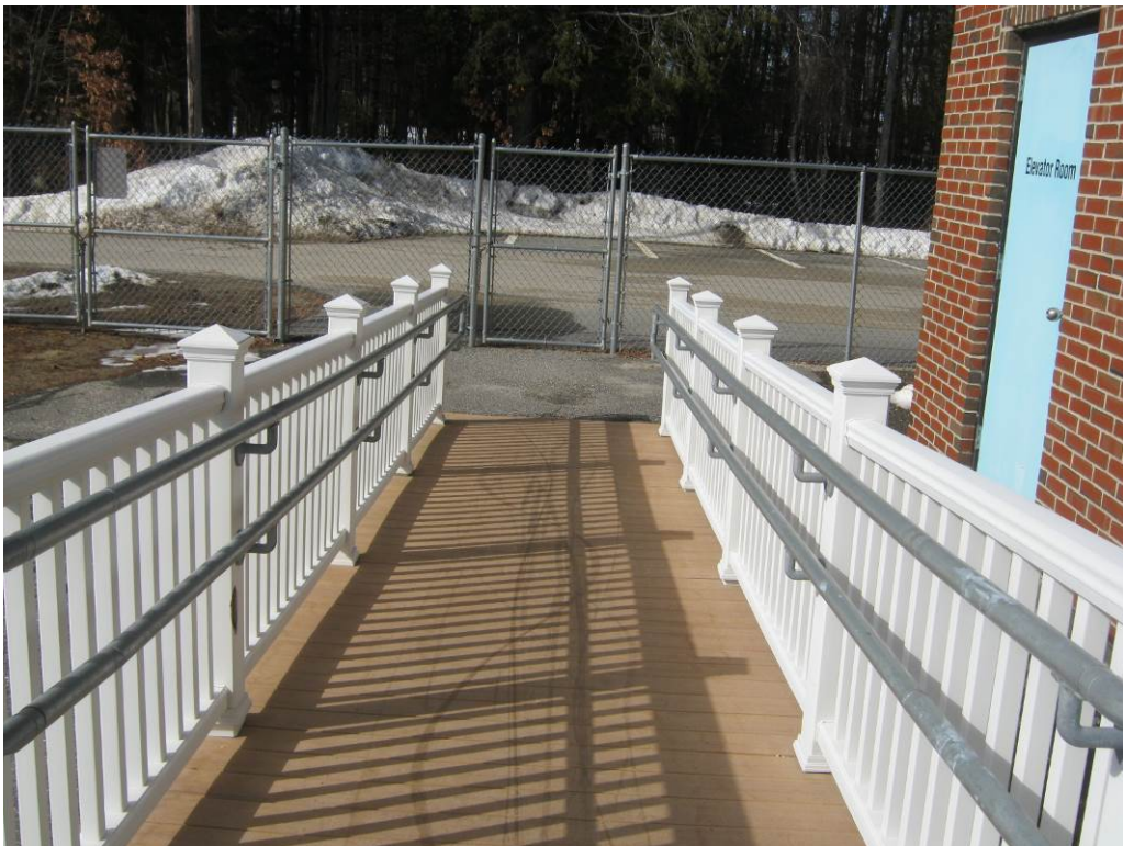
Civil Photo 14 - Composite wood ramp at west entrance.
