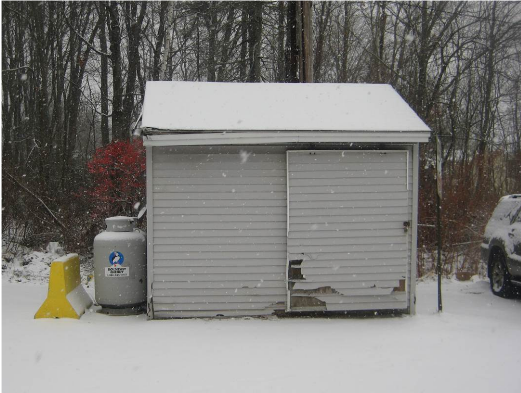
Civil Photo 33 - Storage shed and LP tanks.
