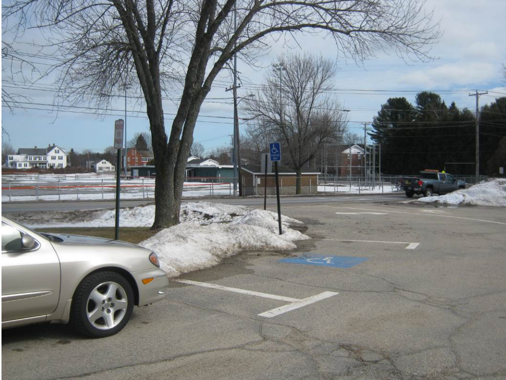
Civil Photo 7 - Designated accessible space at drop-off area.
