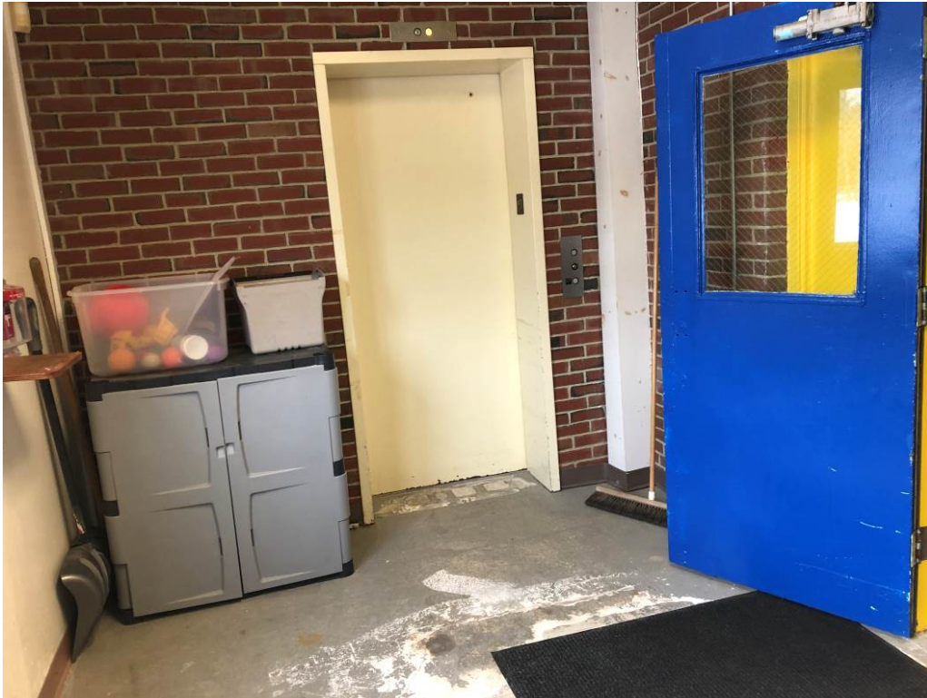
Architectural Photo 11 - Elevator lobby with partially removed floor tile.
