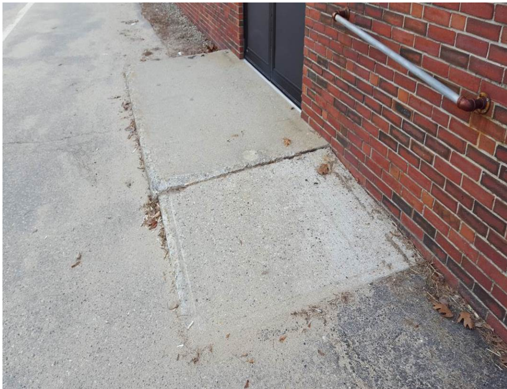
Civil Photo 12 - Curb ramp at multi-purpose room doors.
