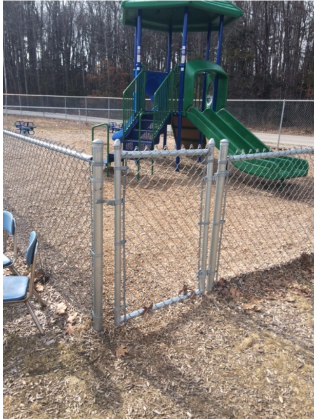
Civil Photo 17 – Chain link fence at Head Start playground.
