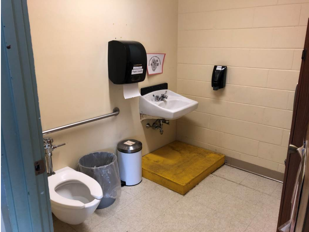
Architectural Photo 19 - Typical single-user classroom toilet.
