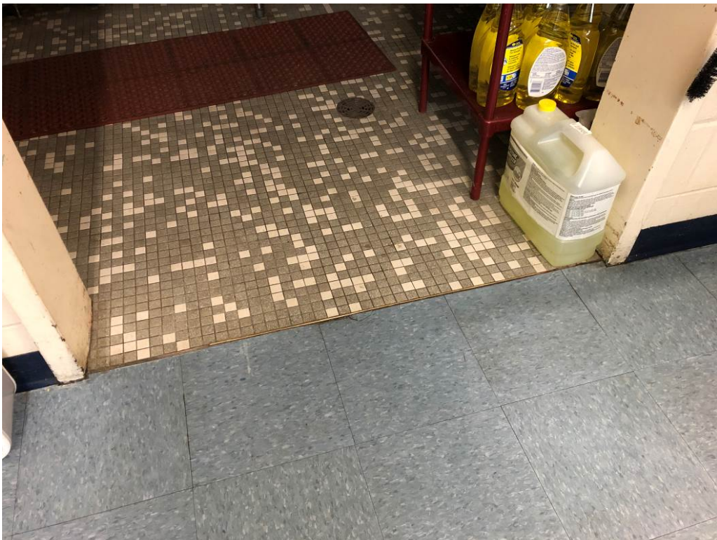
Architectural Photo 16 - Typical door threshold condition in kitchen.
