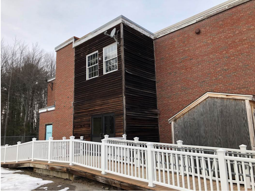
Architectural Photo 3 - Elevator addition with ADA access egress ramp.
