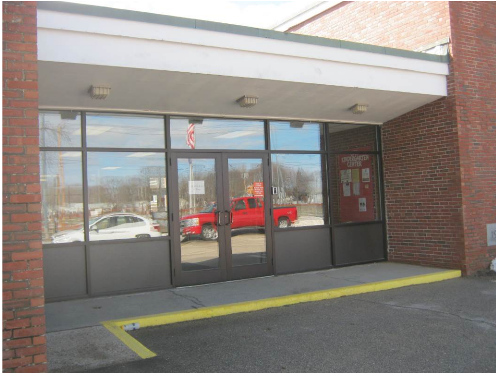
Civil Photo 11 - Main entrance.
