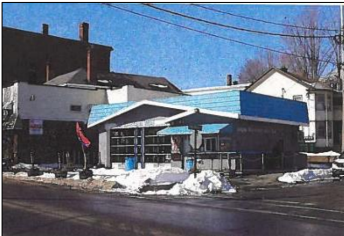
The building as it appeared in the Kleinfelder Survey, 2022
