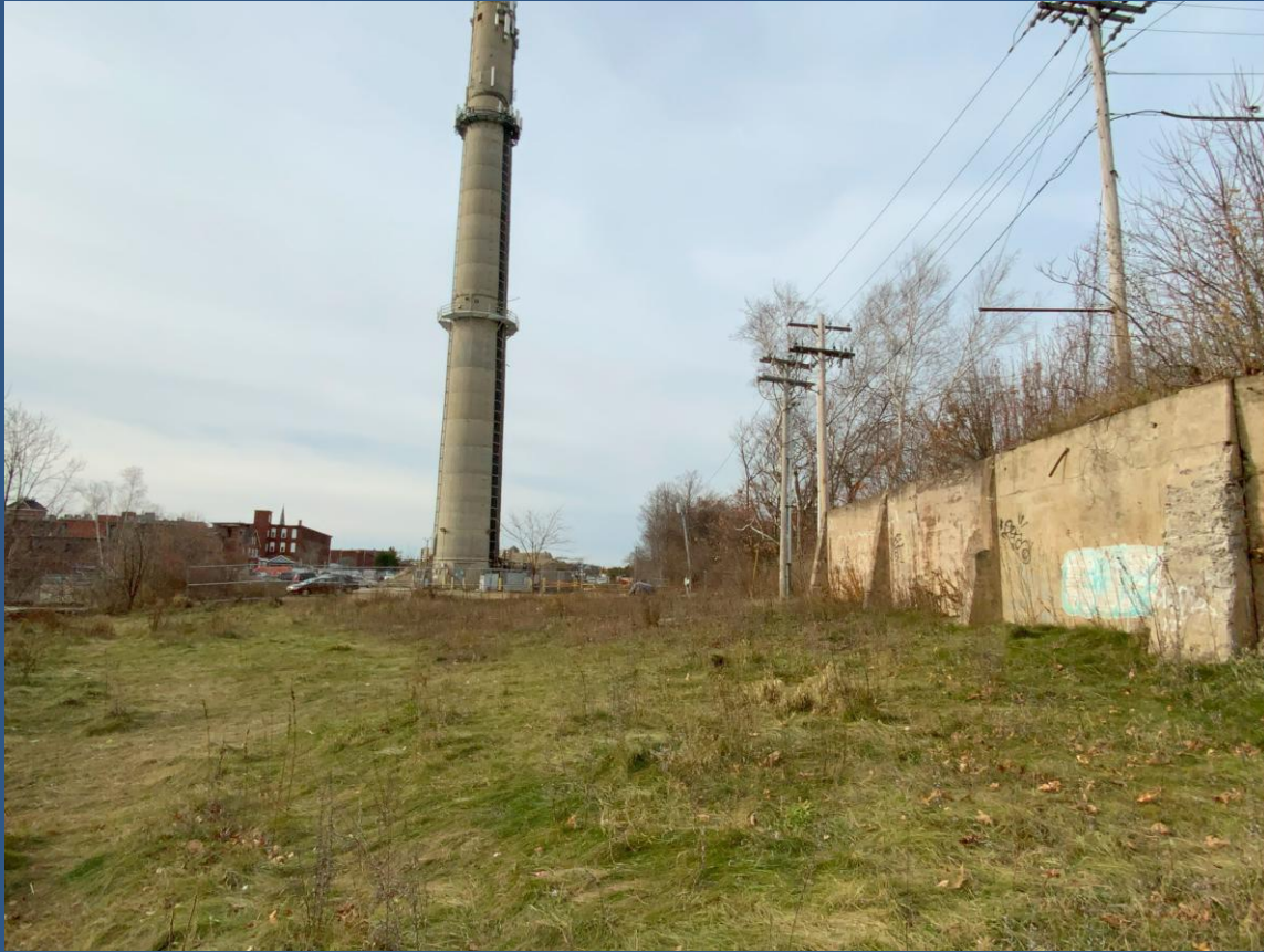
Biddeford Approach — Looking West
