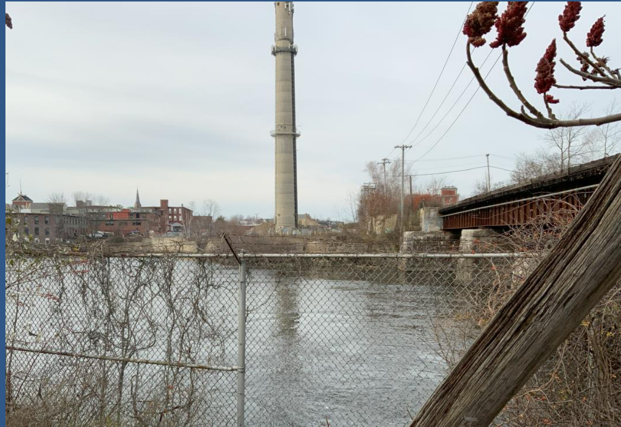
Saco Approach — Looking West (at river)
