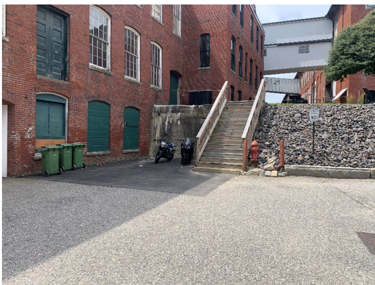
Figure 2: View of the north face of Building 19 (left side of image) facing west.
