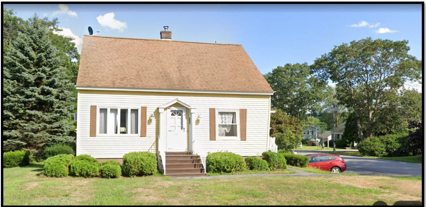
Figure 1: 179 Granite Street - Front Elevation
