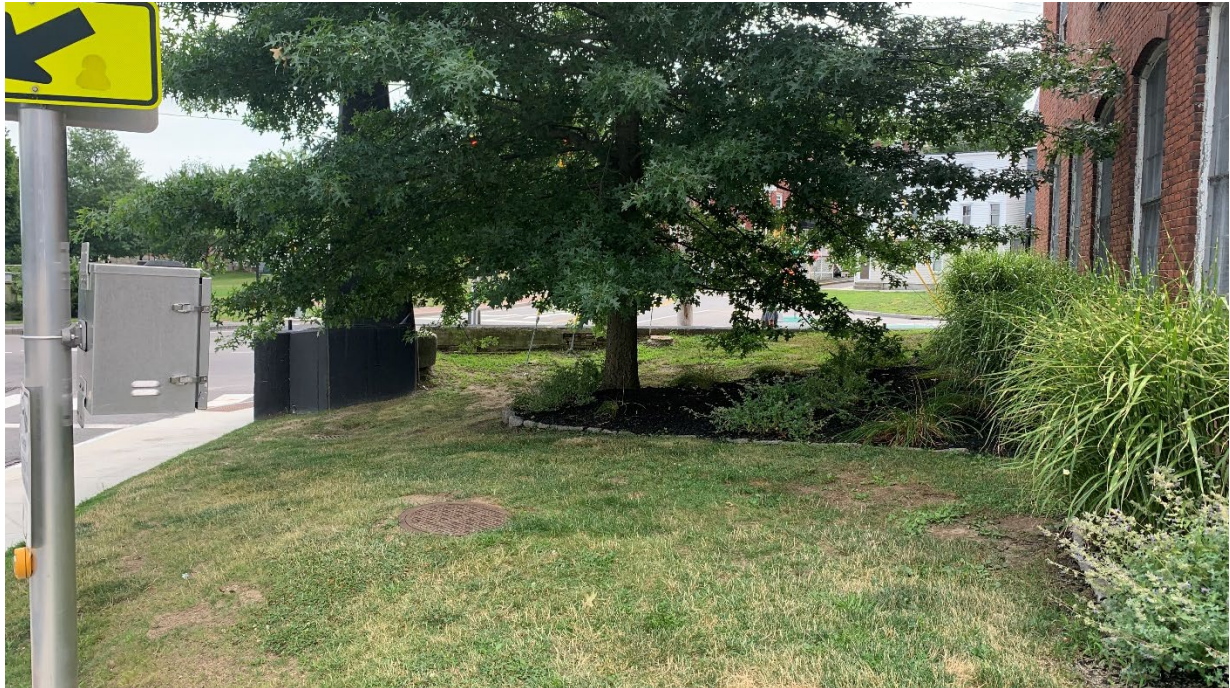
Figure 3: View of the east face of Building 20 facing south.
