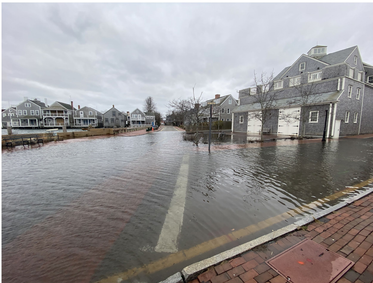
FIGURE 4 Flooding in Downtown Nantucket in Winter 2021.
