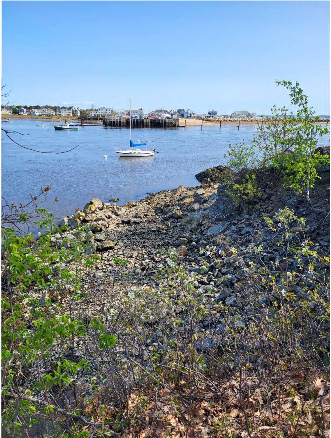
Photo3-Looking east at point from center of pier
