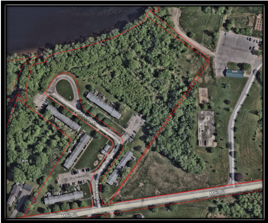
Forest Green Apartments – Existing Conditions
