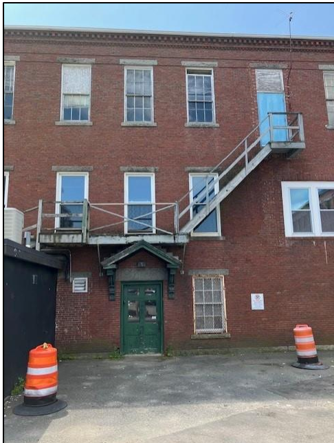
Existing Wood fire escape at North elevation
