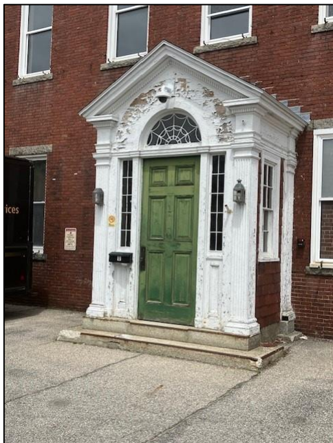
Existing Main Entry - South Elevation
