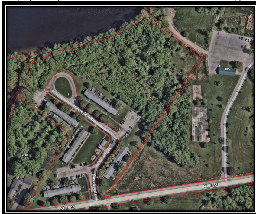
Forest Green Apartments – Existing Conditions
