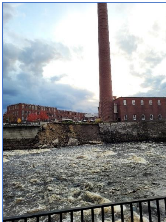
Figure 8 A section of the stone riprap along the Saco River in the Biddeford Mill District was damaged during an extreme precipitation event and subsequent high River flows in late October 2021. Credit: A. Sherwin
