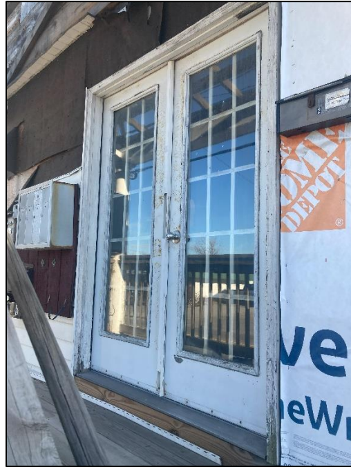
Existing conditions at front door
