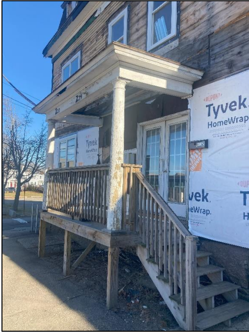
Existing conditions at porch
