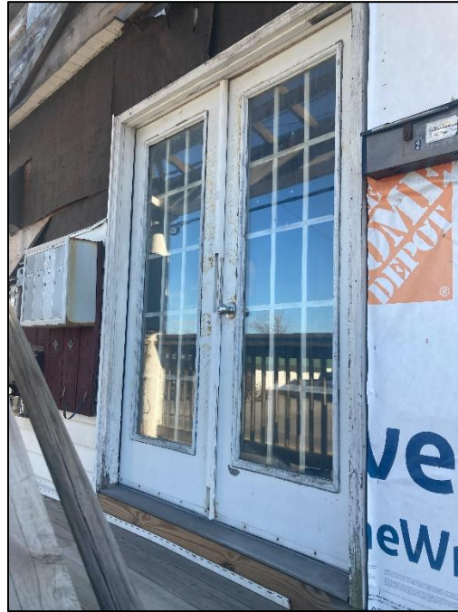
Existing conditions at front door
