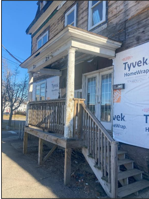
Existing conditions at porch
