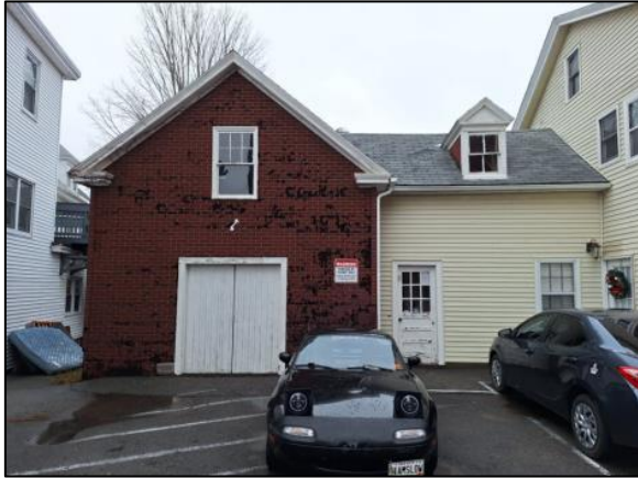
Southwest Elevation - Existing
