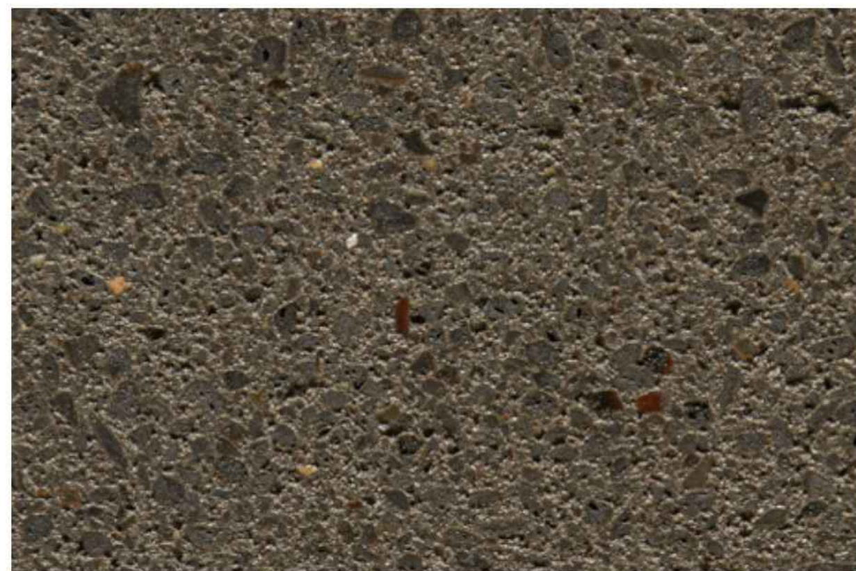
GROUND FACE CMU BASE
