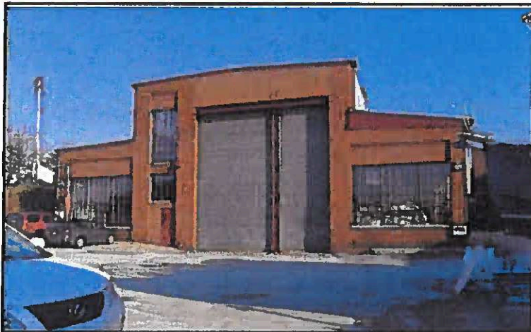
Portland Company Erecting Building Portland, Maine completed 1914
