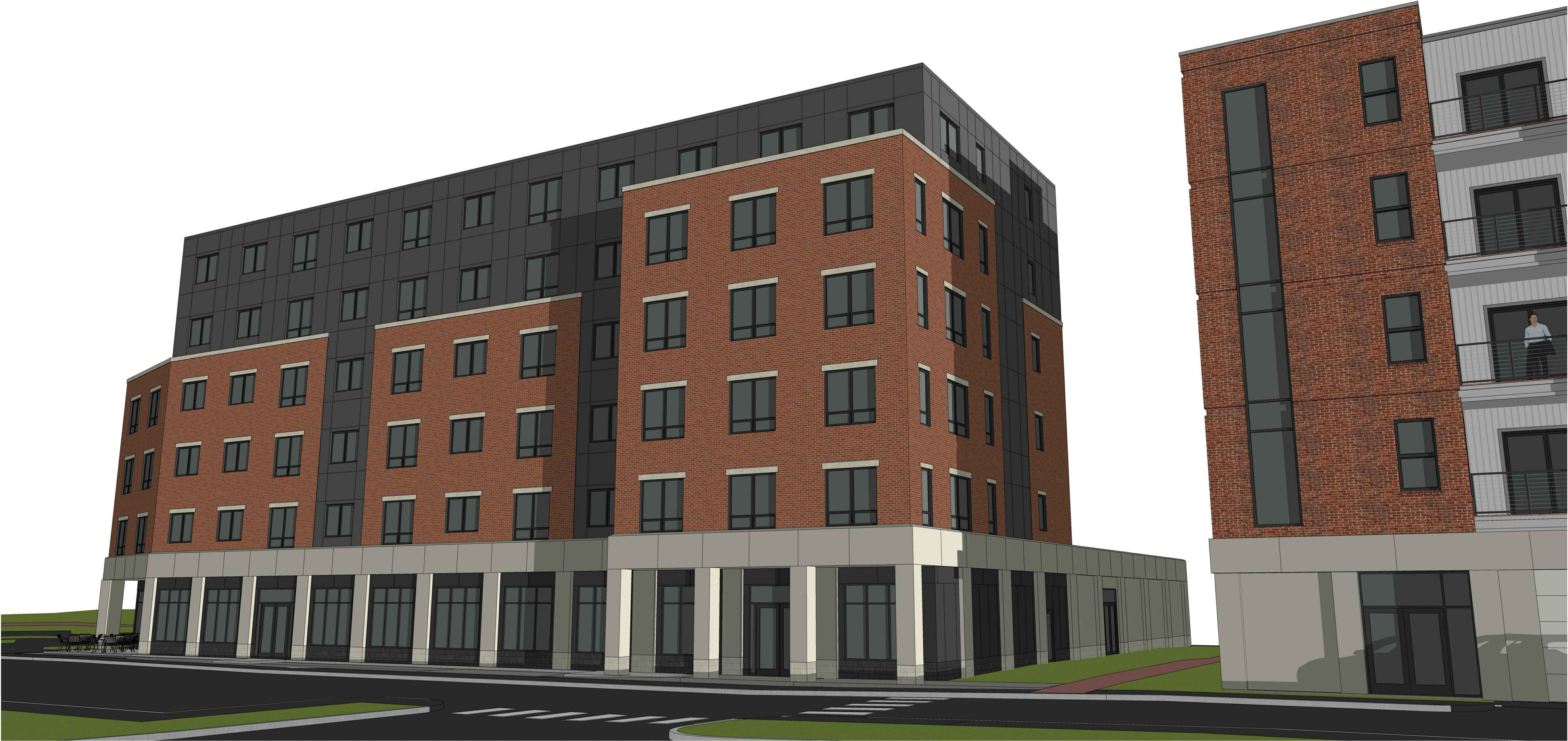
1 10 UPPER FALLS WAY - VIEW LOOKING NORTHWEST FROM UPPER FALLS WAY N.T.S.
