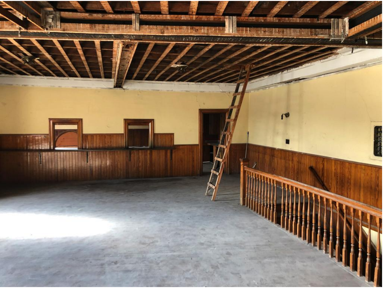
4TH FLOOR - EXISTING STAIR DOWN TO 3RD FLOOR
