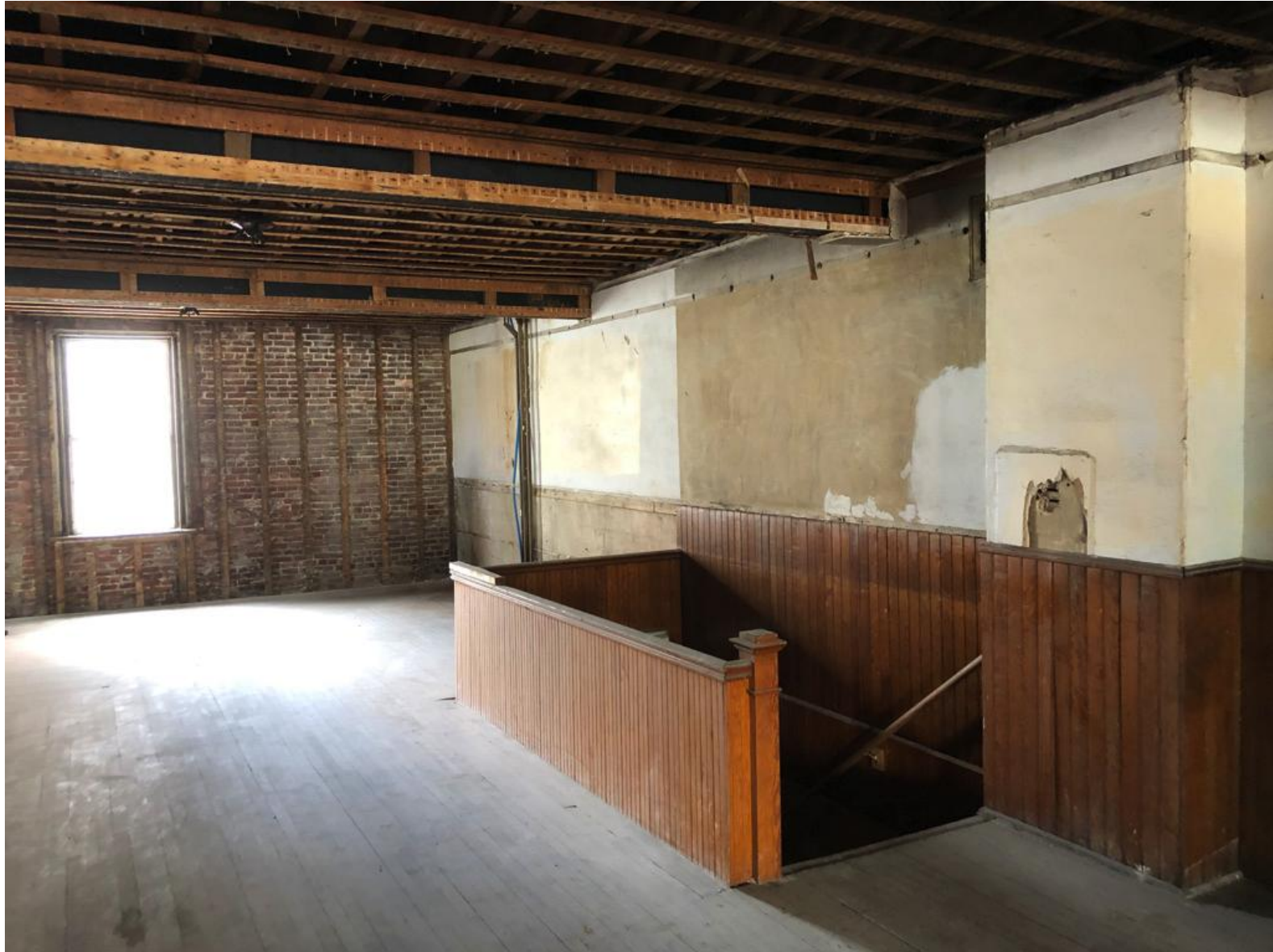
2ND FLOOR - LOOKING TOWARDS PROPOSED ELEVATOR
