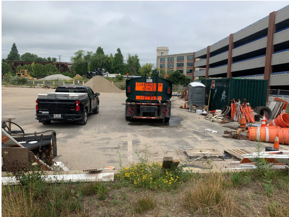
1. Standing west of existing parking garage. Facing north into lot 1.
