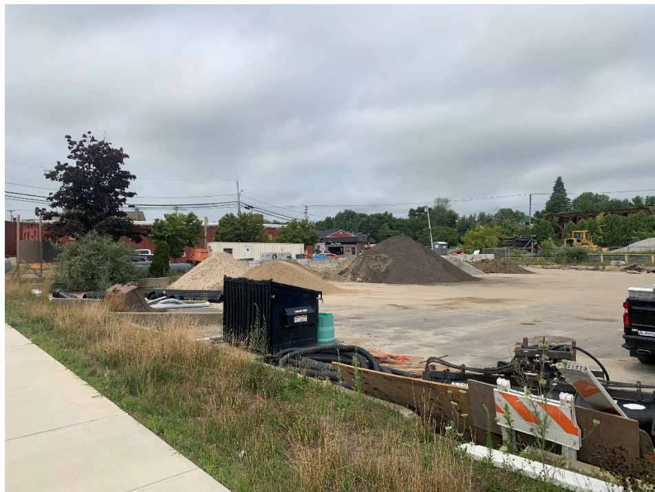
2. Standing west of existing parking garage. Facing northwest into lot 1.
