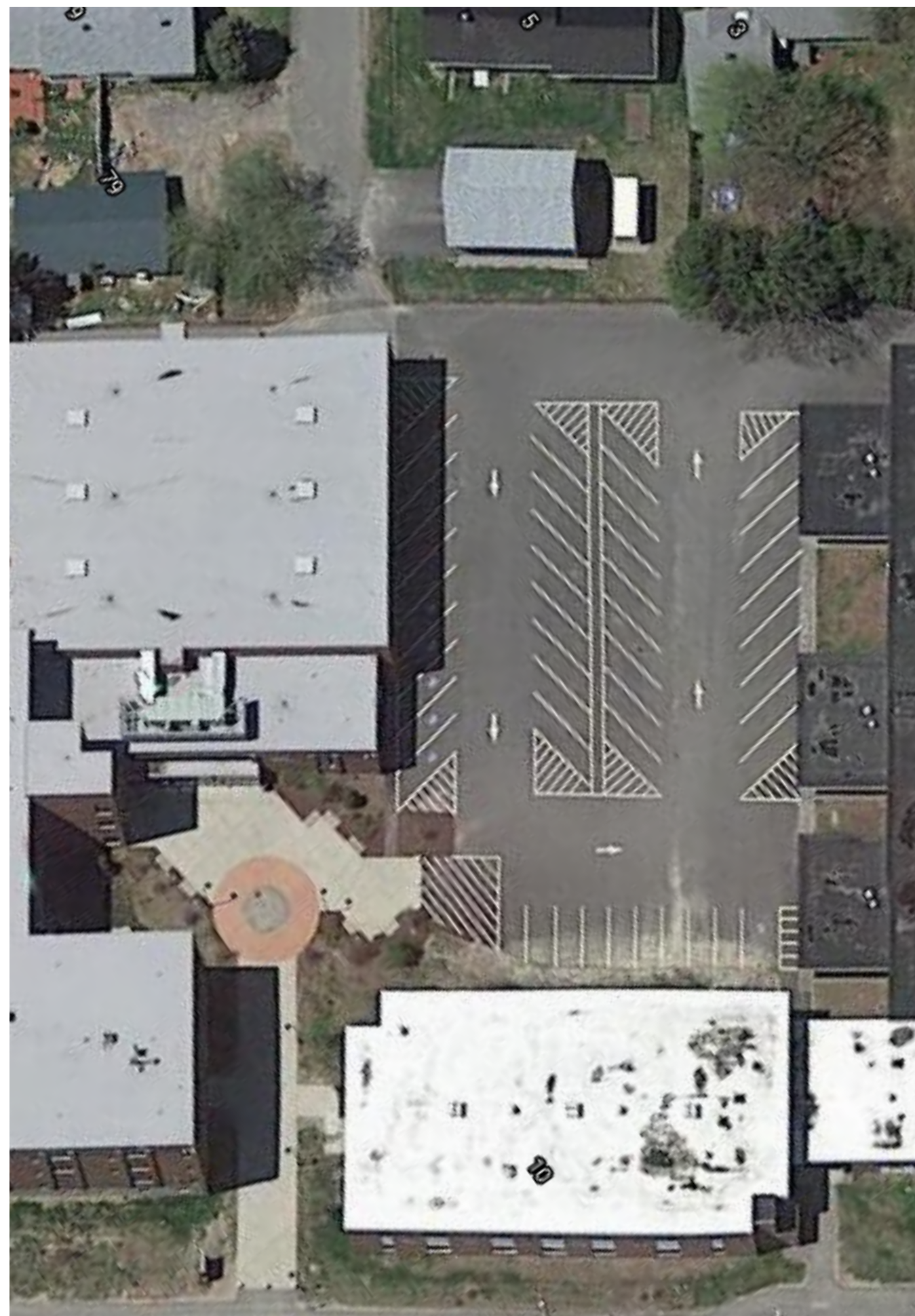
EXISTING PARKING AREA
