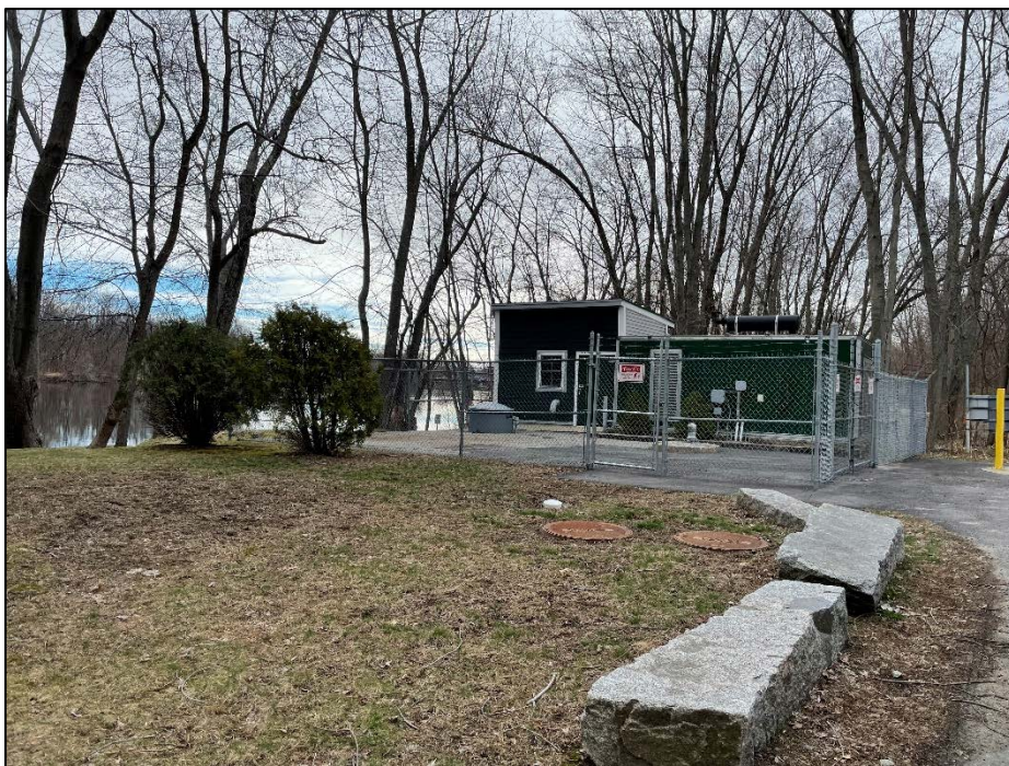
Photo 2: Existing pump station, to be demolished
