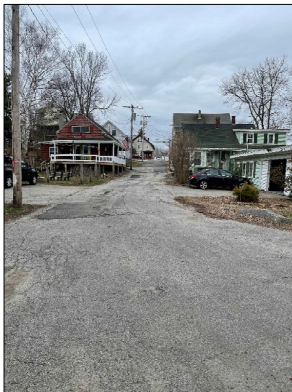
Photo 4: Existing Horrigan Court, to be repaved
