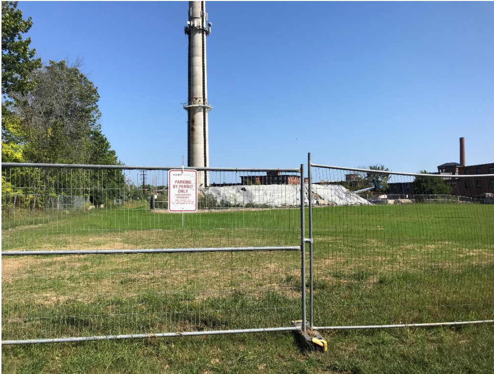
Figure 3. Standing east of existing parking garage, facing east toward Lot 3.
