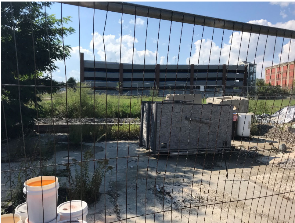
Figure 6. Standing near base of existing Cell Tower (Lot 4), facing west toward Lot 3 and parking garage (Lot 2).
