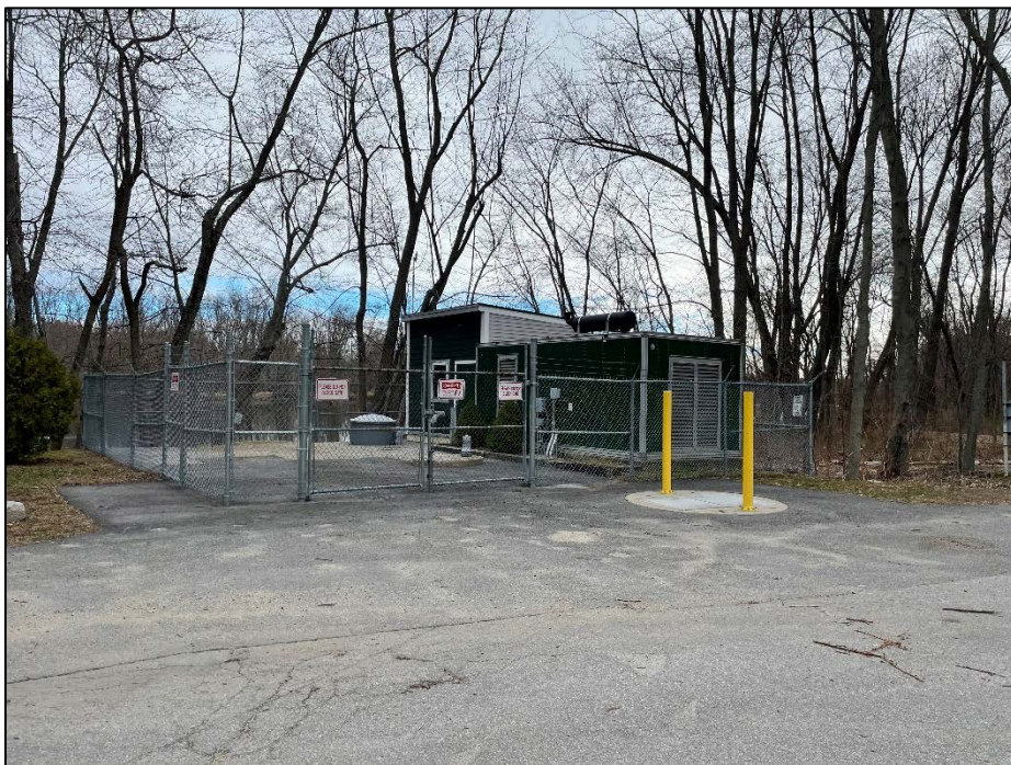
Photo 3: Existing pump station, to be demolished
