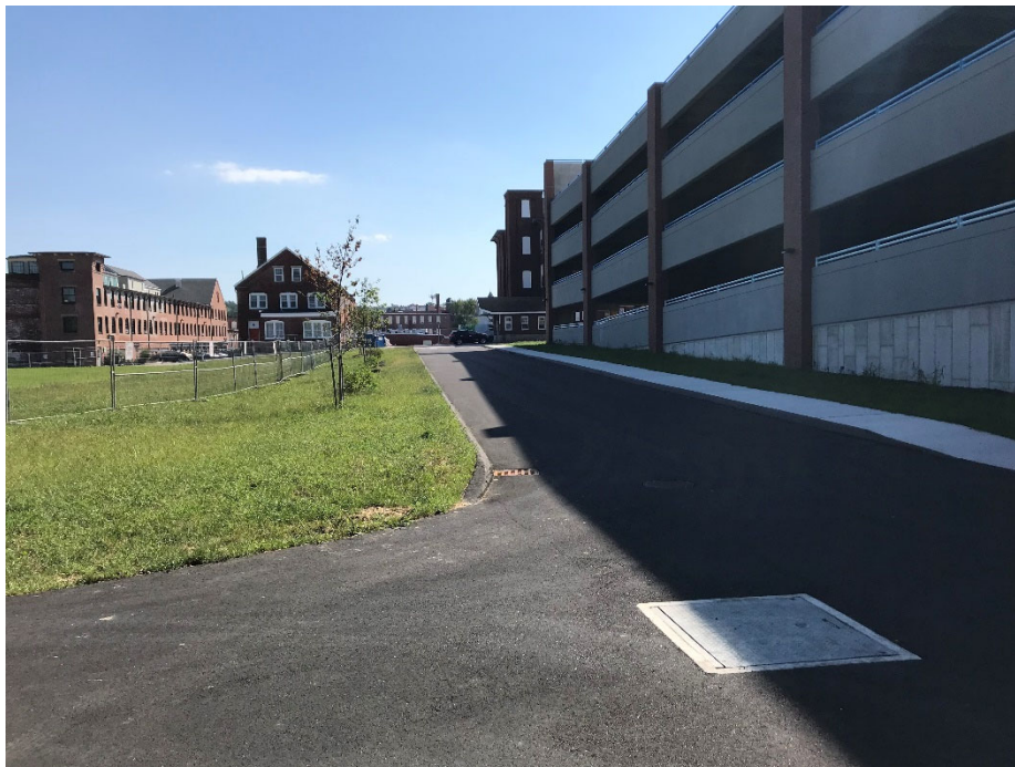
Figure 2. Standing east of existing parking garage, facing south toward Pearl Street. See Lot 3 on the left and Lot 2 on the right.
