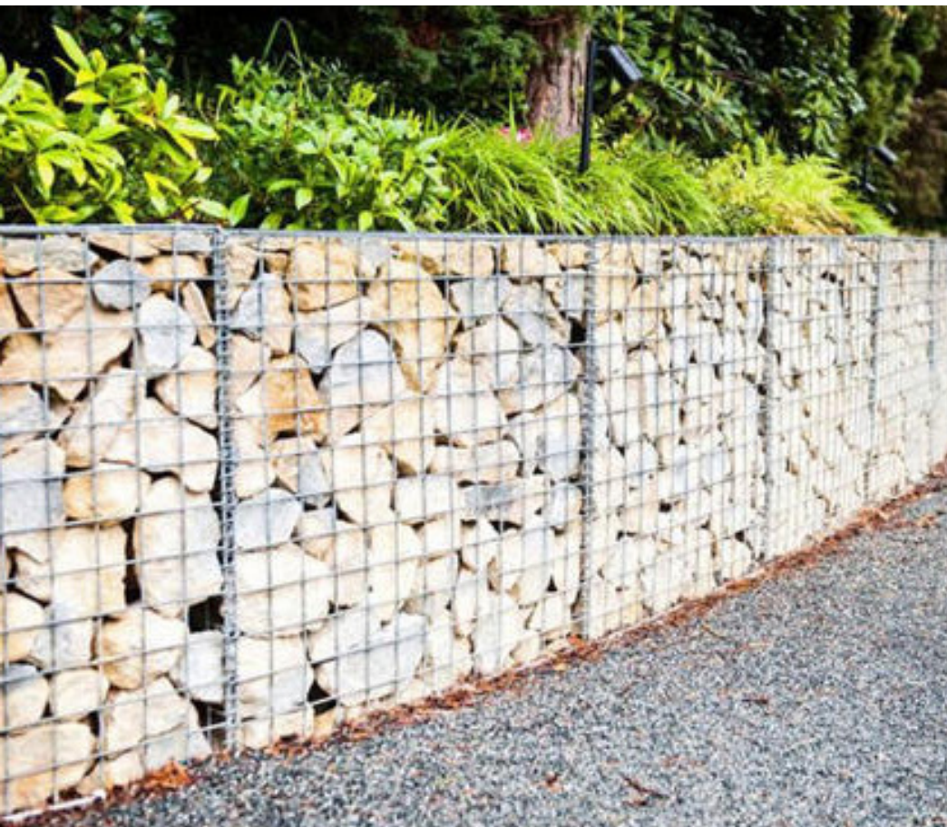
curved gabion walls
