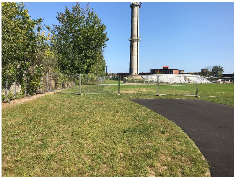
Figure 1. Standing east of existing parking garage on Smith Street, facing east toward the proposed Lot 3.
