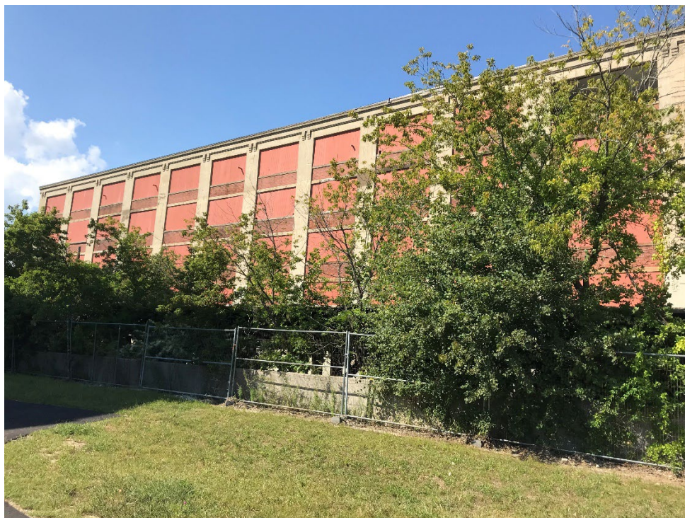
Figure 5. Standing east of existing parking garage, facing northwest toward the rear of Lot 3. See 1 Gooch Street building in background.
