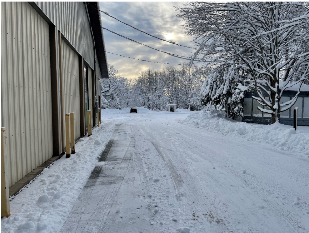
PHOTO 4 – LOOKING EAST ALONG SOUTH SIDE OF BUILDING (STORE ENTRY).
