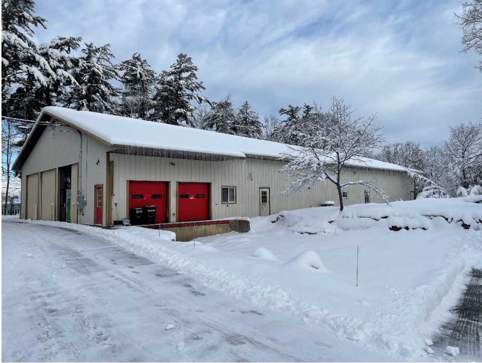
PHOTO 3 – LOOKING NORTH AT EXISTING BUILDING, PROPOSED MAIN ENTRANCE TO THE STOREFRONT LOCATED ON SOUTH FACING (LEFT SIDE OF PHOTO).
