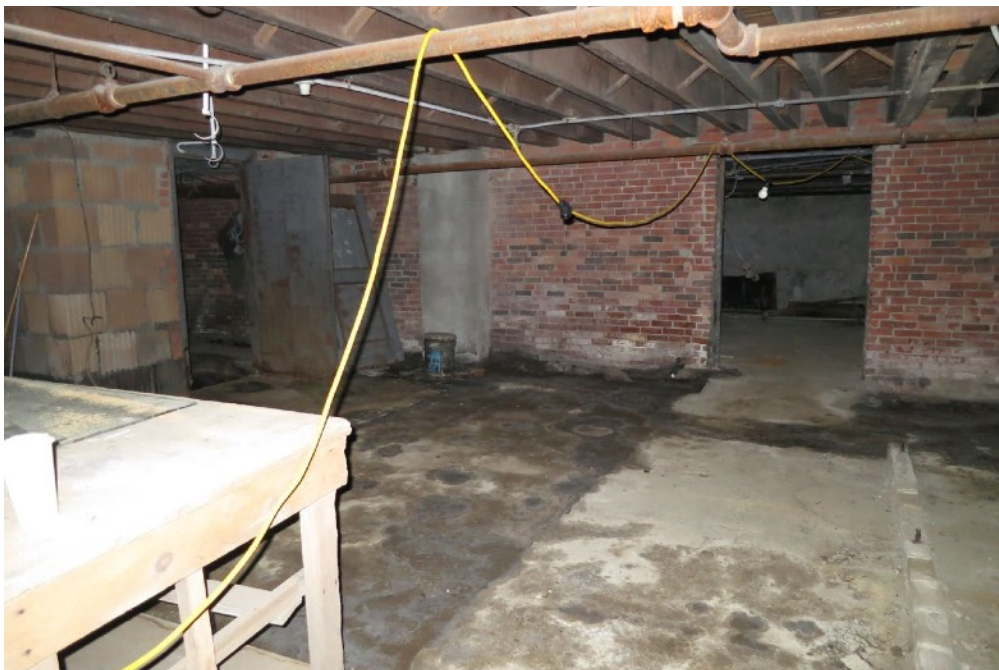
27 | Basement - view west in main block
