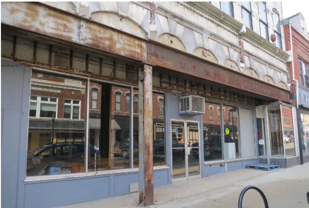
3 Facade (North Elevation) - detail of storefronts
