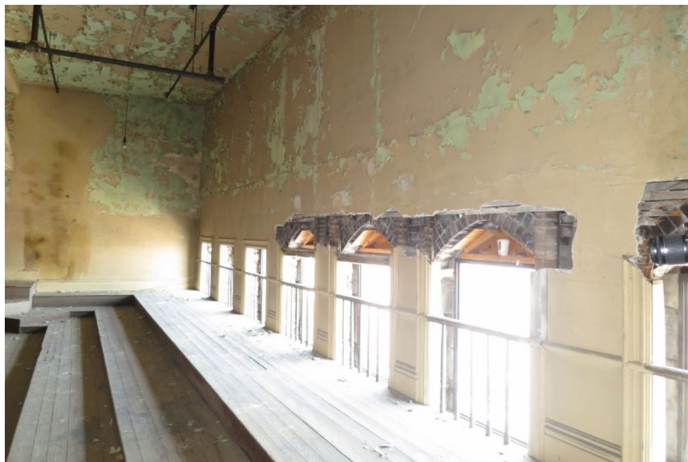
70 | View along north wall in gallery of assembly space
