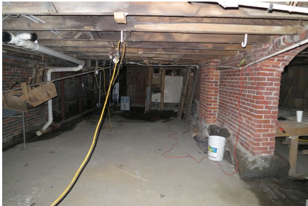
26 | Basement - view south in main block
