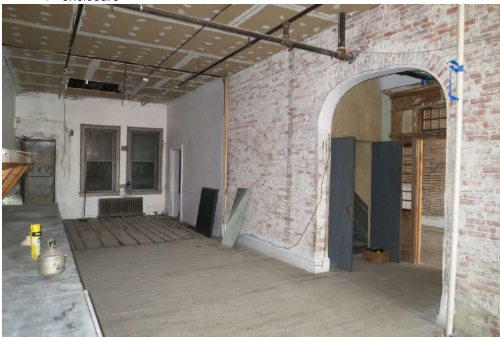
43 | Second Floor - view toward rear (south) at east side of building
