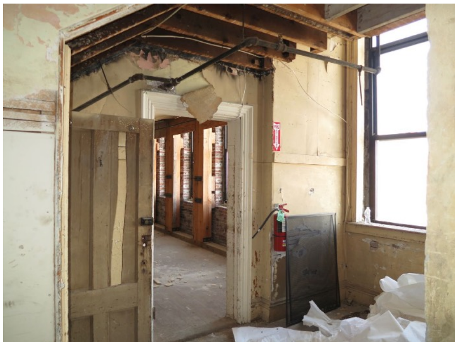
57 Third Floor - view toward north entry to assembly space
