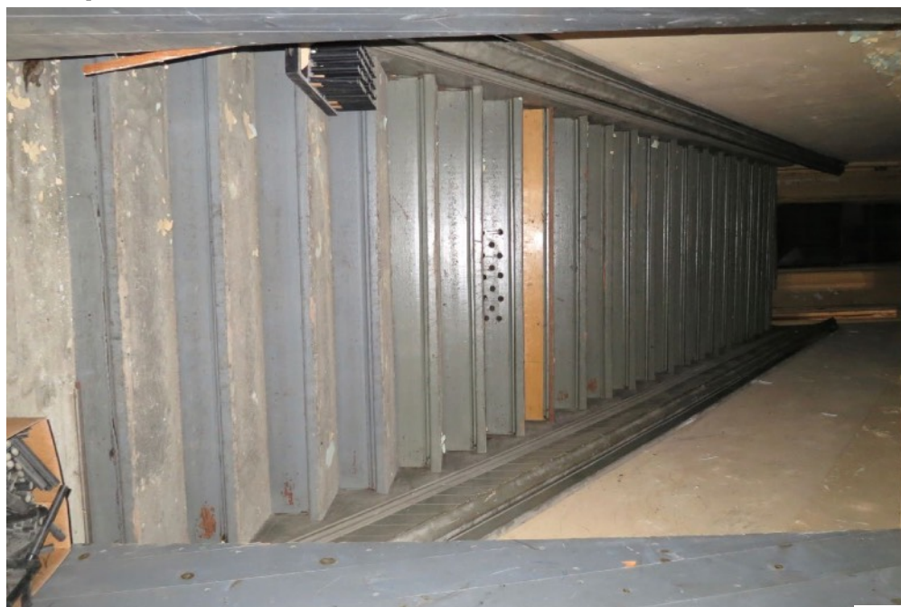
44 | Second Floor - historic stair to third floor
