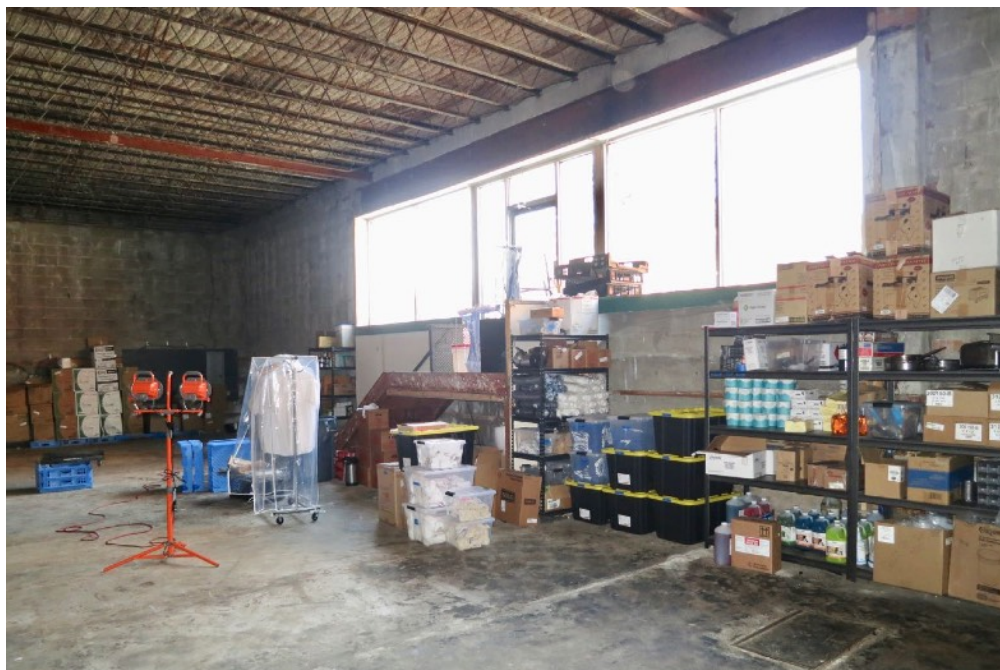
37 First Floor - view along storefront in ca. 1950 addition
