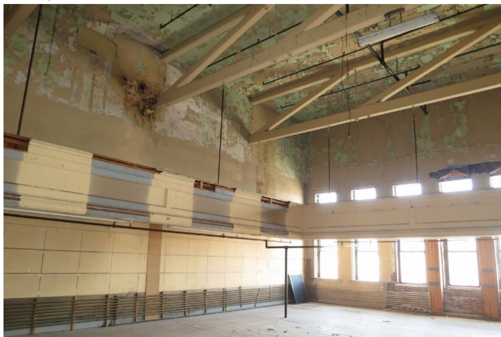
60 Third Floor - view northwest in assembly space
