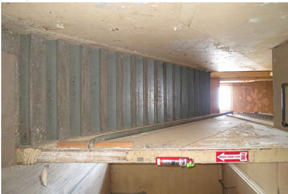
55 | Second Floor - stair to fourth floor (gallery level of assembly space)
