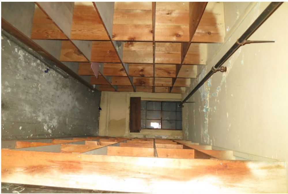
63 | Third Floor - storage room in southwest corner
