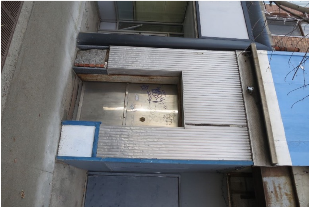
5 | Facade (North Elevation) - detail of added elevator enclosure
