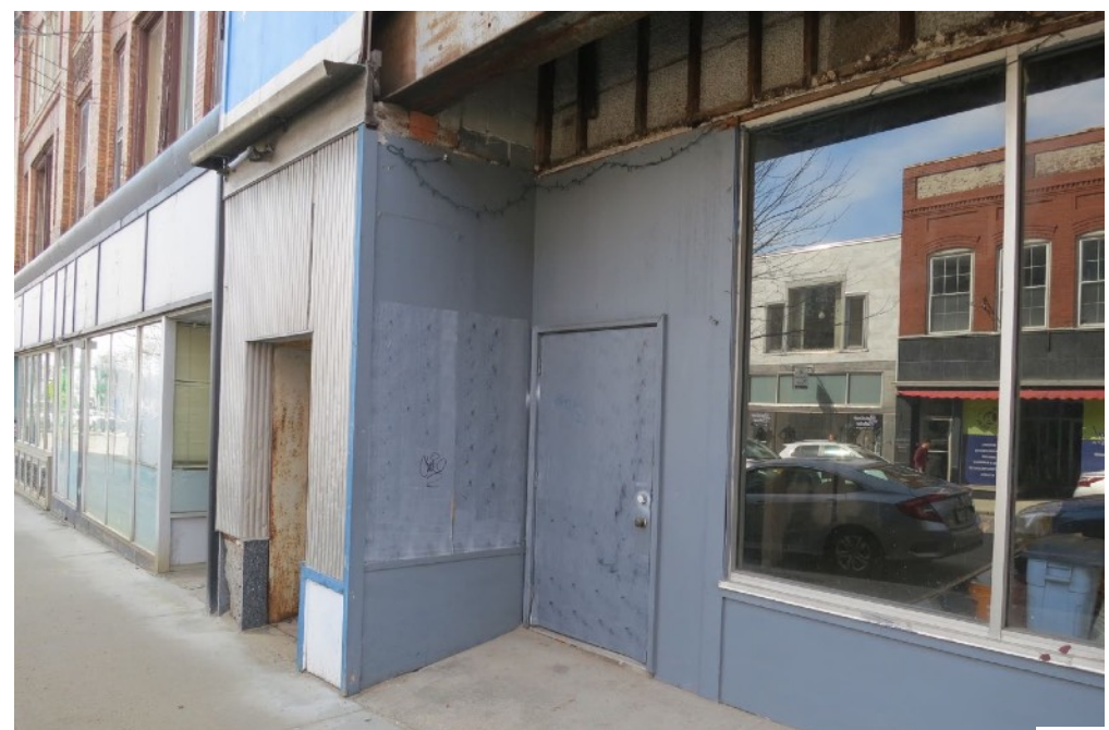
4 Facade (North Elevation) - view toward added elevator enclosure at e end
