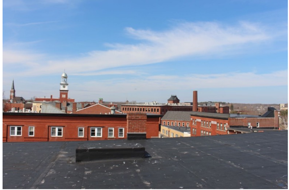
22 | Main Block - roof
