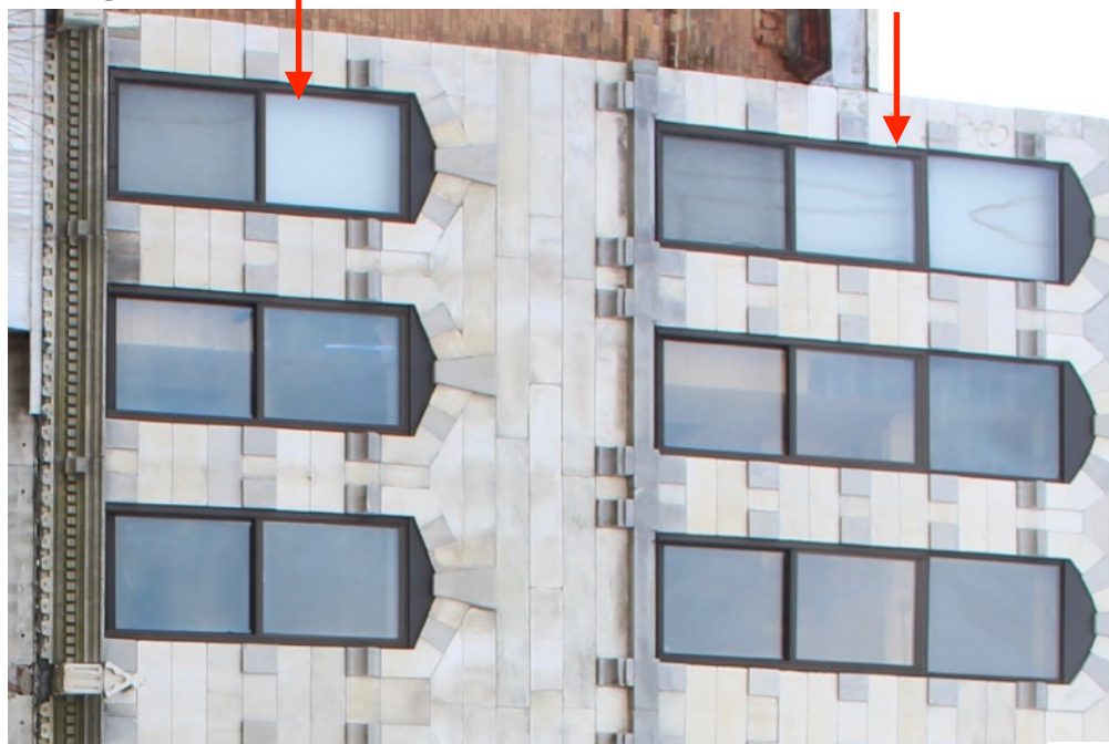
72 | Facade detail showing blocked windows (on interior) in easternmost b 123
