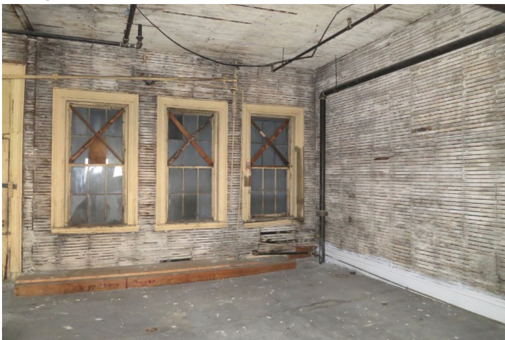
51 | Second Floor - view toward southwest corner
