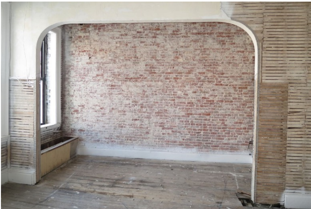
45 | Second Floor - view toward former stairhall
