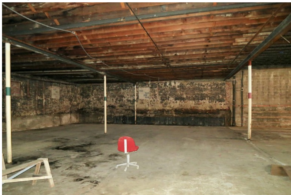
39 First Floor - view south in ca. 1929 addition
