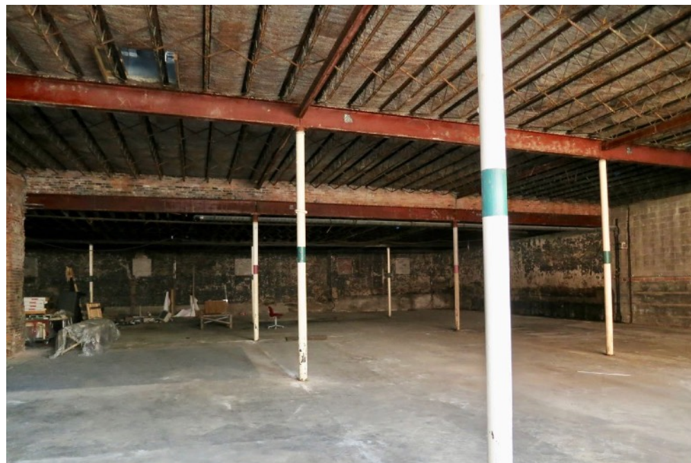
38 First Floor - view east in ca. 1950 addition, toward ca. 1929 addition
