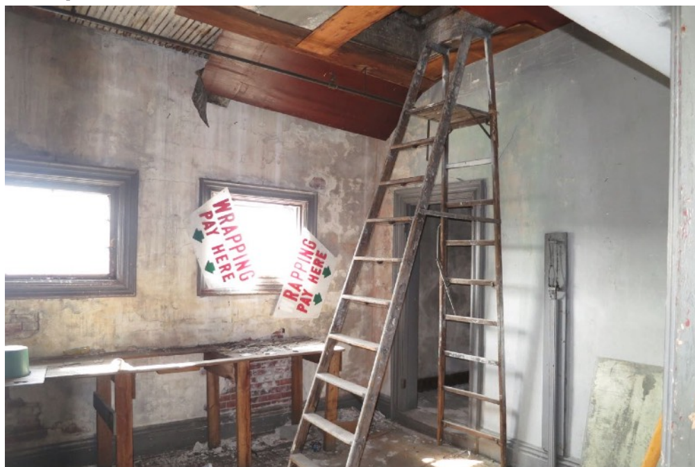
68 | Mezzanine - southeast room
