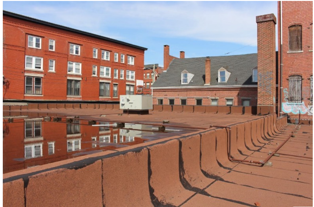
24 | Circa 1950 Addition - roof
