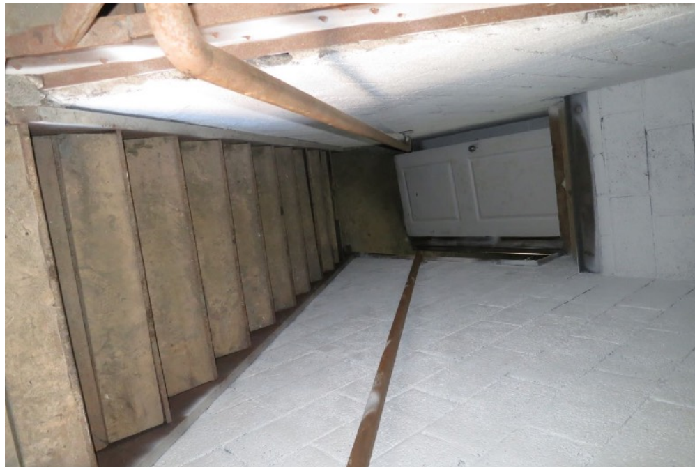
34 | First Floor - added stair to basement in northeast corner
