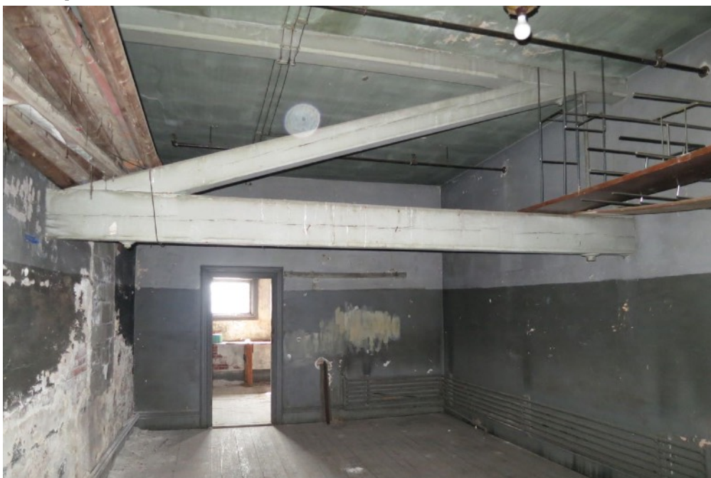
67 | Mezzanine - central room along east wall
