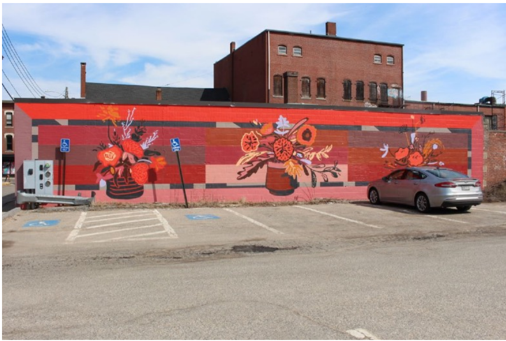
19 | Circa 1950 Addition - south elevation at west end
