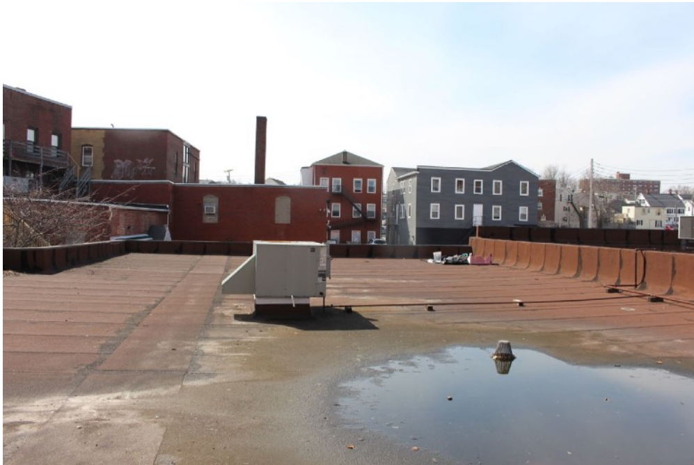
23 | Circa 1929 Addition - roof
