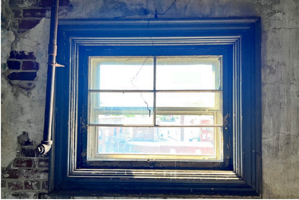
73 | Example of historic six-pane window at uppermost level of rear elevation (lower vertical muntin missing)
