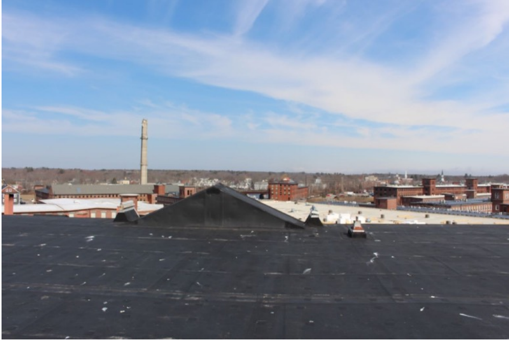
21 | Main Block - roof
