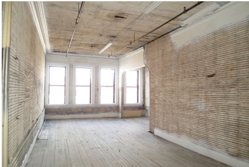
46 | Second Floor - view toward front (north) at center of building
