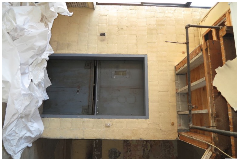
56 | Third Floor - added elevator in northeast corner
