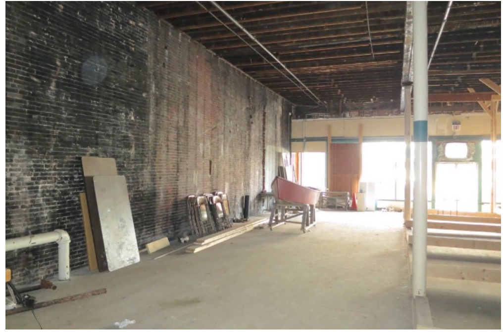
30 | First Floor - west wall of main block
