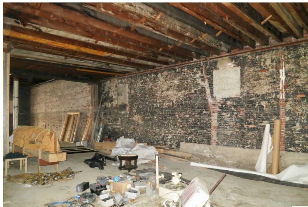
40 First Floor - view of west wall in ca. 1929 addition
