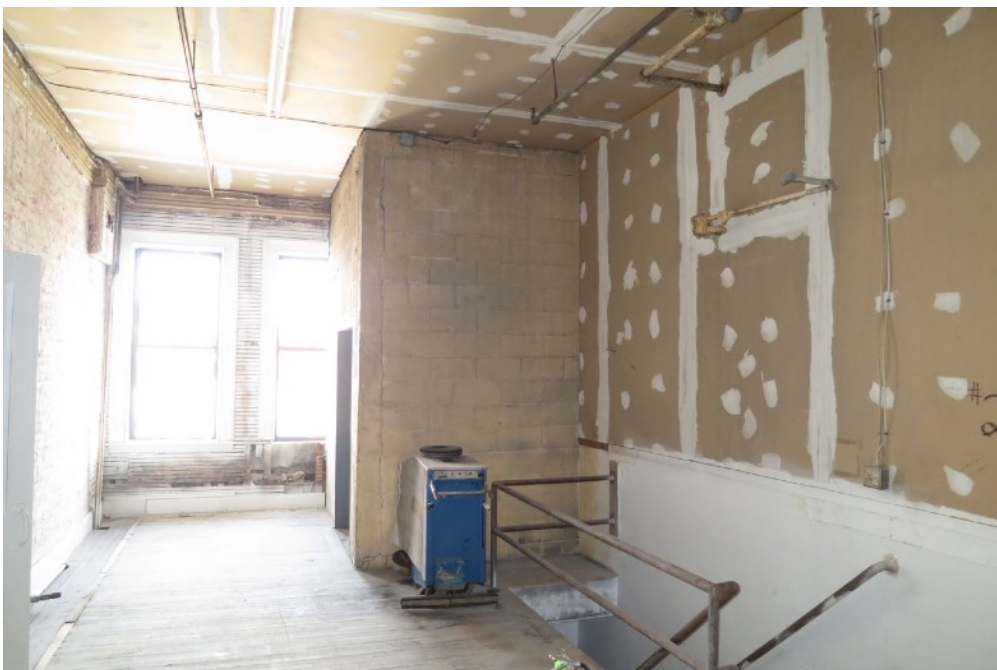
41 | Second Floor - view in northeast corner showing added stair and elevator enclosure
