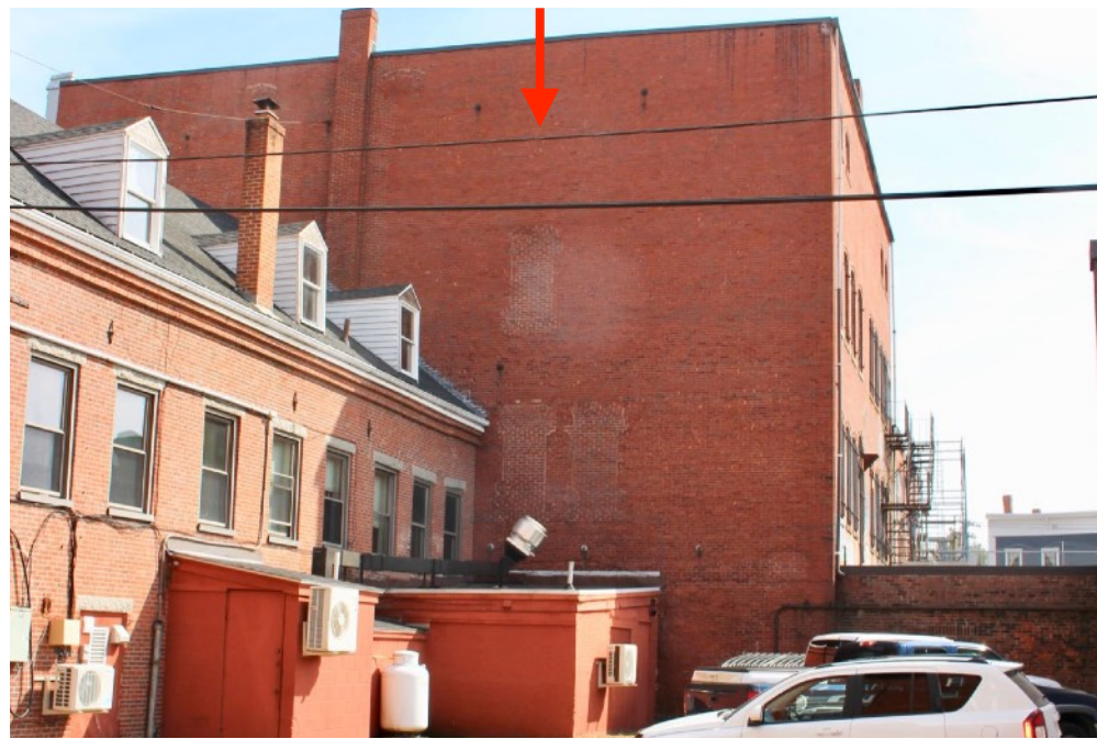
10 | West Elevation from south end
