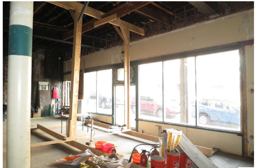
32 | First Floor - view along storefront in main block
