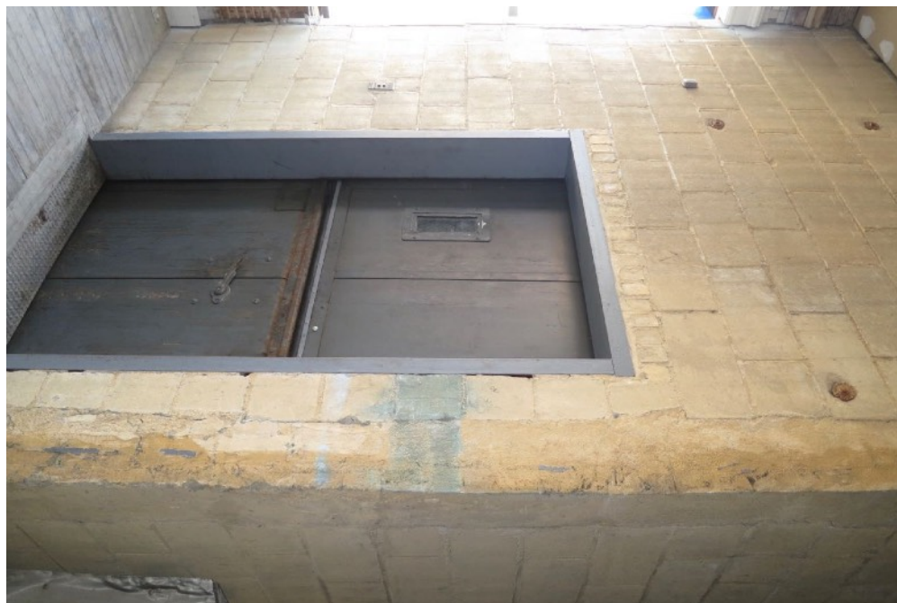
42 | Second Floor - added elevator in northeast corner
