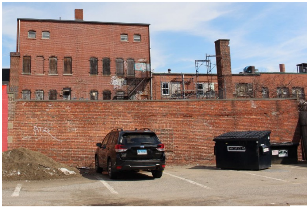
20 | Circa 1929 Addition - south elevation at east end
