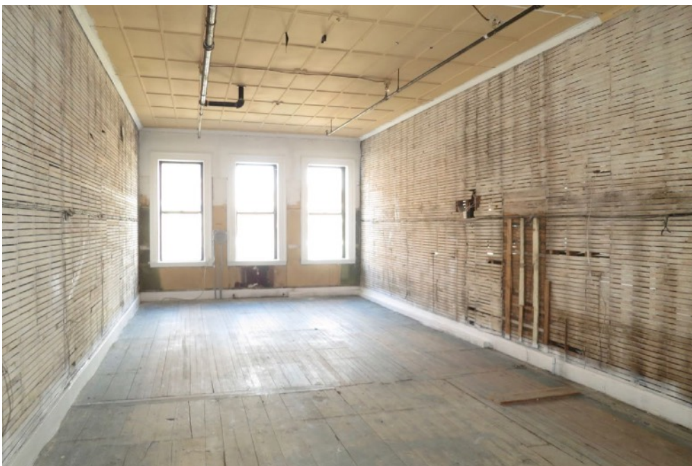
49 | Second Floor - view toward front (north) on west side of building
