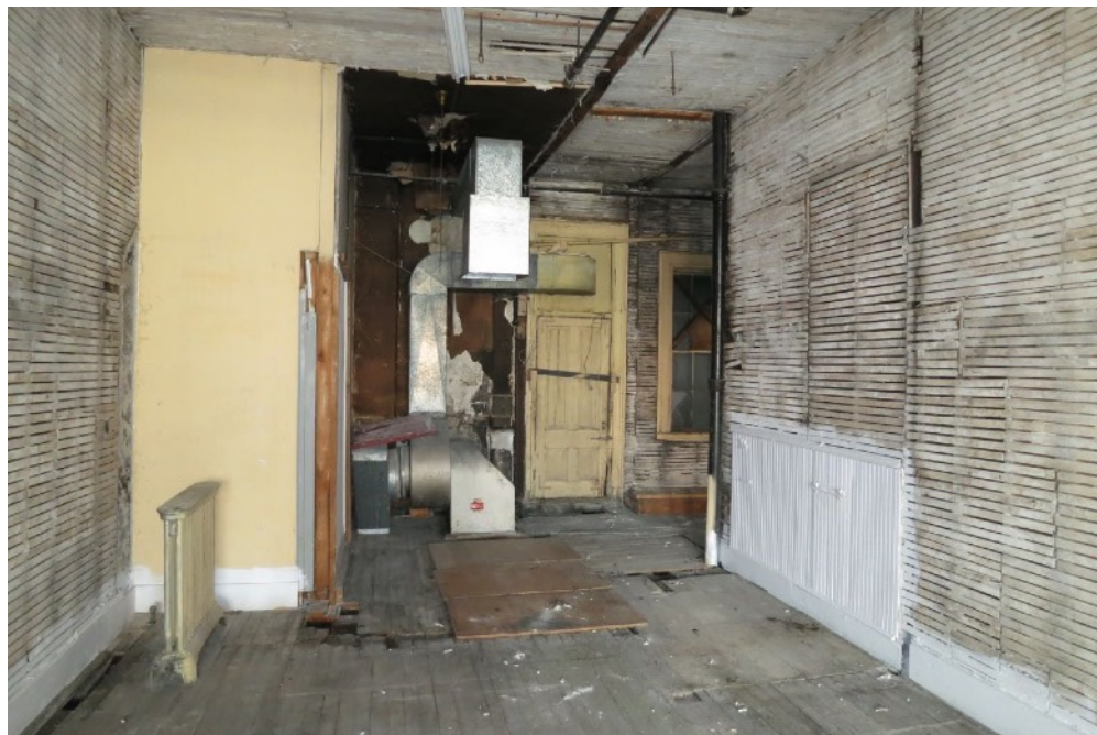
48 | Second Floor - view toward rear (south) at center of building
