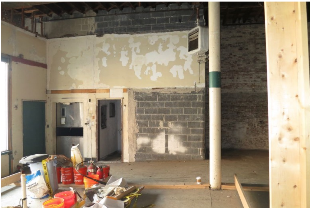
33 | First Floor - view toward added stair enclosure
