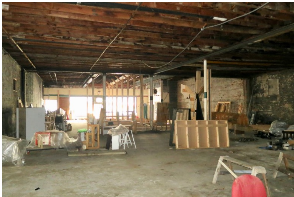
28 | First Floor - view toward storefronts of main block
