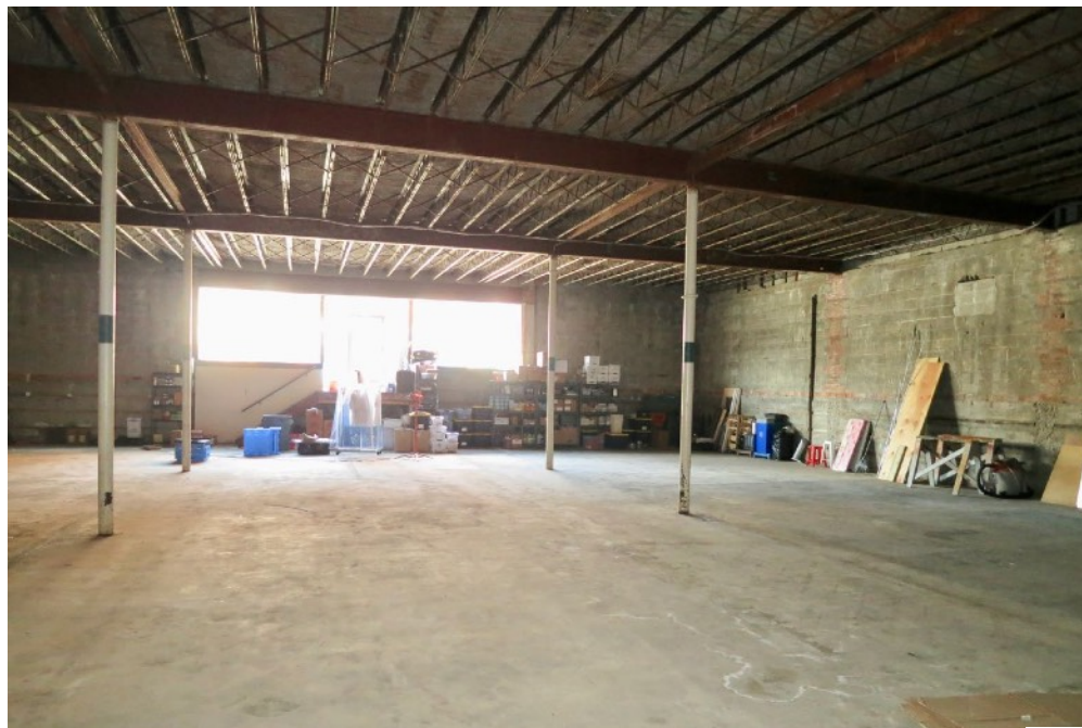
36 | First Floor - view west in ca. 1950 addition
