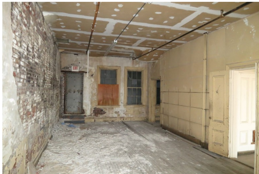
54 | Third Floor - view south along east side of building
