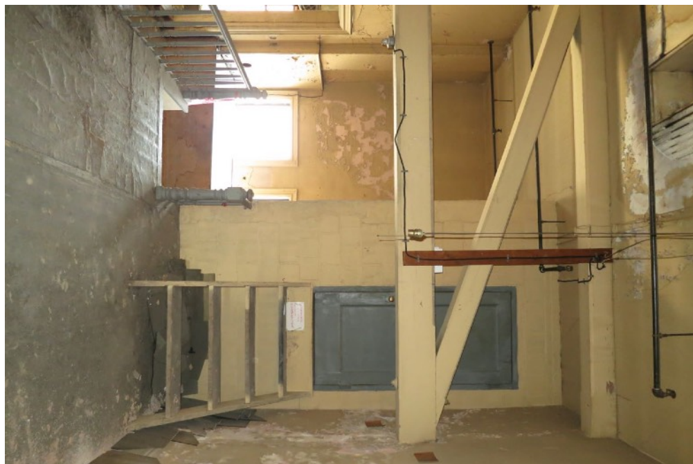
66 | Mezzanine - view north along east side of building
