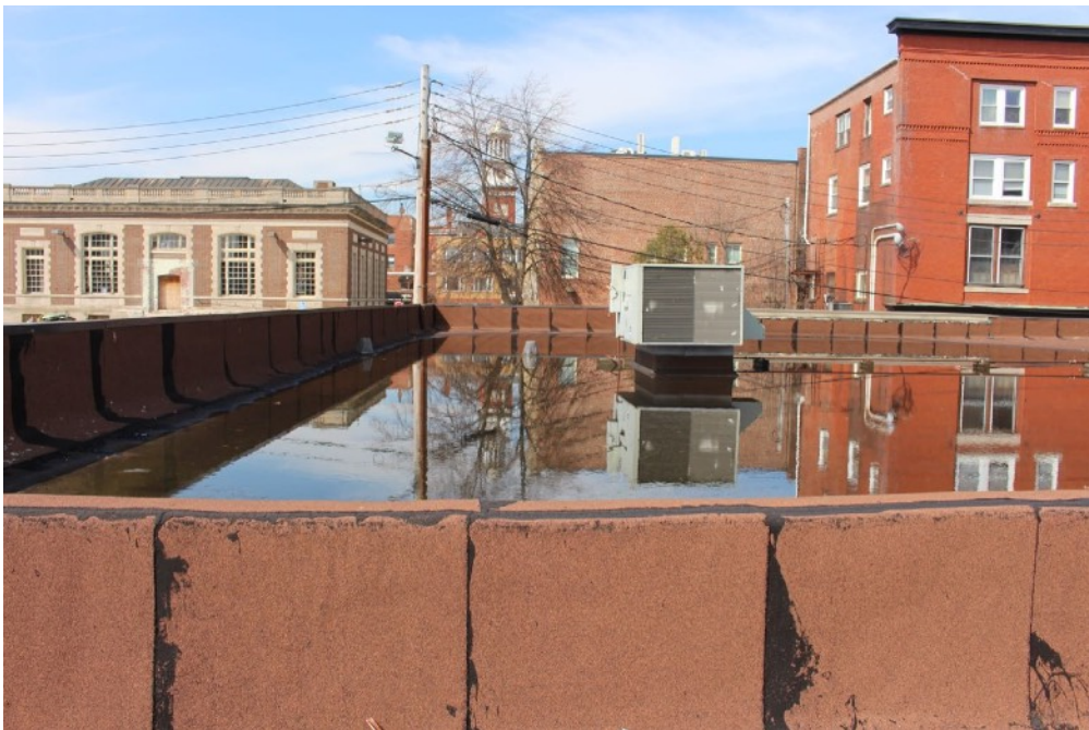
25 | Circa 1950 Addition - roof
