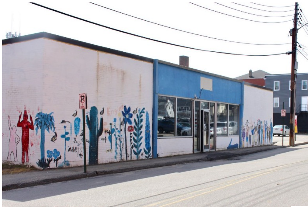
16 | Circa 1950 Addition - west elevation (facing Franklin Street)
