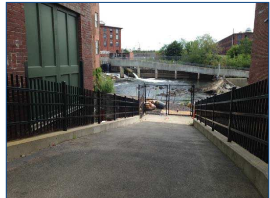
Photo 5: View of Ramp to Fall Plaza Area.
