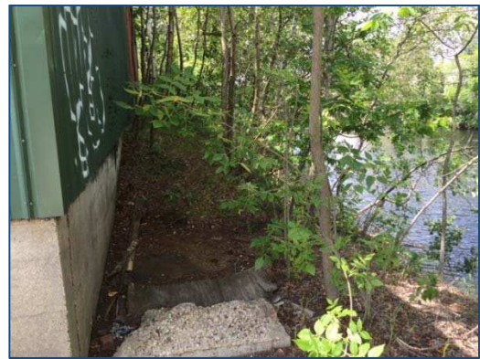
Photo 9: View behind existing Spring Island Buildings
