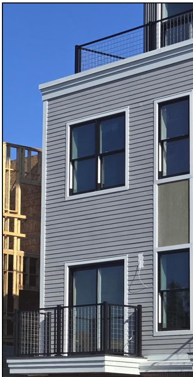
The Trex railing system as installed at 26 Upper Falls Road
