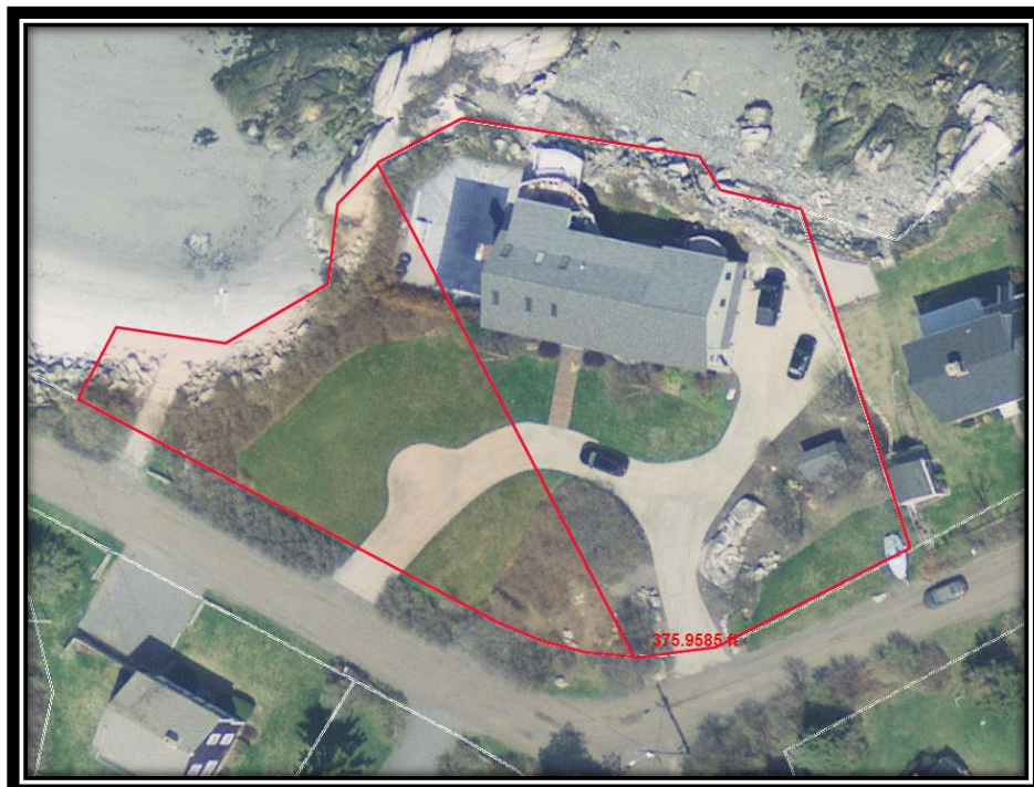
3 Sea Spray – Ramp Repair (Ramp shown far left from street to beach)
