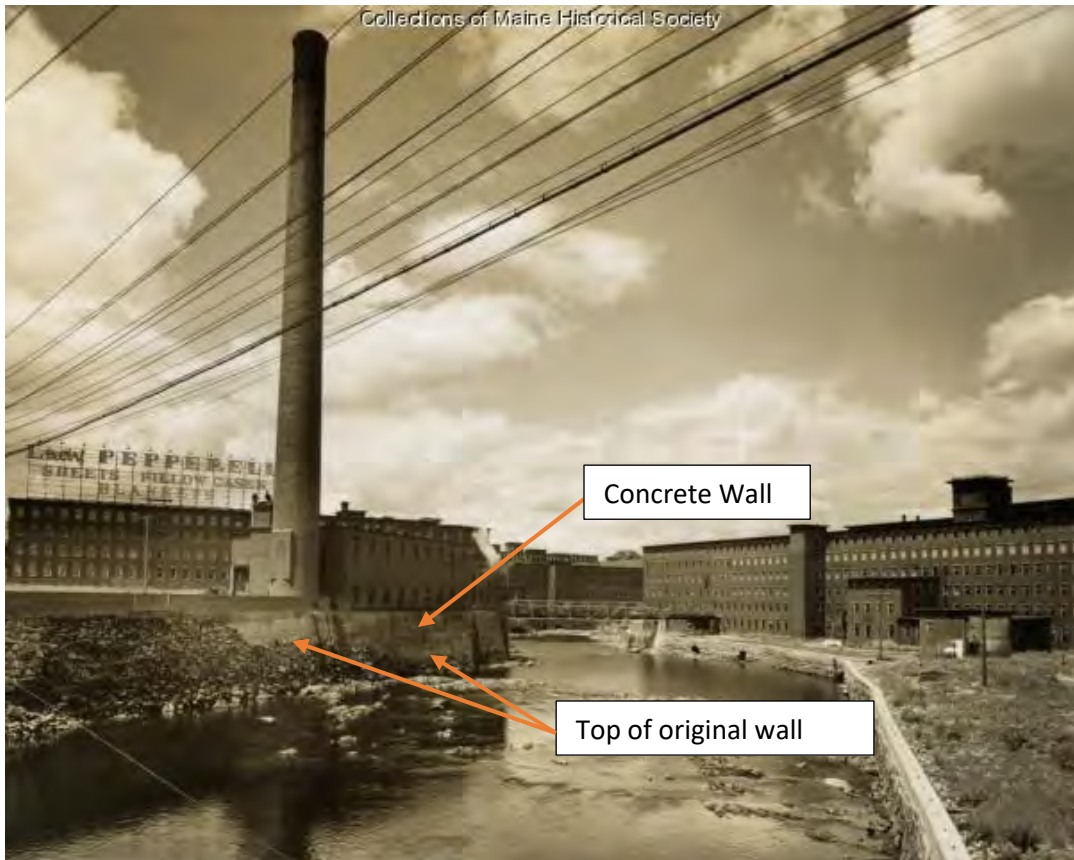
Photo 3 – Wall, Smokestack, and Boiler House Building Circa 1920 from mainmemory.net
