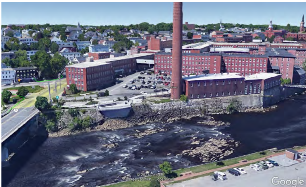
Photo 4 – Wall and Overhang Structure from Google Maps
