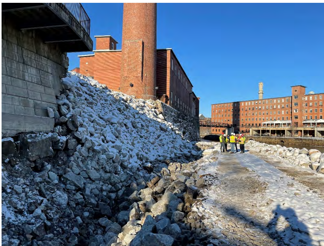
Photo 8 – Riprap Stabilized Slope and Access Road, December 9, 2021
