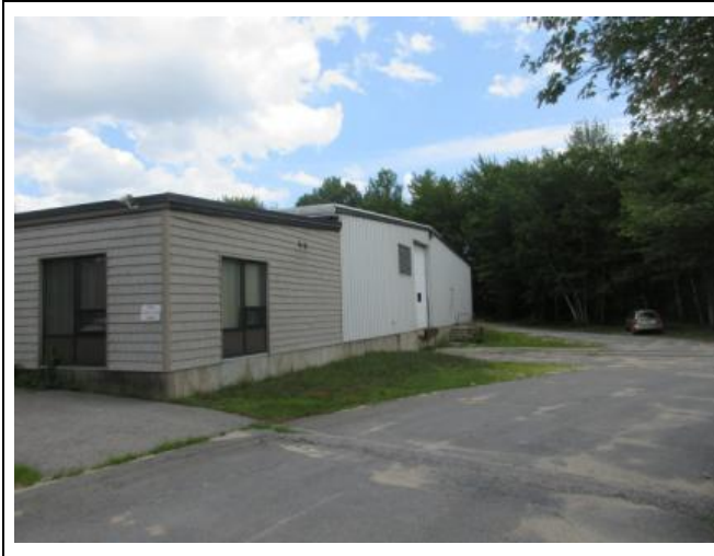
7) Southerly building elevation
