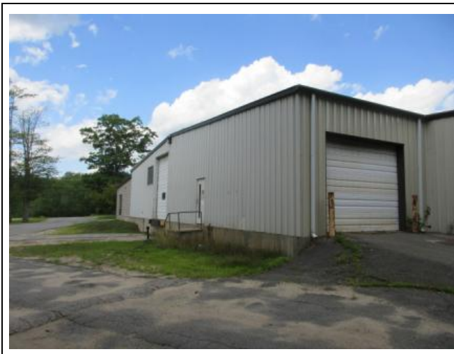
9) Southerly building elevation
