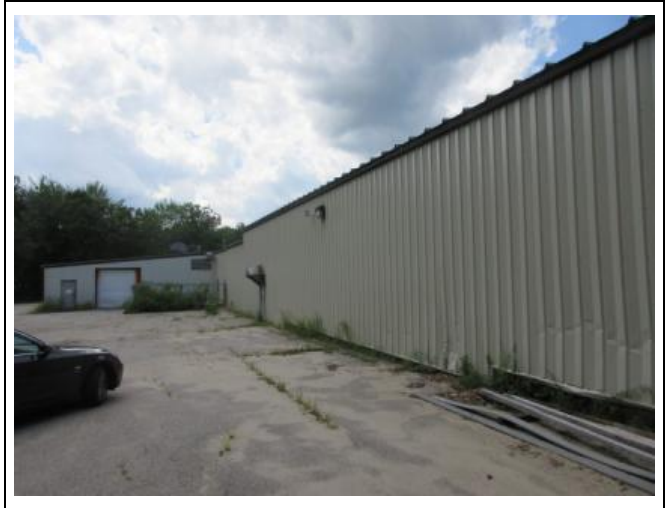
14) Easterly building elevation
