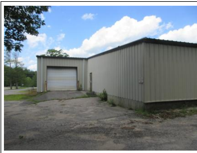
11) Southerly building elevation
