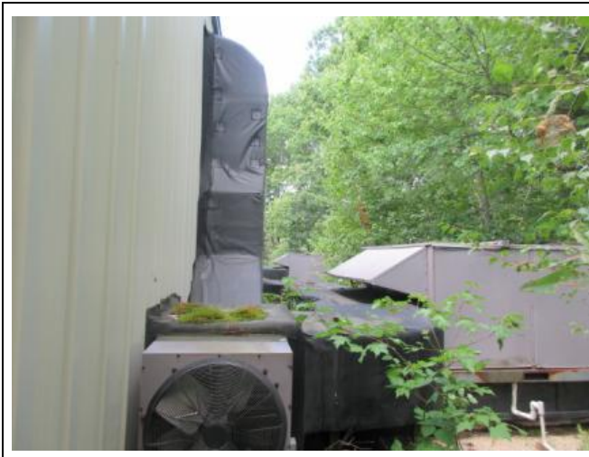
15) Northerly elevation showing exterior air handlers
