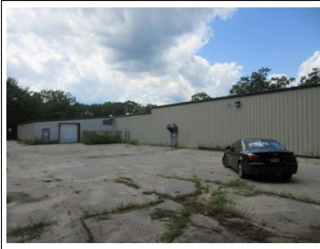
13) Easterly (rear) building elevations
