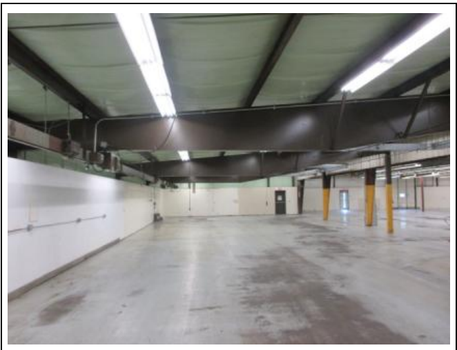
36) View of side production area
