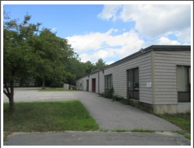
6) Westerly (front) elevation of office section
