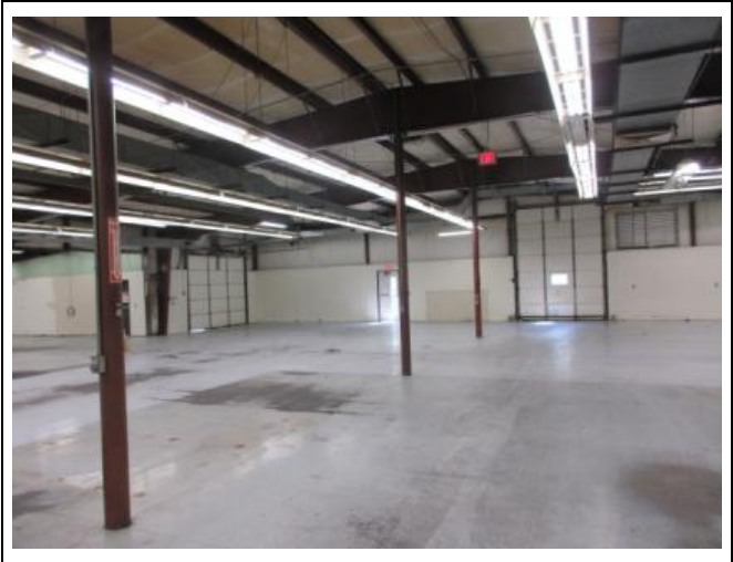
32) Original production floor looking toward loading door
