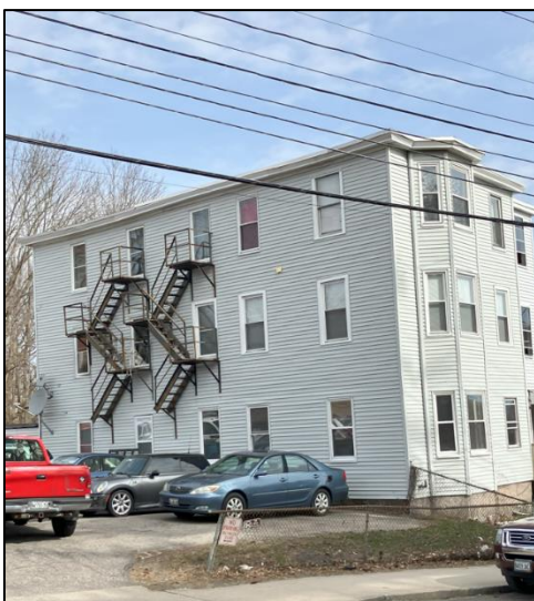
Installation of satellite dish at rear.
