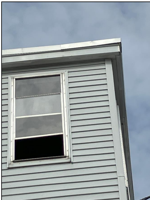
Fascia and soffit with flat coil stock.
