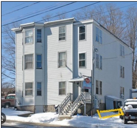
Approximate location of deck and condenser units, as seen from, street.
