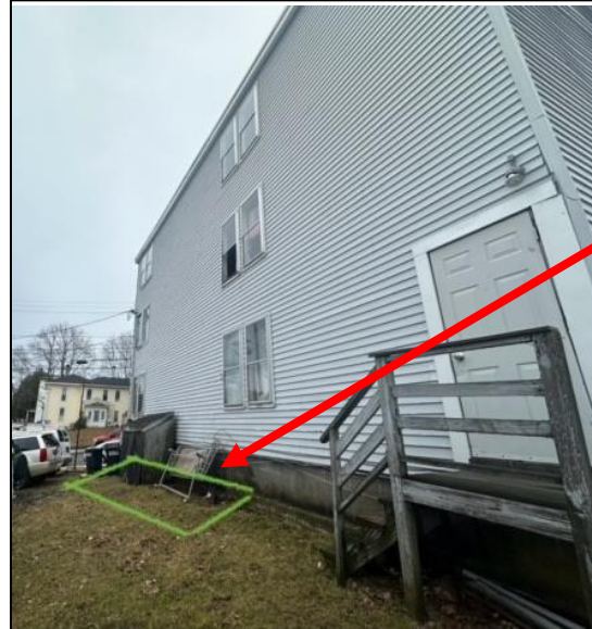
Approximate location of deck and condenser units
