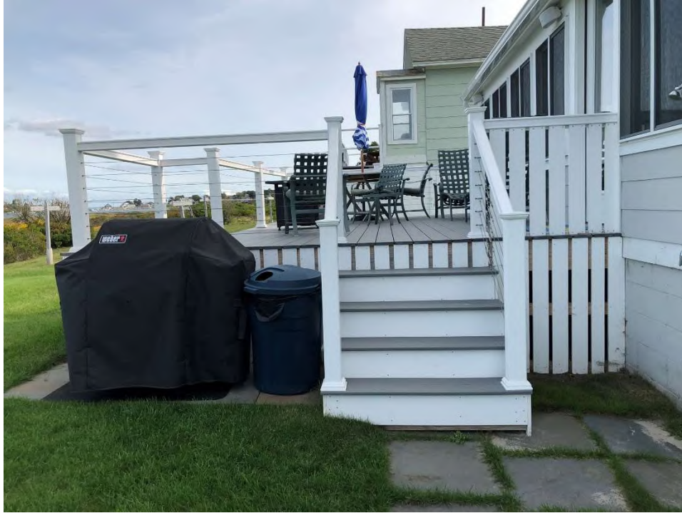
Photo 5: Back deck of building
