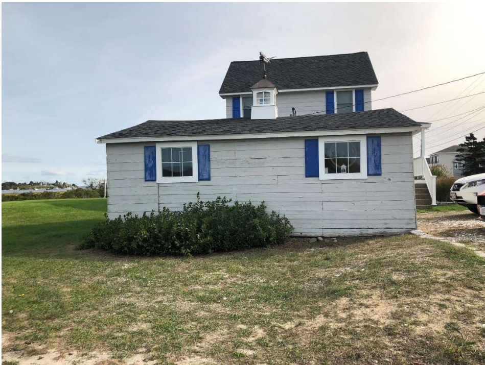
Photo 2: South Wall of Garage
