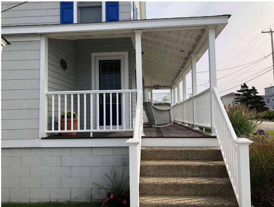
Photo 6: Covered front porch
