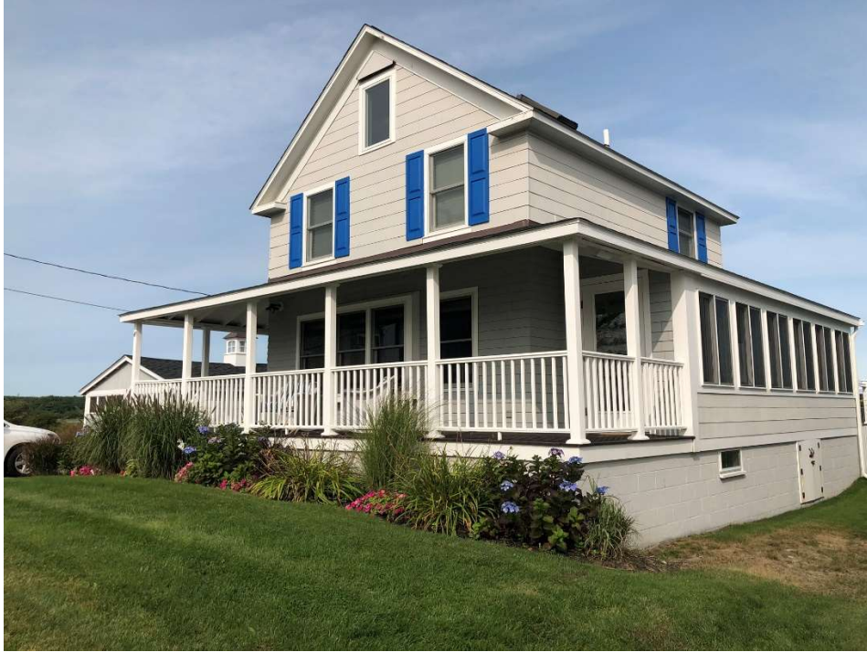
Photo 1: Southeast corner of property facing Building
