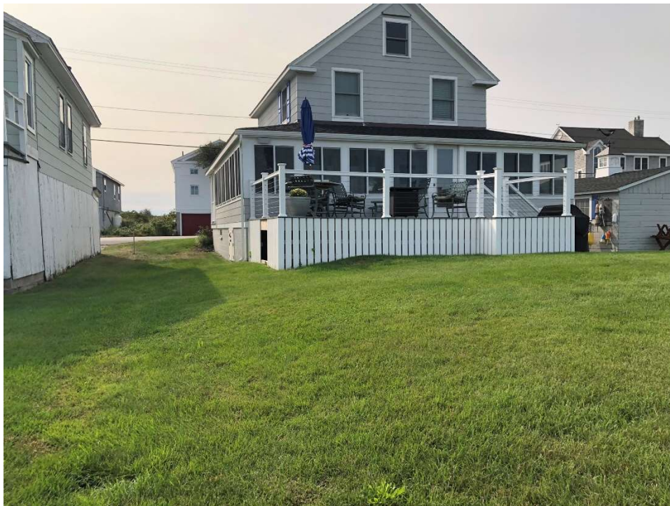
Photo 4: North corner of property showing building and property line
