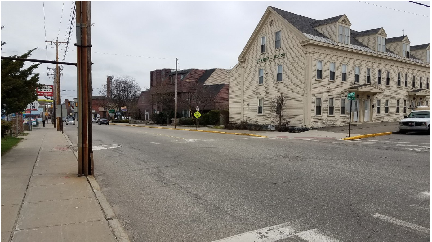
Figure 3 – View of East Side of Alfred Street
