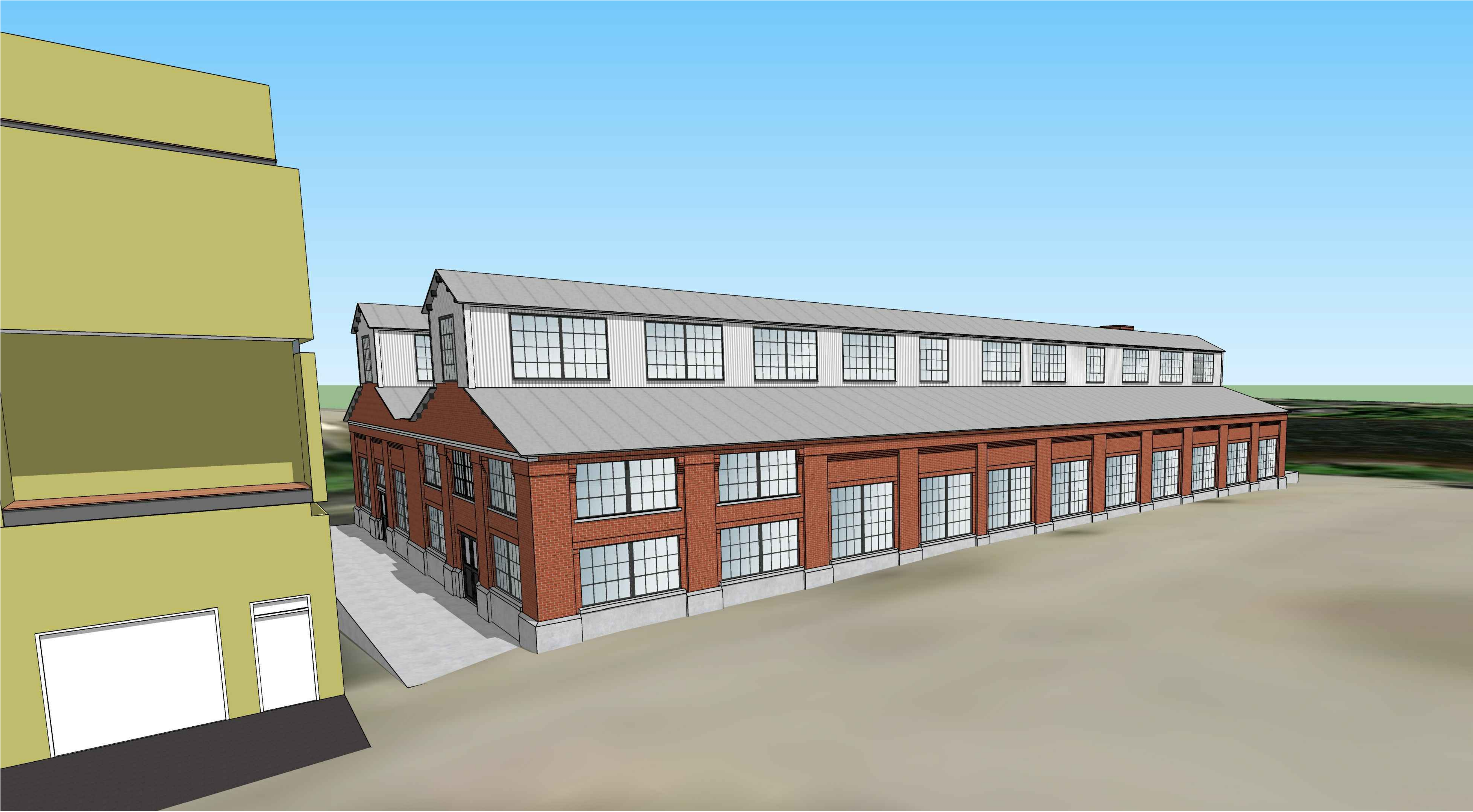
1 VIEW LOOKING EAST FROM GOOCH STREET
