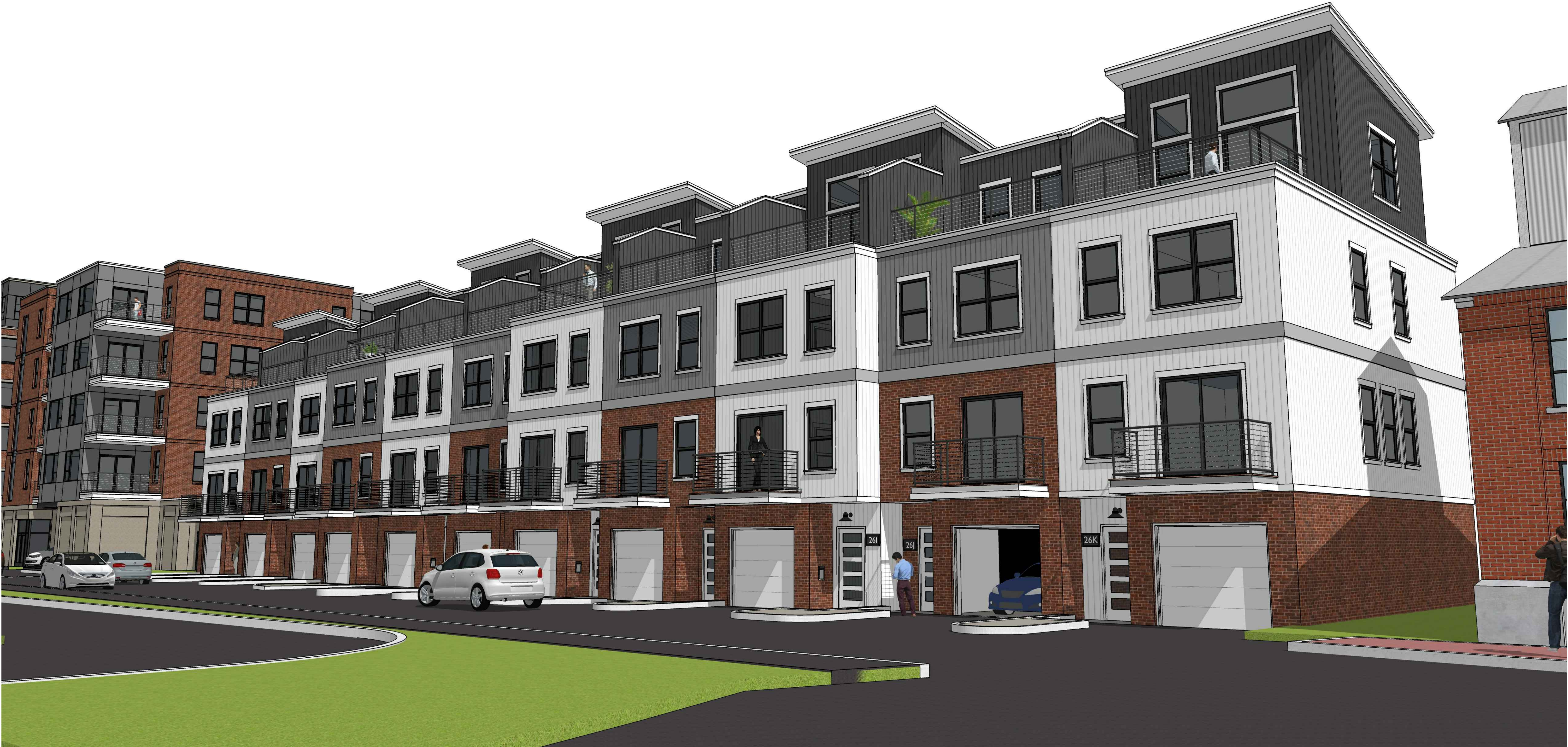
1 BUILDING C - VIEW LOOKING NORTH WEST N.T.S.
