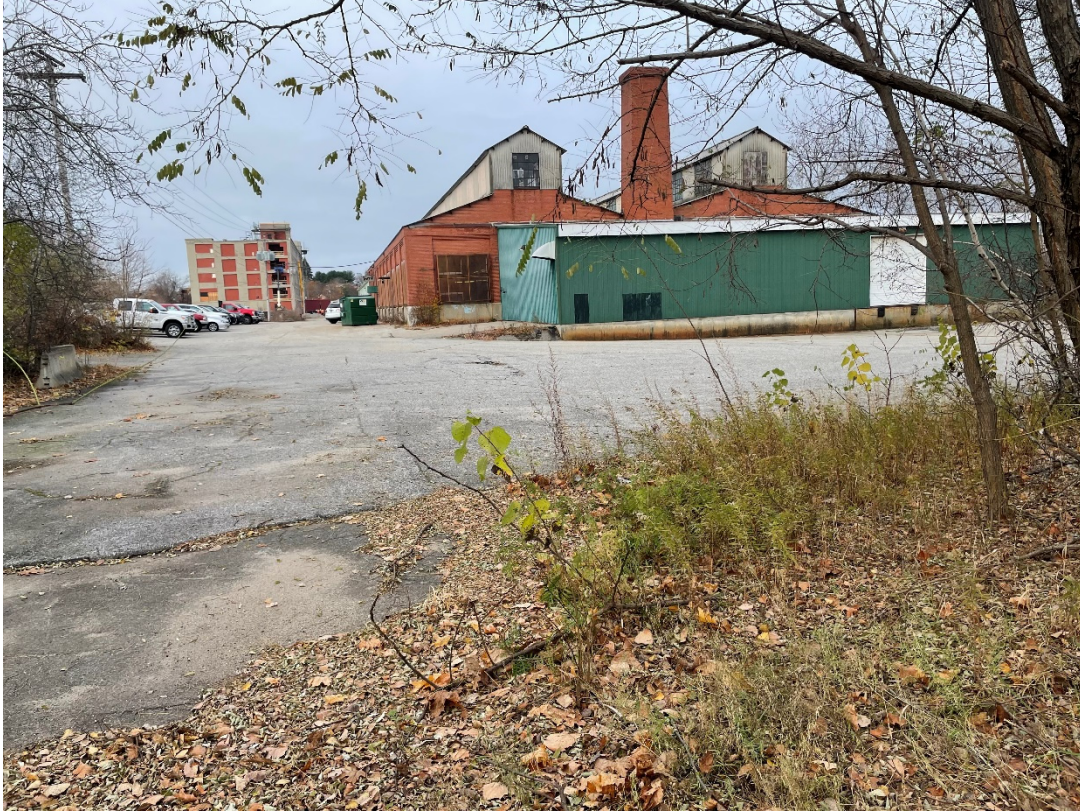
Figure 9: View of 30 Gooch Street facing west.
