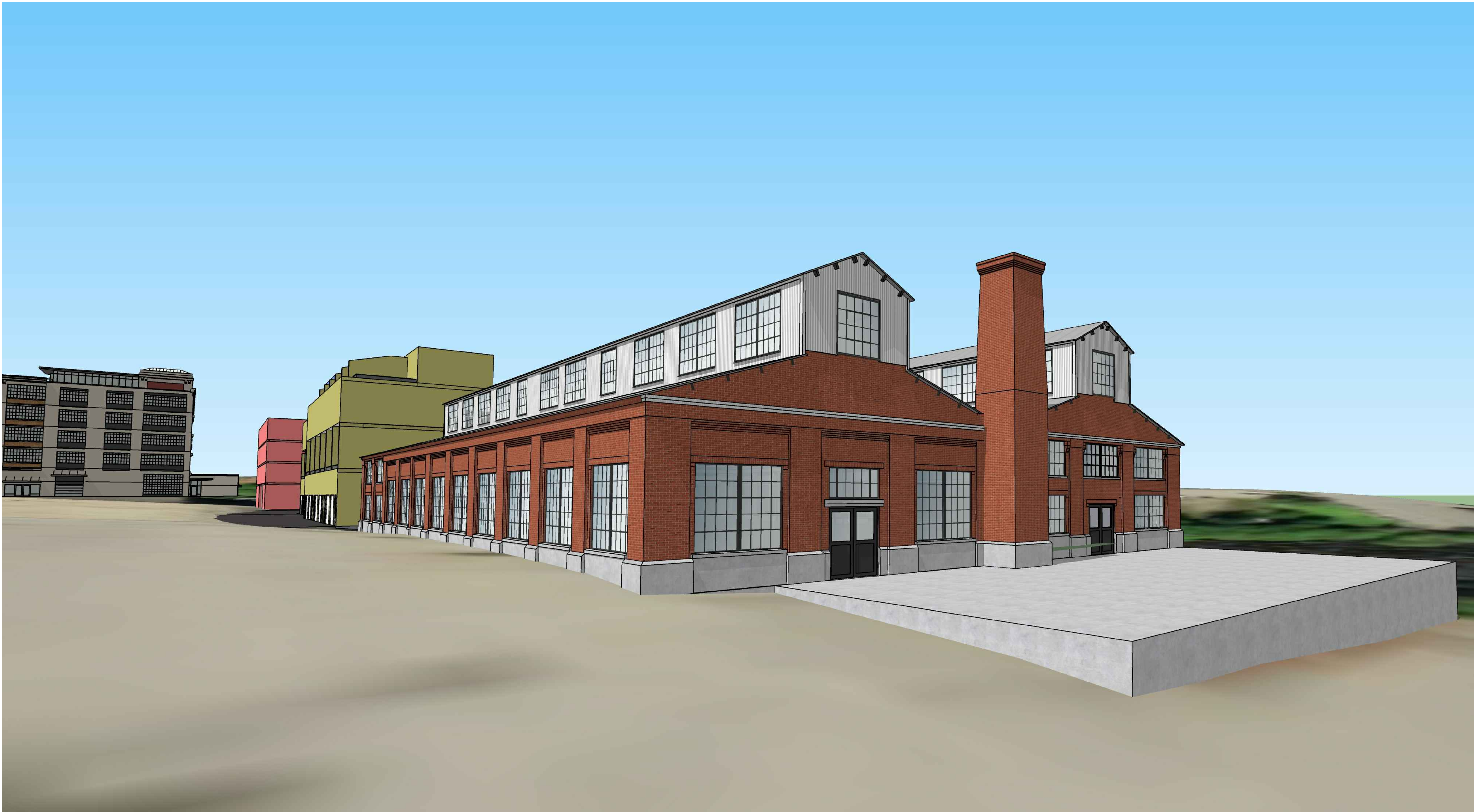
1 VIEW LOOKING NORTH-WEST FROM GOOCH STREET
