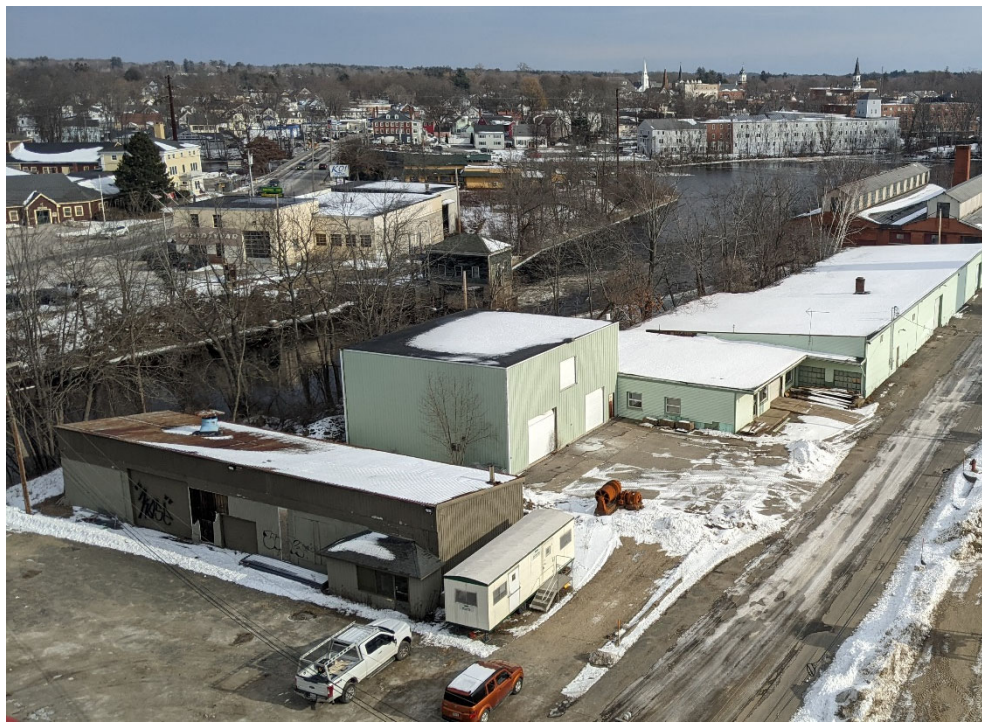
Figure 1: View of part of 10 and 20 Gooch Street taken from the roof of 1 Gooch Street building.
