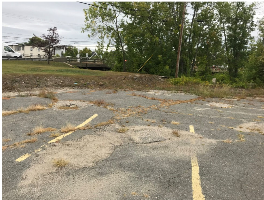
Figure 4: Standing on the existing parking lot on 10 Gooch site facing northwest toward the Saco River.
