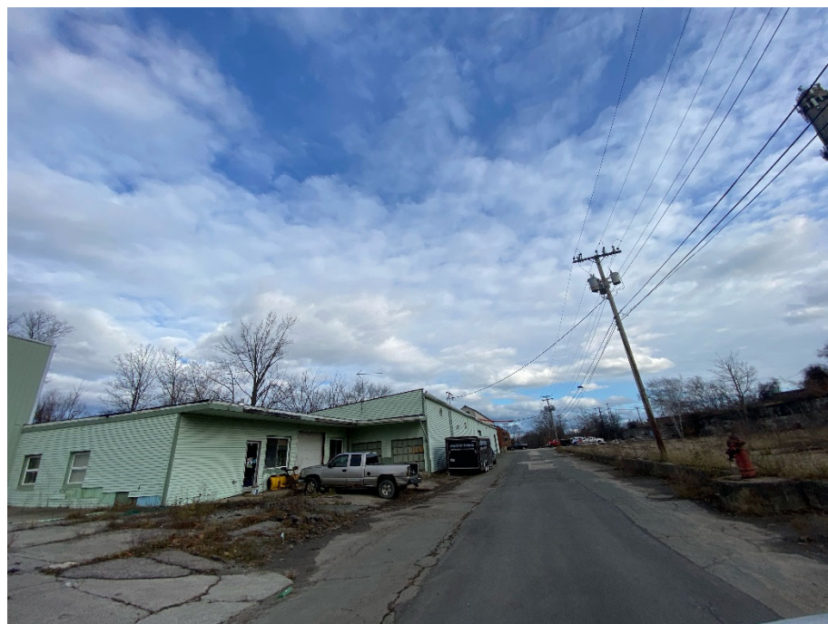
Figure 8: View of 20 Gooch Street facing east.
