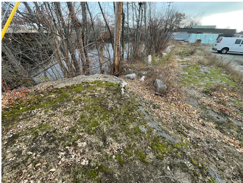
Figure 6. Standing northeast of the existing 10 Gooch Street parking lot facing east.
