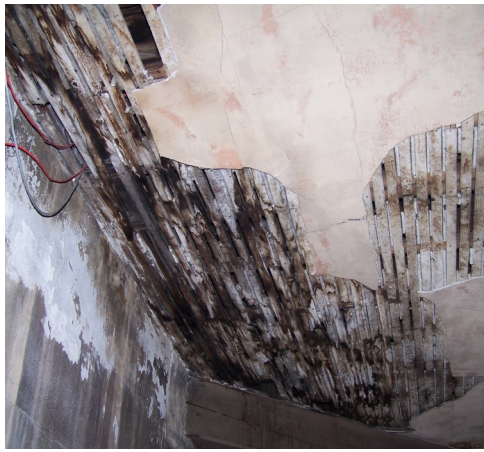
Belfry Deck Before Restoration
