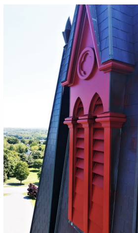
Wood Louver After Repair
