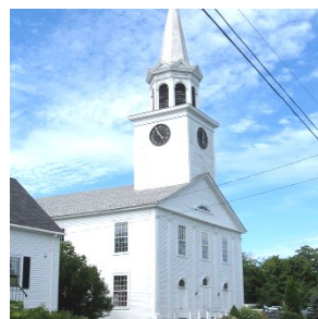
EASTPORT CONGREGATIONAL CHURCH Eastport, Maine
