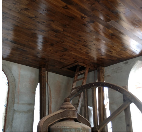
Belfry Roof After Restoration
