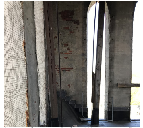
Lancet Opening Before Weatherproofing
