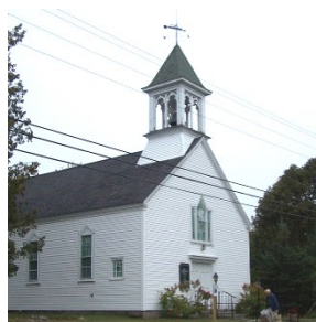
SUNSET CONGREGATIONAL CHURCH Stonington, Maine
