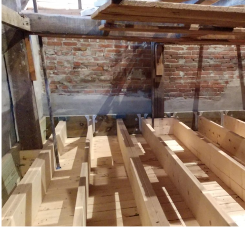
Belfry Deck After Restoration
