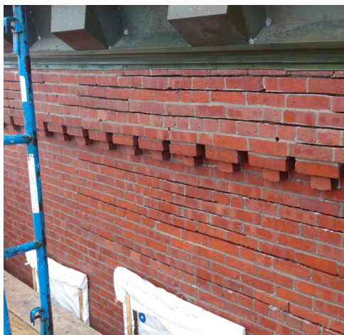
Masonry After Repair
